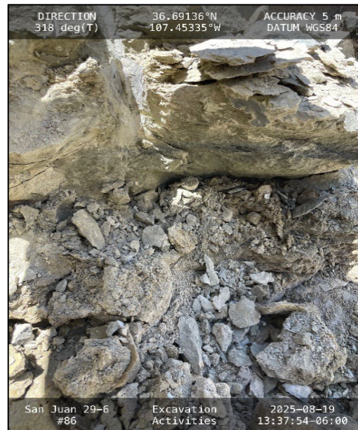
Photograph: 4 Date: 8/19/2025 Description: Stained layer @ ~25' bgs. View: Northwest.
