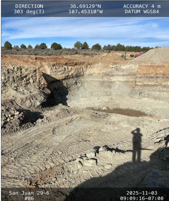
Photograph: 1 Date: 11/3/2025 Description: Deep side of excavation View: Northwest
