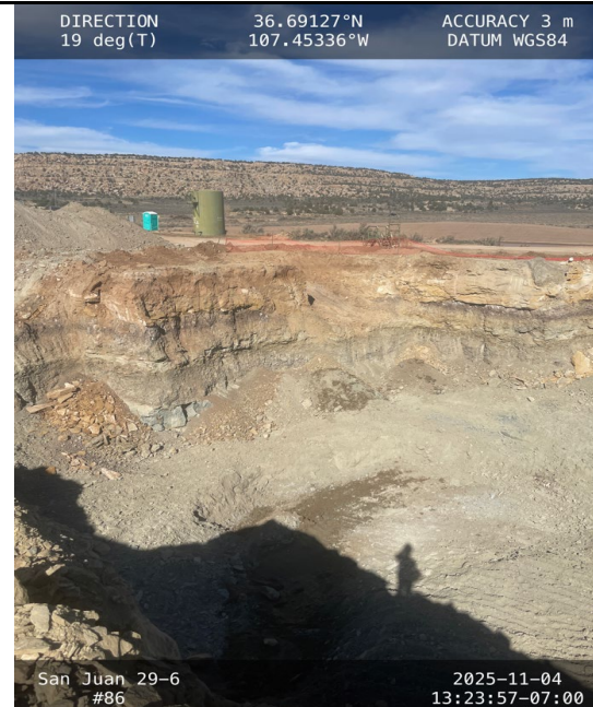
Photograph: 3 Date: 11/4/2025 Description: Final Excavation Extent View: Northeast
