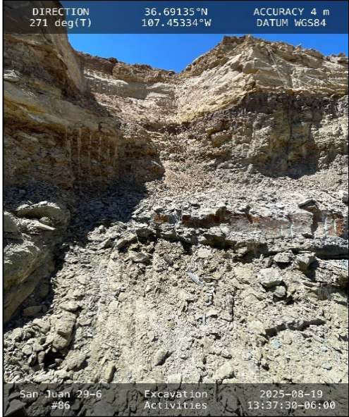
Photograph: 1 Date: 8/19/2025 Description: NW Sidewall View: SS21 directly below the lower bench.
