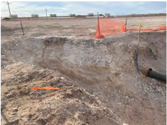
Photograph 4 Date: 04/01/2021 Description: East Excavation View: Northwest
