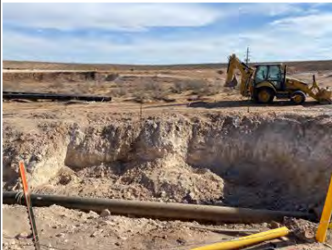
Photograph 3 Date: 03/15/2021 Description: East Excavation View: South
