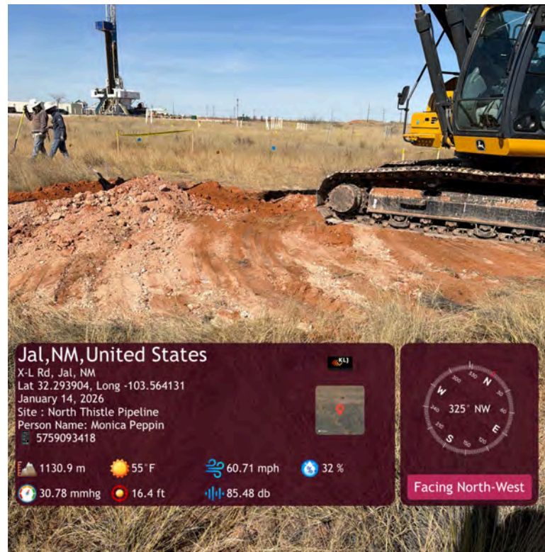
TP07 being backfilled.
