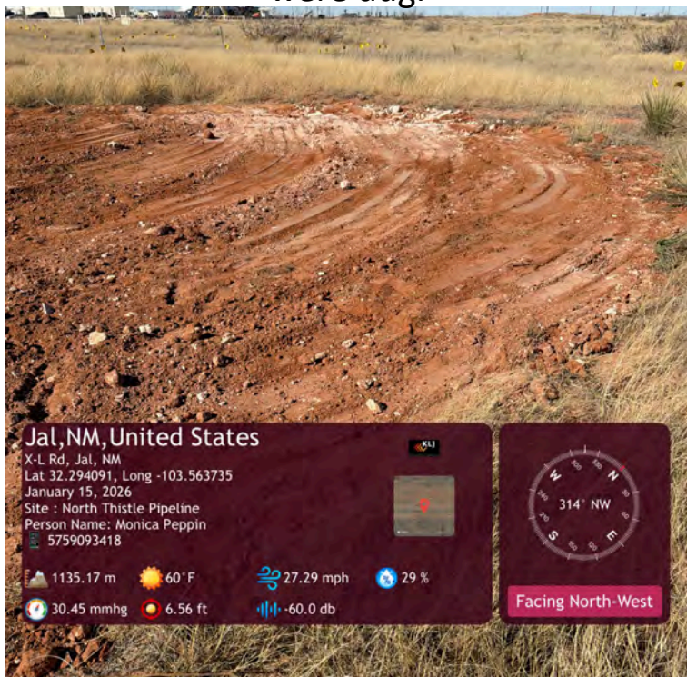
backfill area of TP09.
