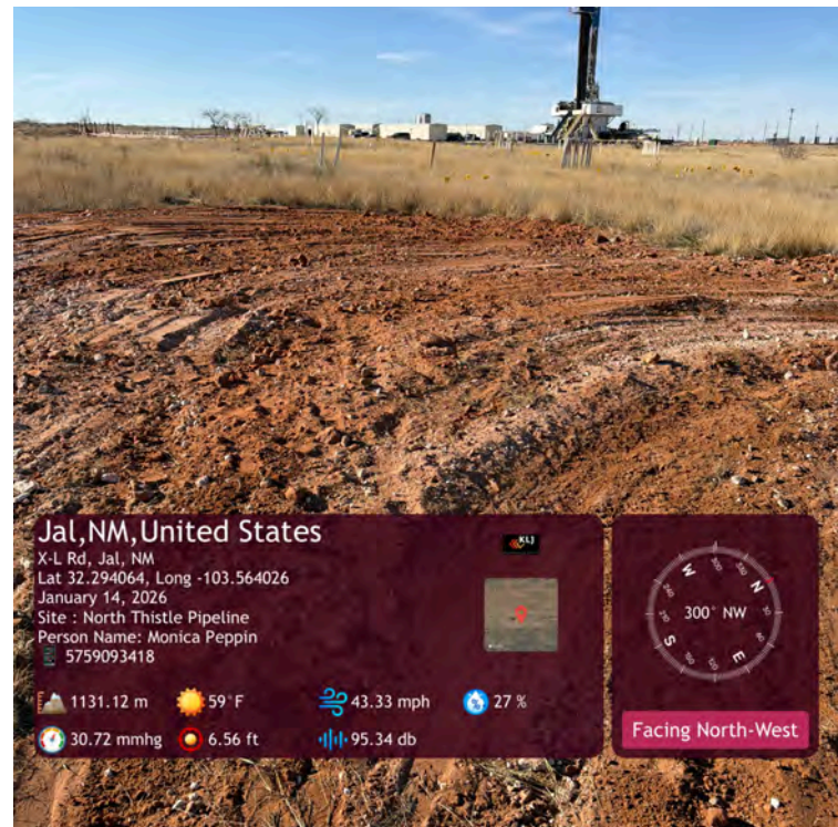
Backfill area of TP 07 on west end.
