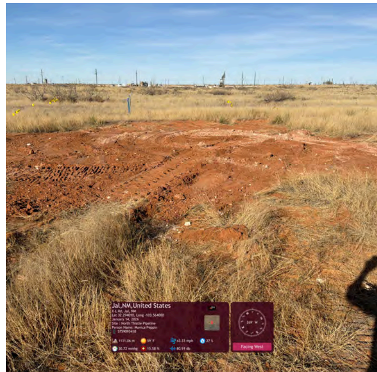
Backfill area from TP04.
