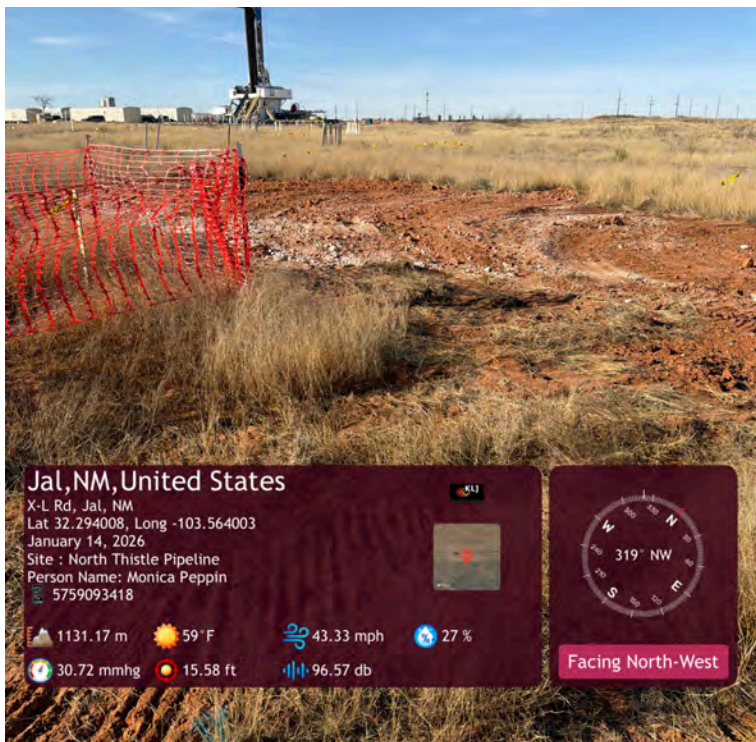
TP05/TP06 area backfilled.
