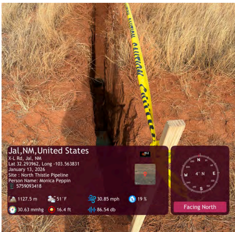
Flowlines hydrovacted for visibility of underground utilities.
