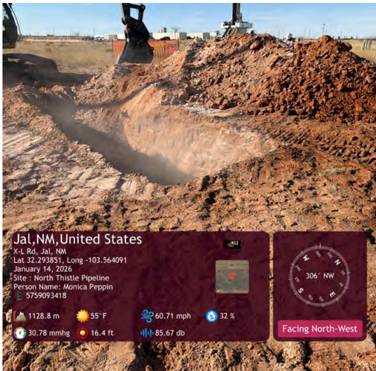
TP09 being dug for sample collection.
