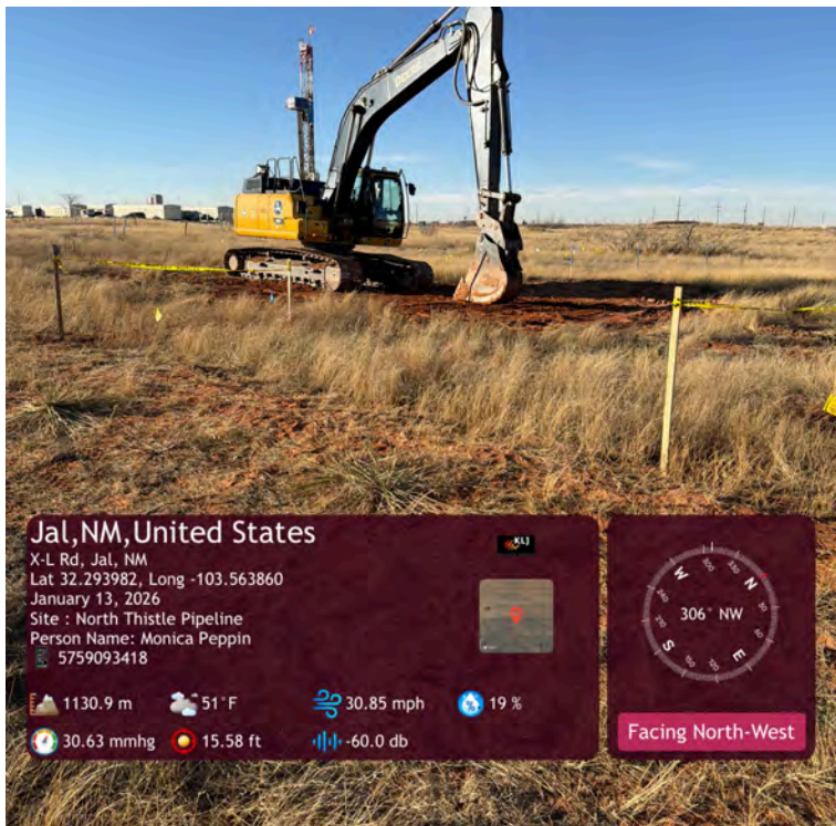
Backfill of test pit location TP04.
