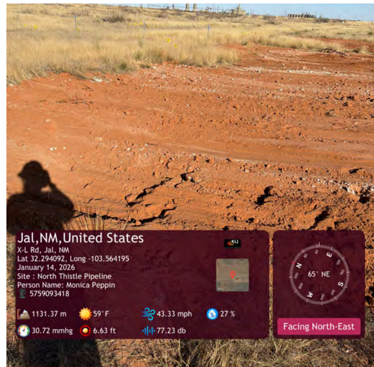
Backfilled area from test pits on north side.
