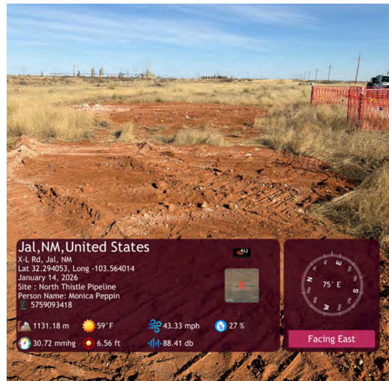
Backfill area from test pit locations on north side.
