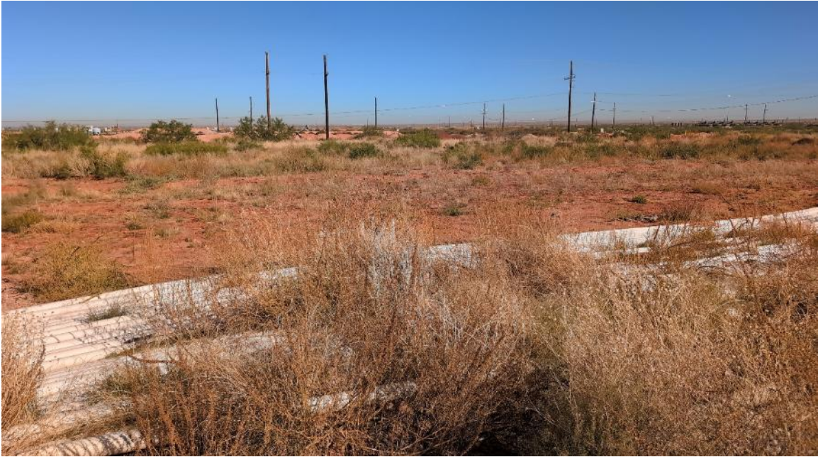
Photograph 15: PP-03, facing north
