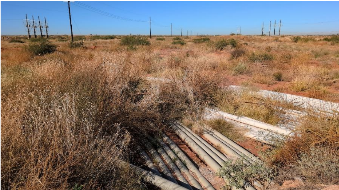
Photograph 16: PP-03, facing northwest
