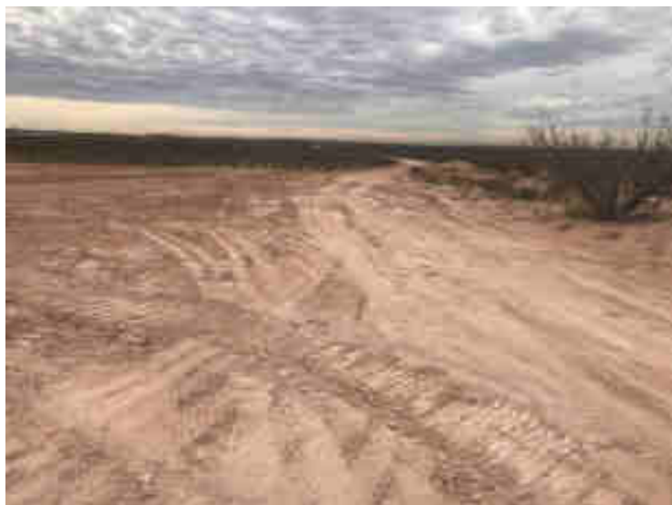
Photograph 5: View south of western side of pad after scraping.
