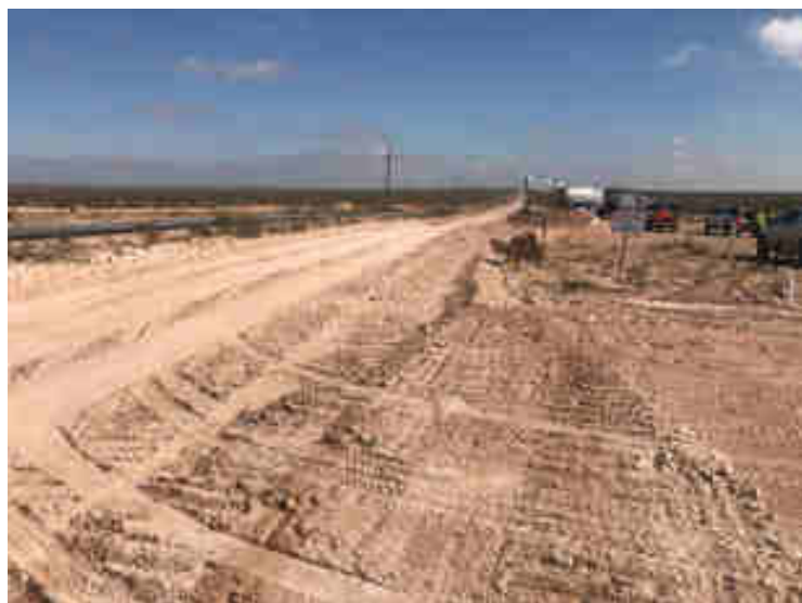
Photograph 7: View east of lease road after scraping road.
