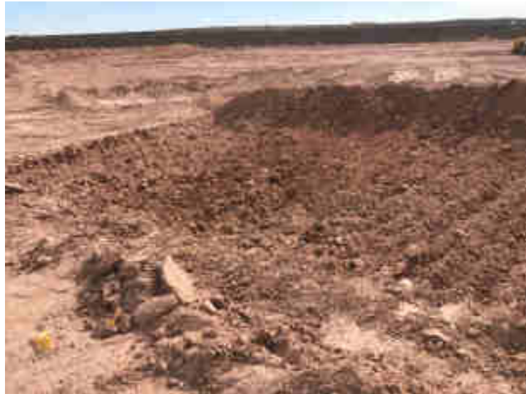
Photograph 3: View of the excavation on pad facing south.
