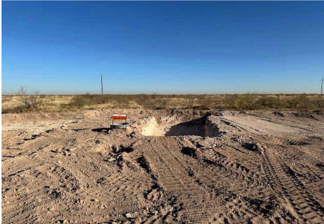
Photo 5 View of looking N at the 6-foot deep excavation area.
