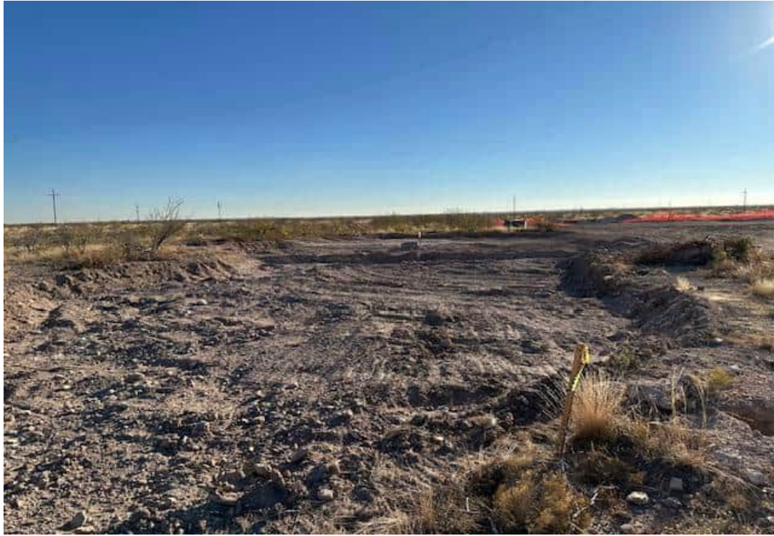
Photo 1 View from W side of excavation looking E at release area.
