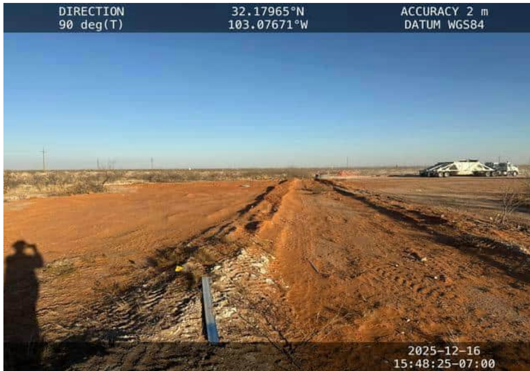
Photo 2 View from W side of excavation looking E backfilled.
