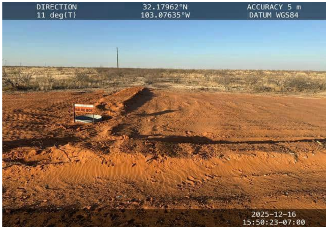
Photo 6 View of looking N at the 6-foot deep excavation area backfilled.
