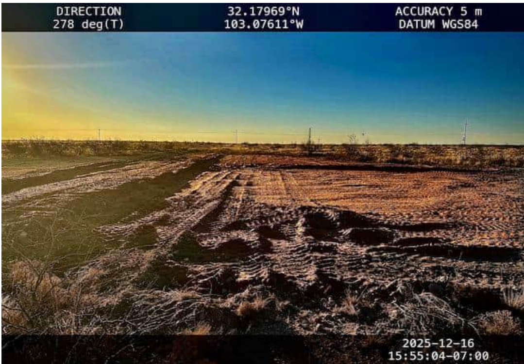
Photo 4 View from E side of excavation looking W backfilled.
