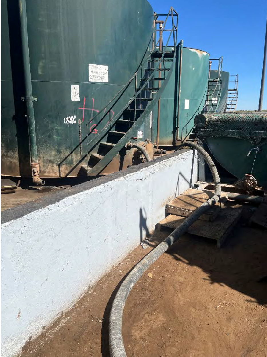
Image 4. Eastern Perimeter Wall Showing no Evidence of Permeability Exposure
