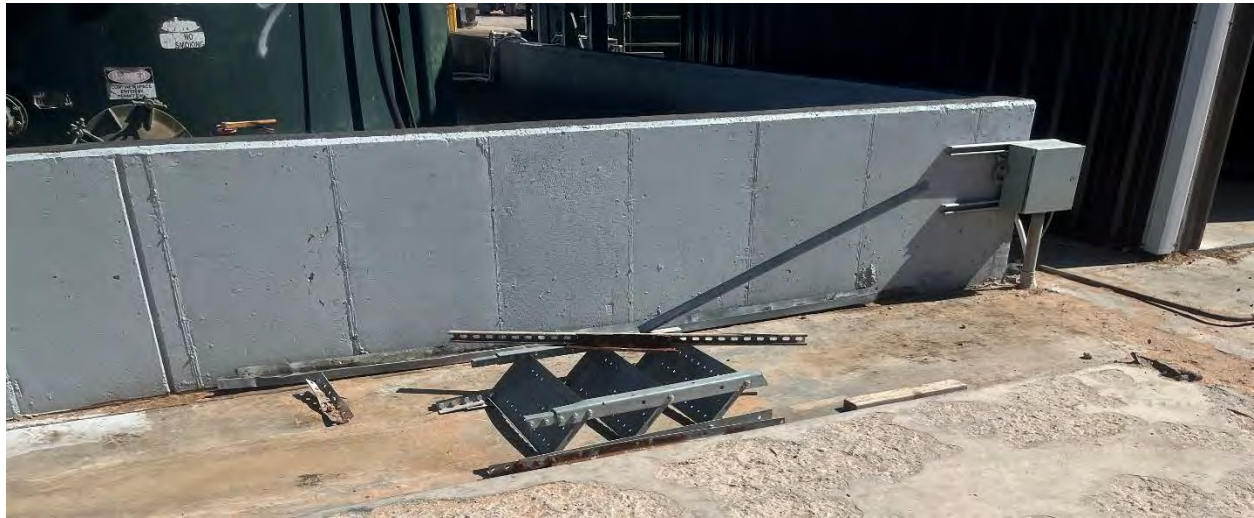
Image 7. Southern Exterior Perimeter wall of Secondary Containment
