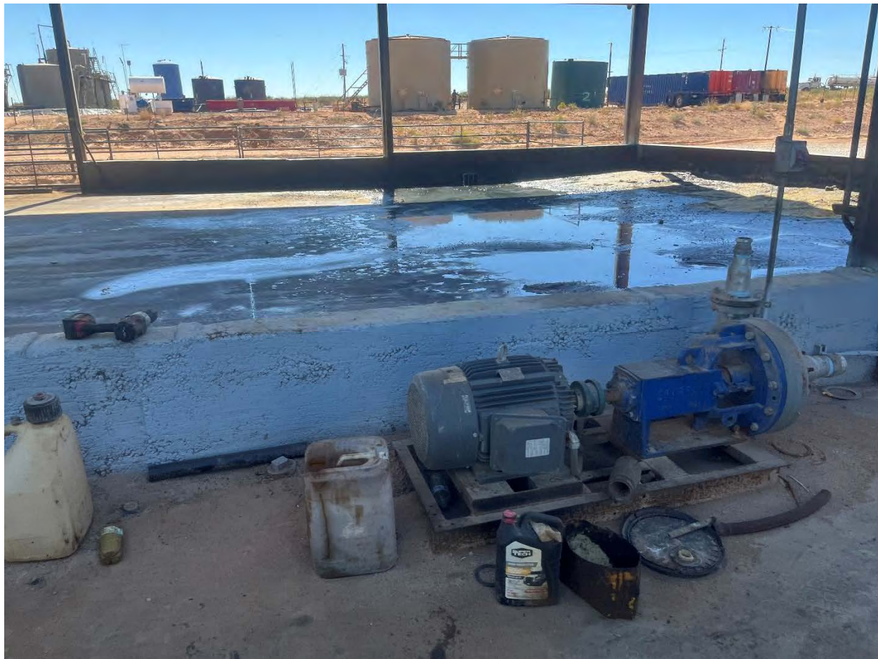
Image 12. The other Half of the Outer Western Perimeter of Washout Pad showing Honeycombing
