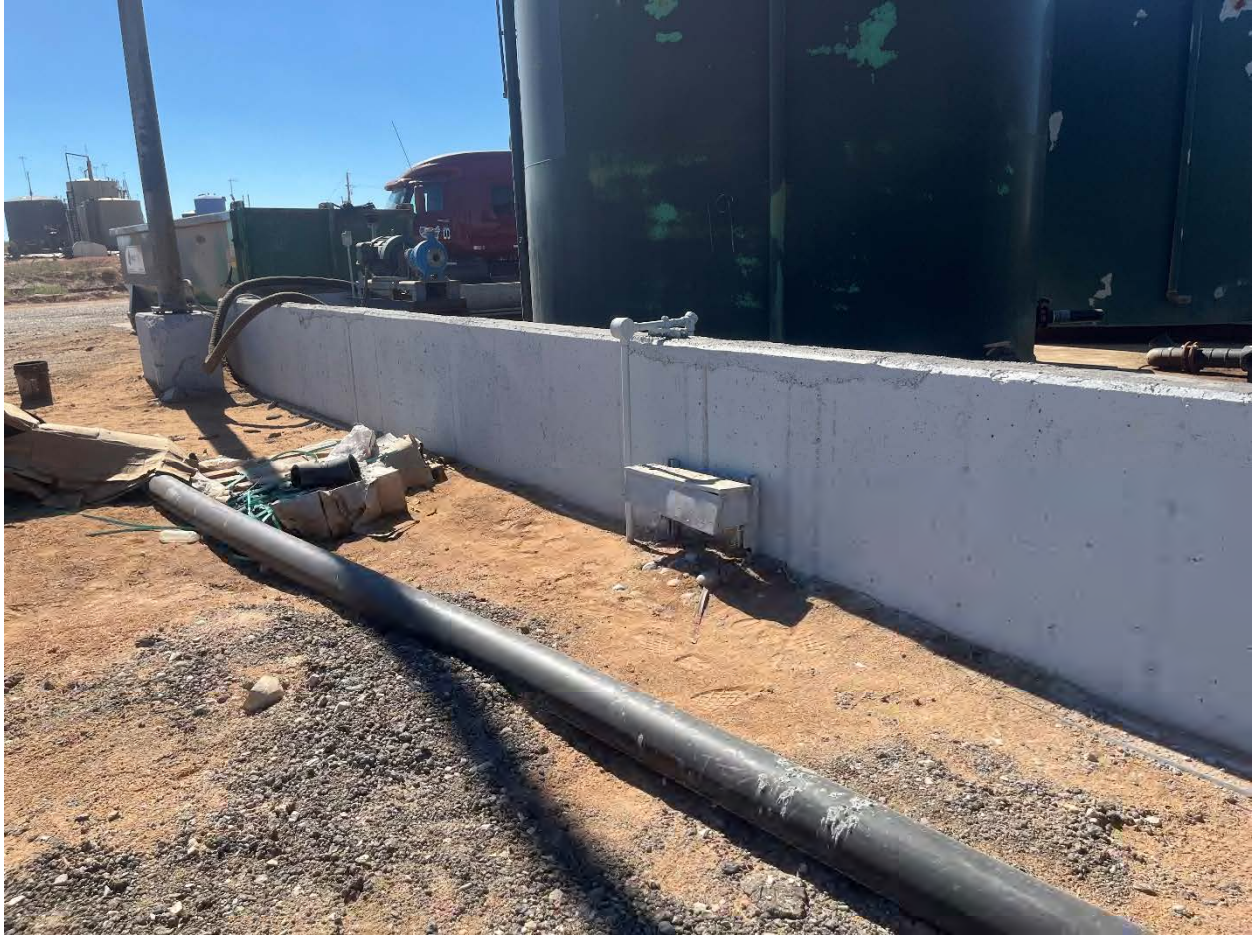
Image 2. Northern Perimeter Wall Showing no Evidence of Permeability Exposure
