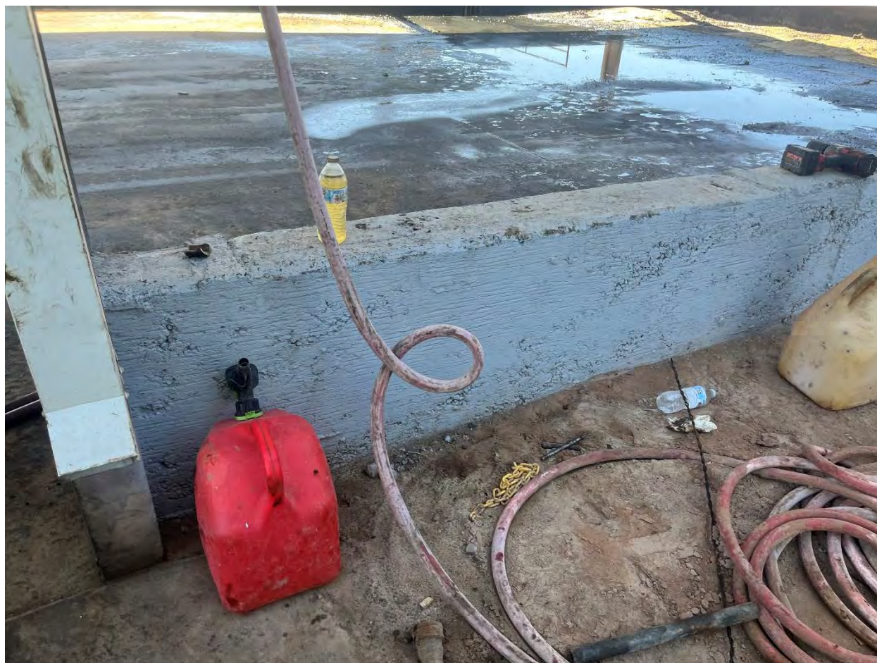
Image 13. The other Half of the Outer Western Perimeter of Washout Pad showing Honeycombing
