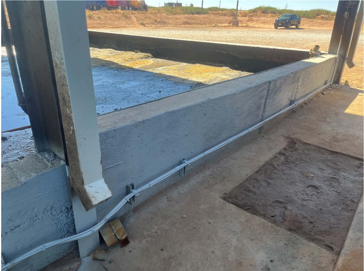
Image 11. Half of the Outer Western Perimeter of Washout Pad
