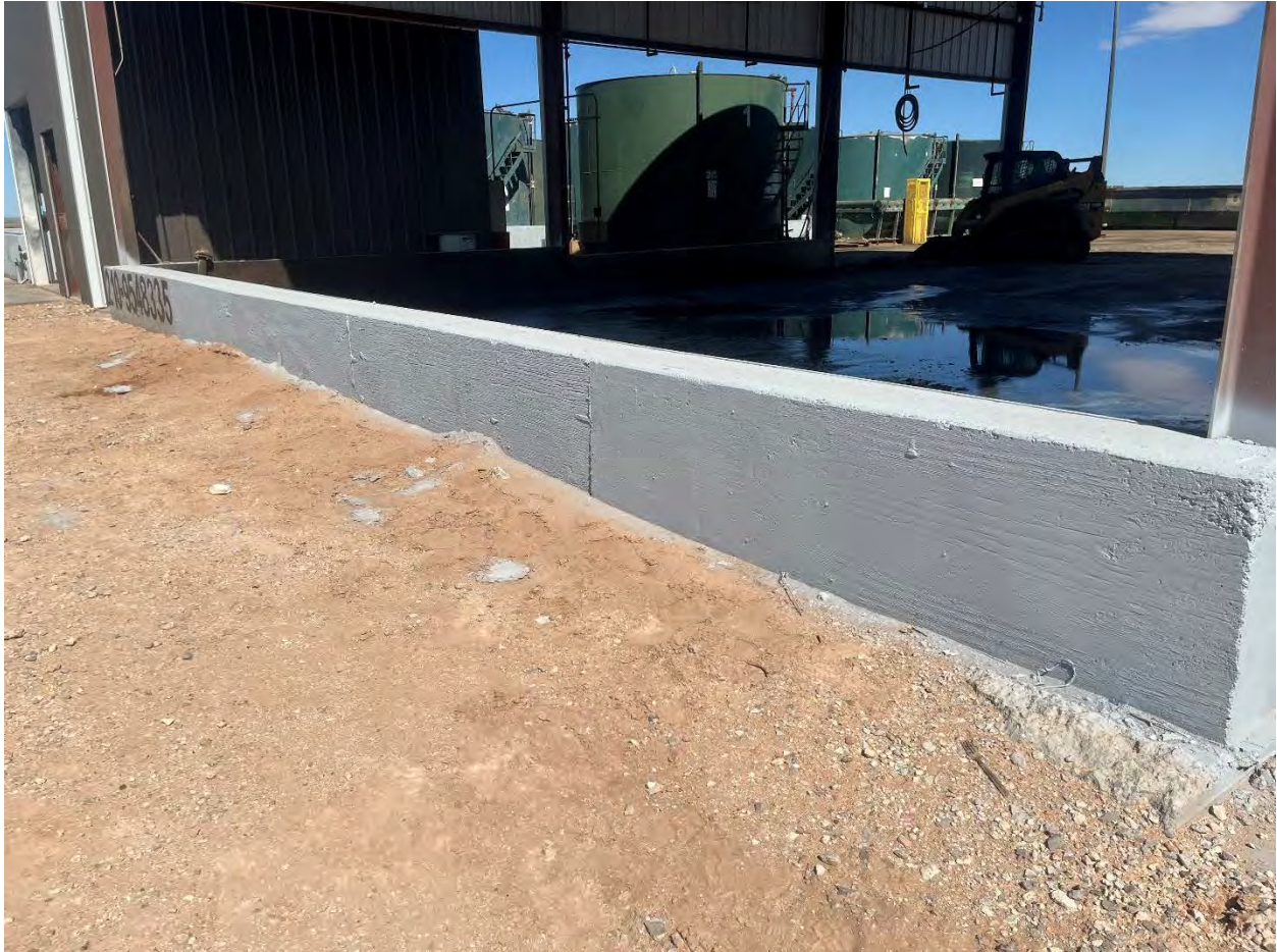
Image 10. Outer Southern Perimeter of Washout Pad
