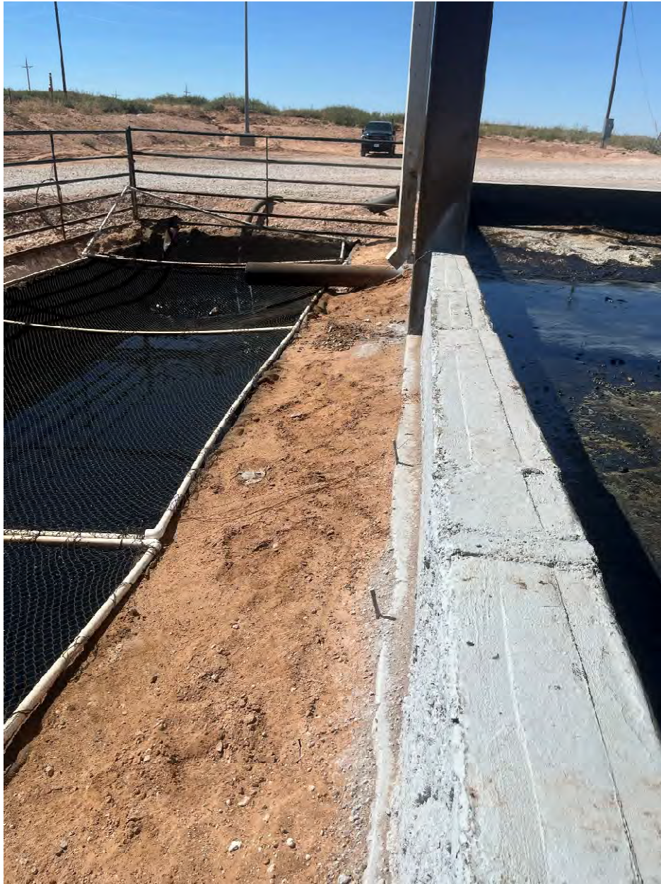
Image 9. Outer East Perimeter of Washout Pad with Steel Sumps
