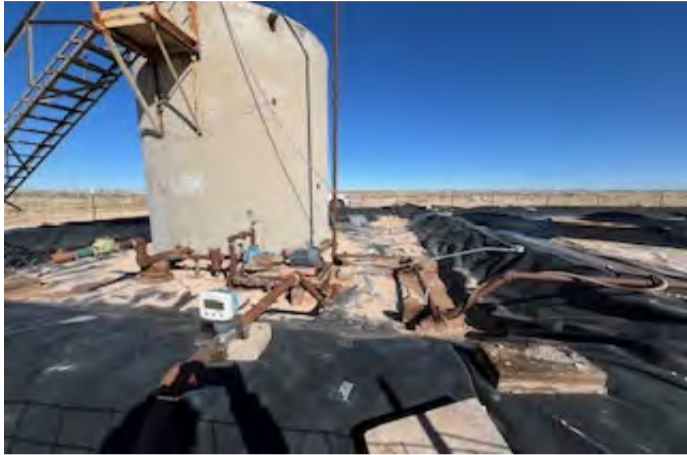
View to N of liner (2/4/26).
