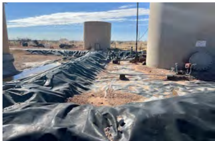
View to S of liner (2/4/26).
