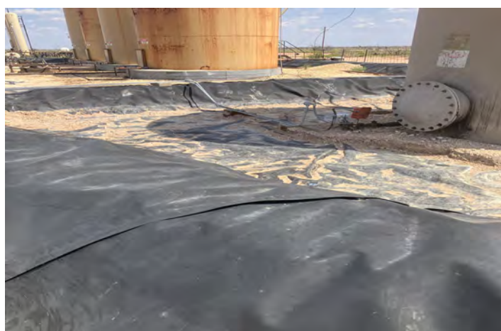
View to SE of containment (8/4/25).
