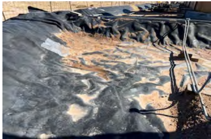
View to E of liner (2/4/26).
