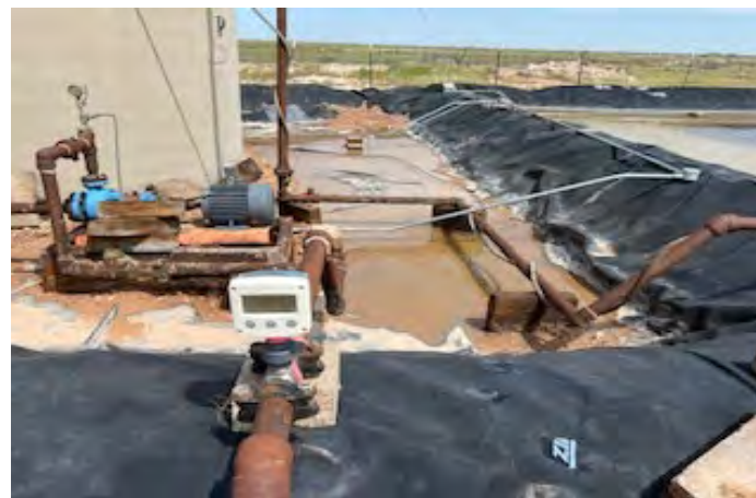
View to N of containment (9/17/25).
