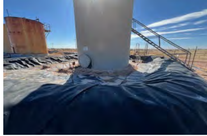
View to S of liner (2/4/26).
