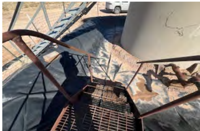
View to N of liner (2/4/26).
