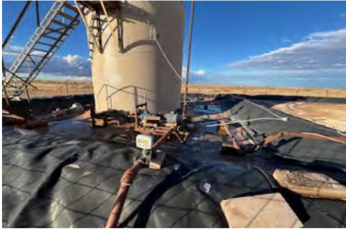
View to N of liner (11/20/25).
