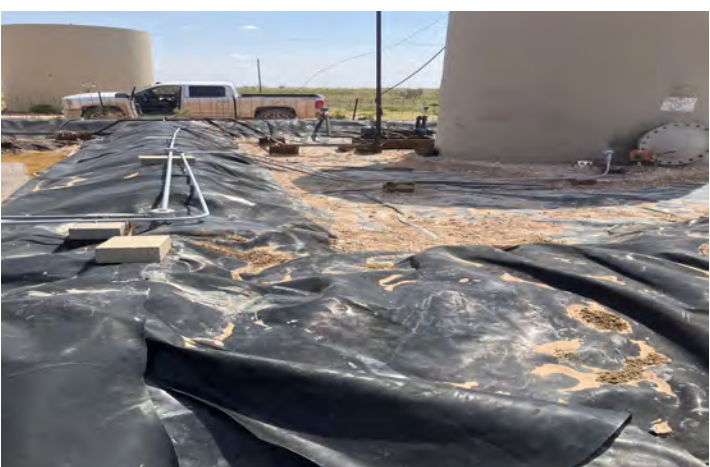
View to S of containment (8/24/25).
