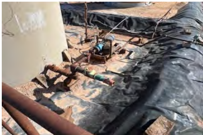
View to E of liner (2/4/26).
