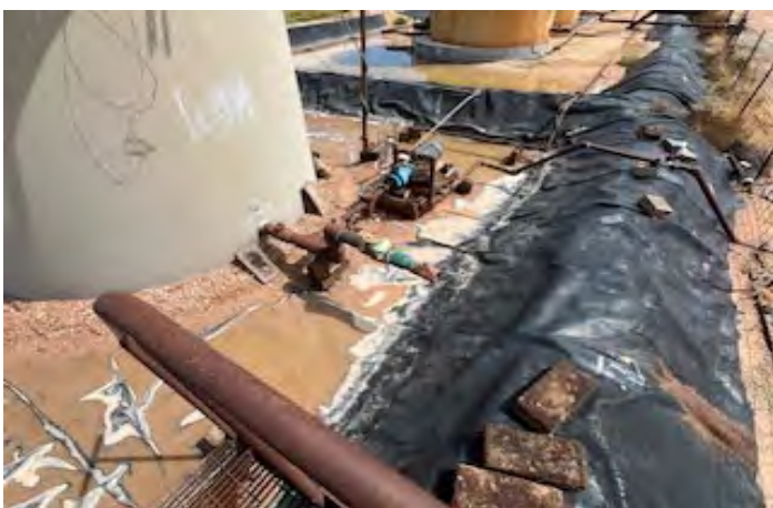
View of S side of containment (9/17/25).
