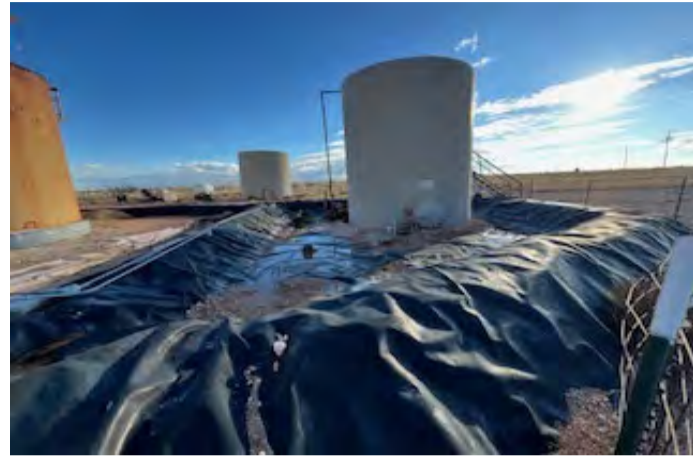
View to S of liner (11/20/25).
