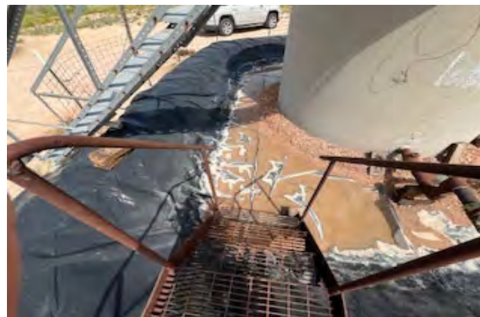
View of W side of containment (9/17/25).
