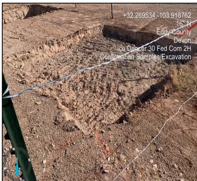
Photograph of excavated areas underlying sample points S19 & S22 facing northeast.
