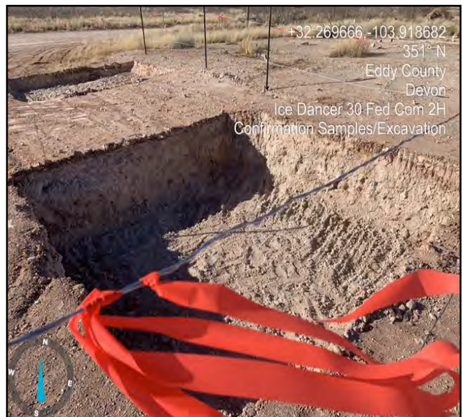
Photograph of excavated areas underlying sample points S19 & S22 facing north.
