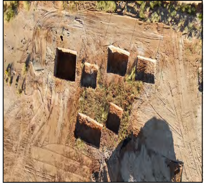
Aerial Photo taken during the excavation process.
