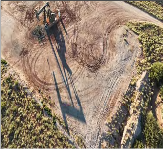
Aerial photo of the excavated area backfilled with clean material.
