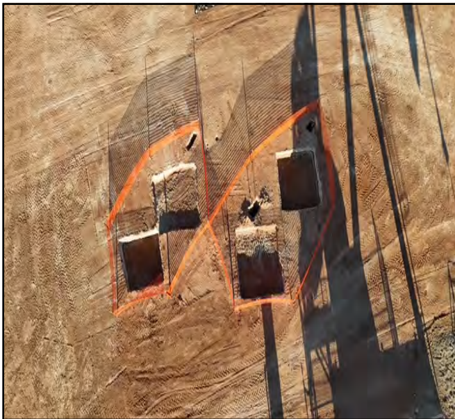
Aerial Photo taken during the excavation process.
