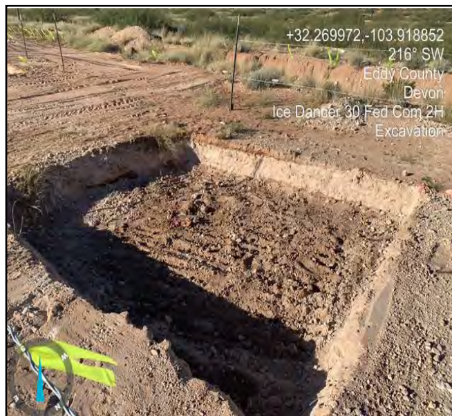
Photo taken during the excavation process facing southwest.
