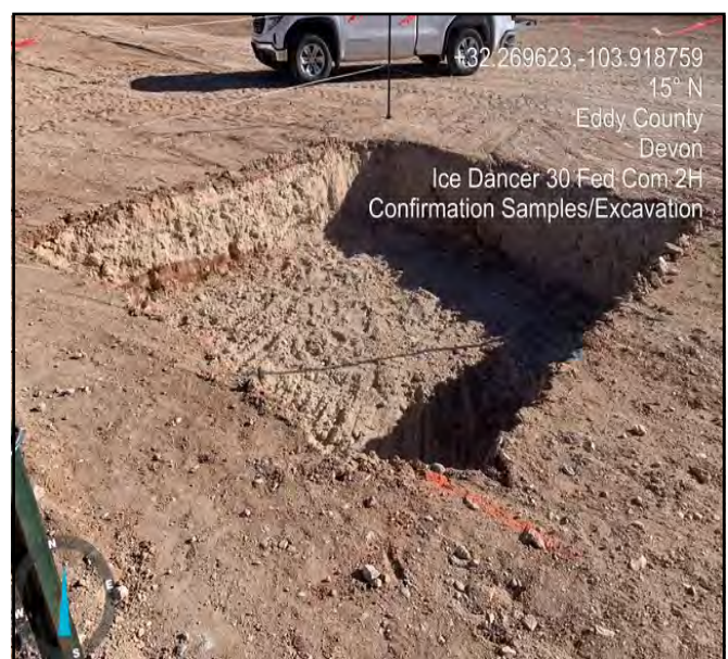
Photograph of excavated area underlying sample point S19 facing northeast.
