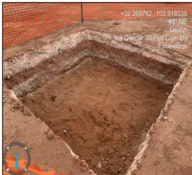
Photo taken during the excavation process facing northeast.
