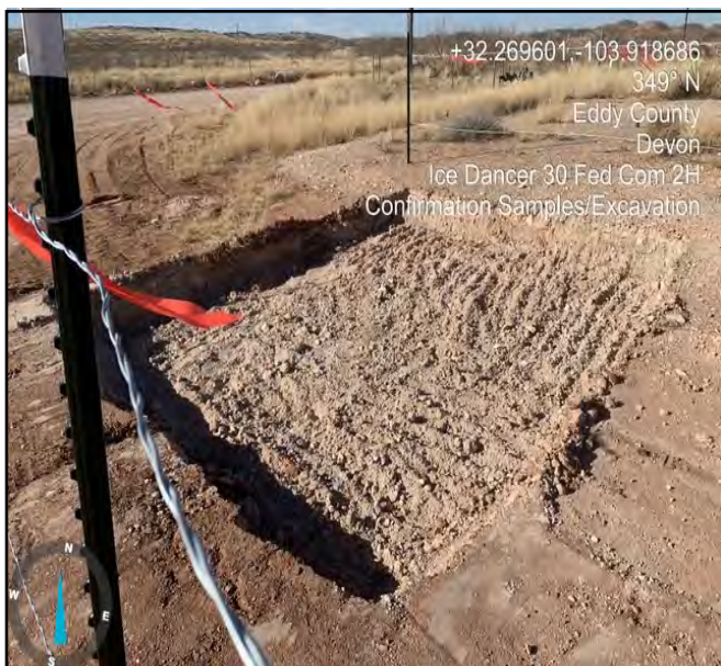
Photograph of excavated area underlying sample point S22 facing northwest.
