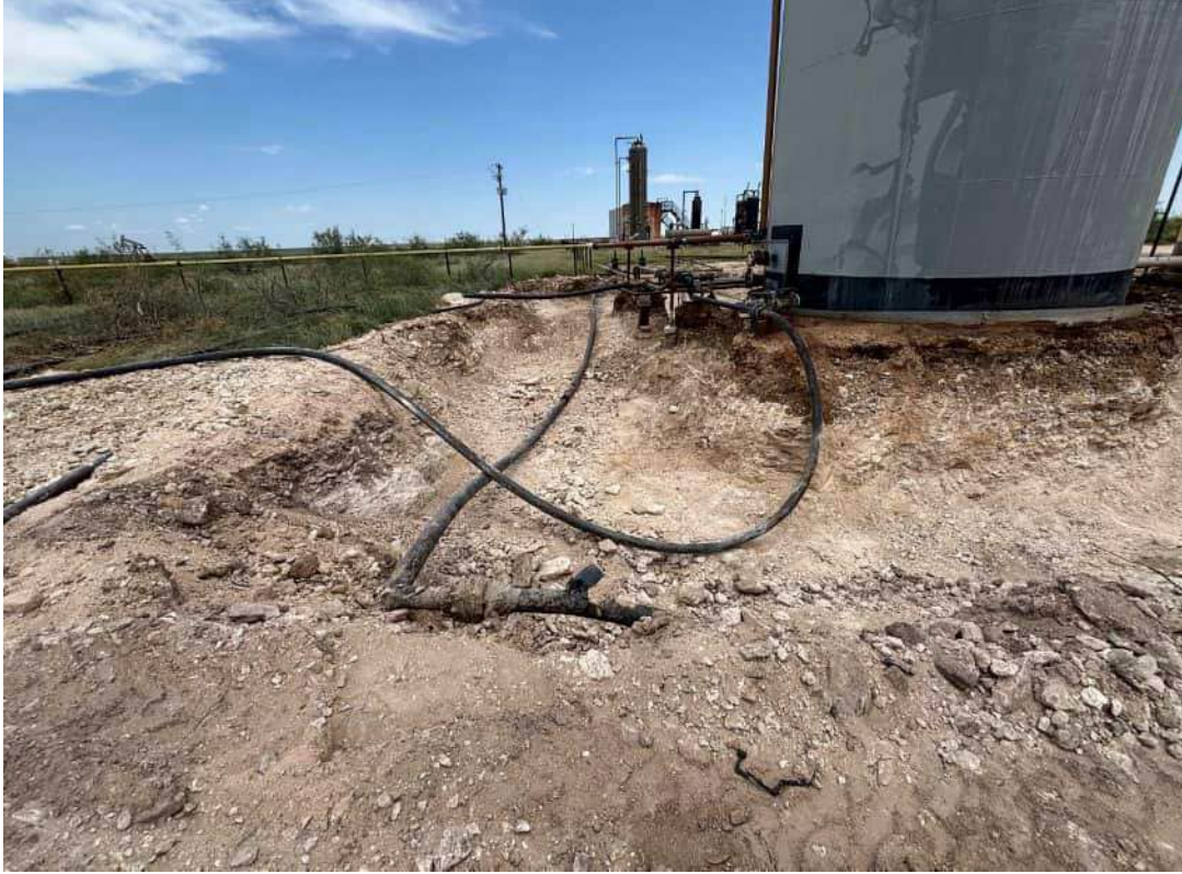
Photo 5 View of excavation from NW corner of tank battery looking E.
