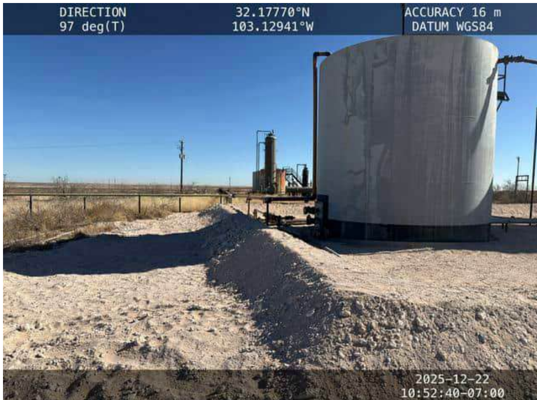
Photo 6 View from NW corner of tank battery looking E after backfilling.
