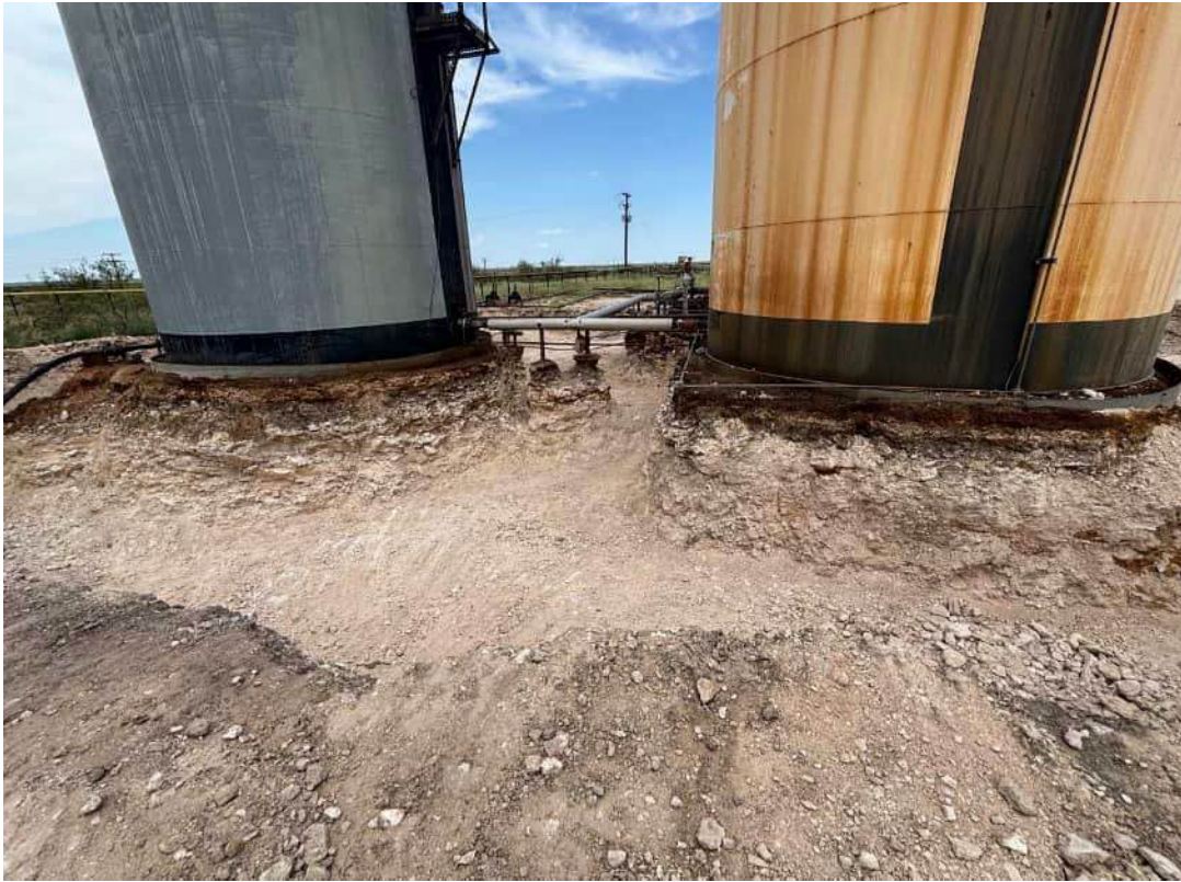
Photo 9 View of excavation from W side of tank battery looking E.
