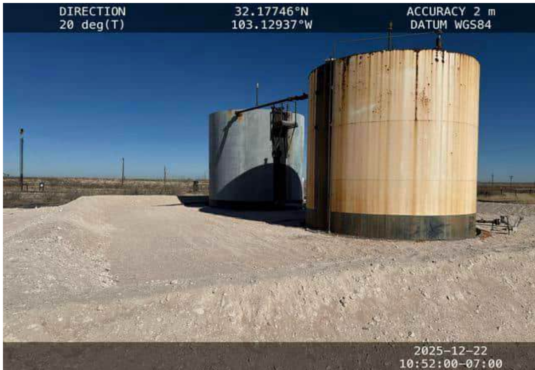
Photo 4 View from SW corner of tank battery looking N after backfilling.
