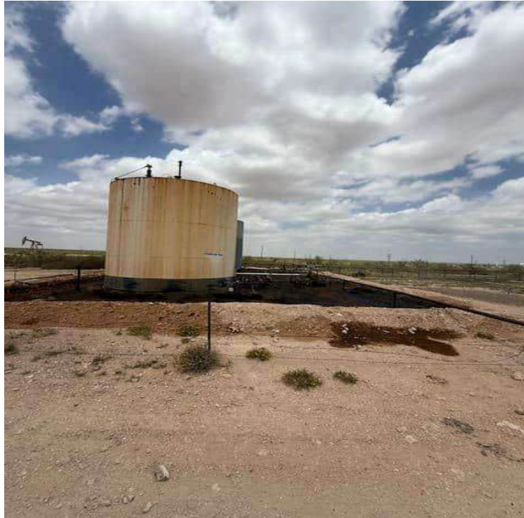
Photo 1 View of release from S side of Tank Battery looking N.
