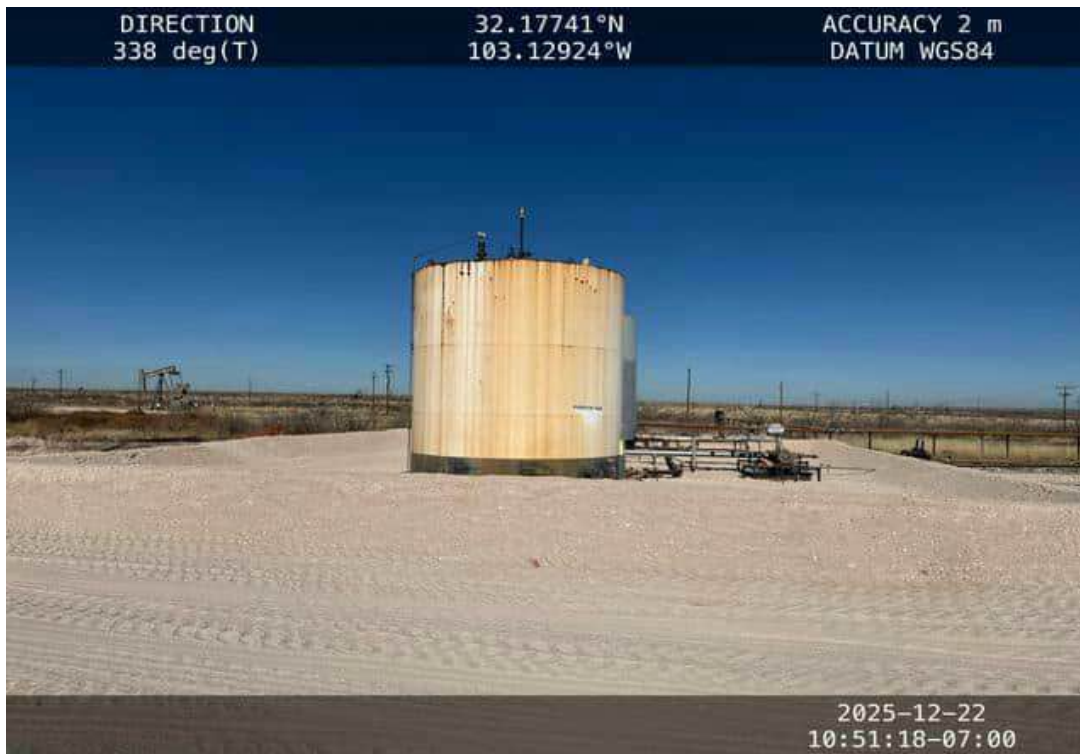
Photo 2 View from S side of Tank Battery looking N after backfilling.
