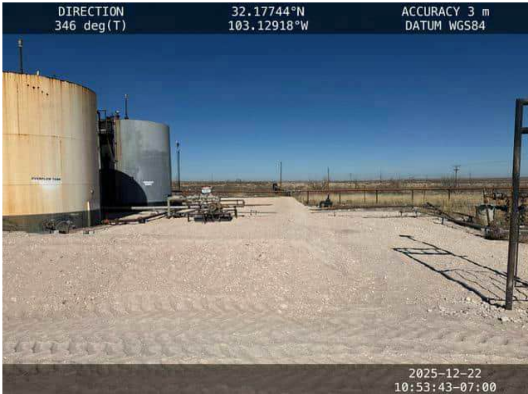
Photo 8 View from NE corner of tank battery looking N after backfilling.
