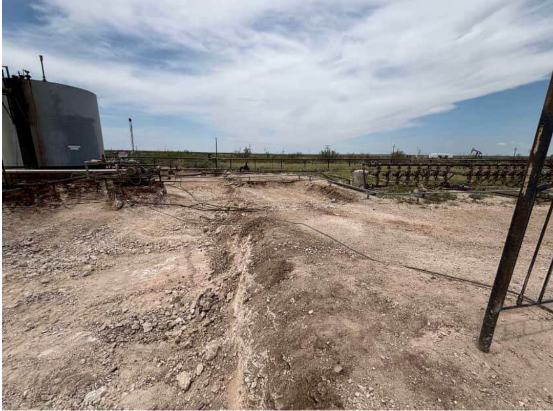
Photo 7 View of excavation from NE corner of tank battery looking N.
