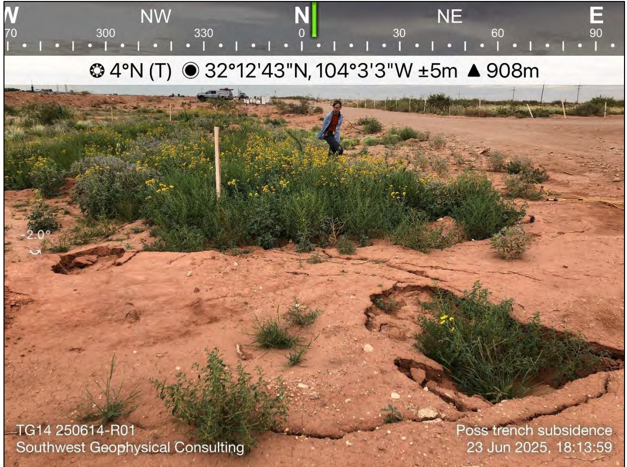
Figure 7: Feature 250614-R01. Soil subsidence within a trench.
