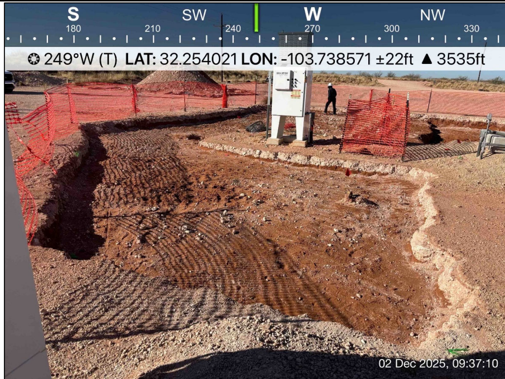
PHOTO 12: Southwestern view during excavation activities. 12/2/2025
