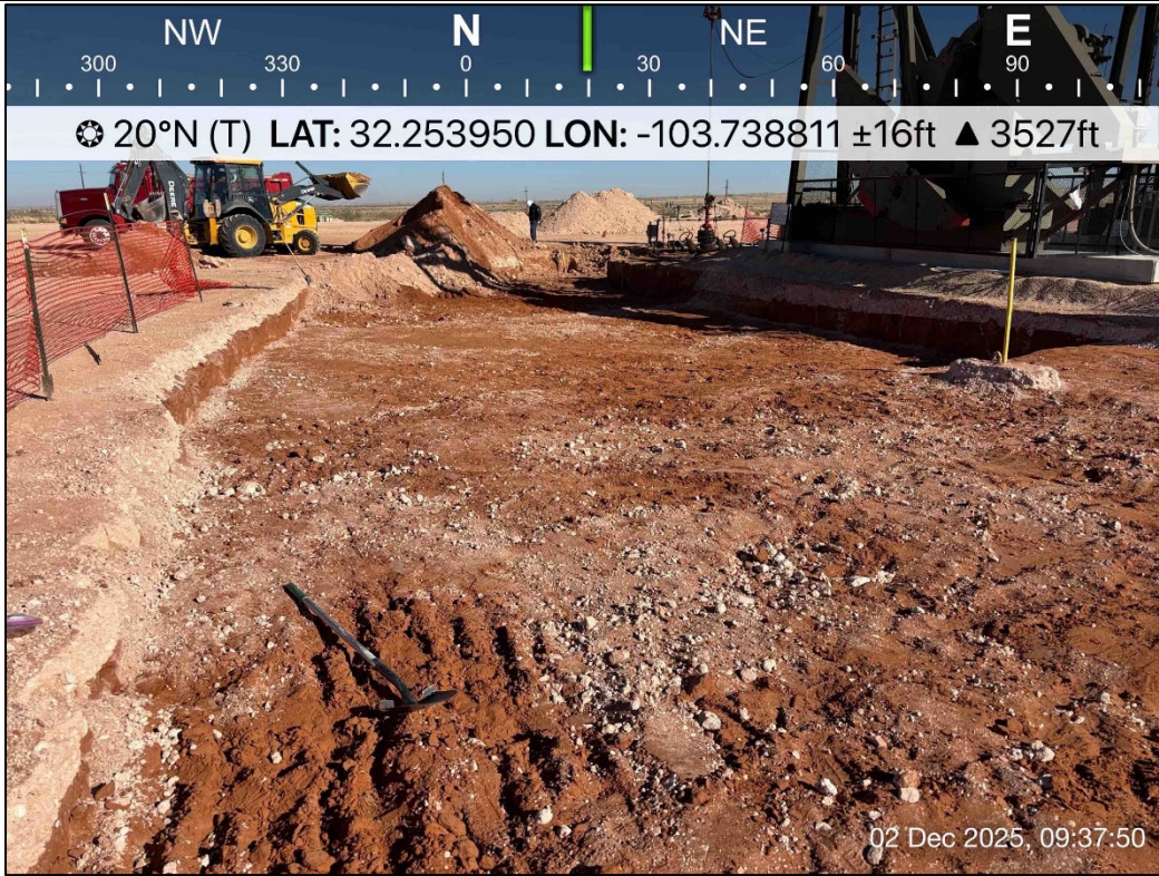
PHOTO 13: Northeastern view during excavation activities. 12/2/2025
