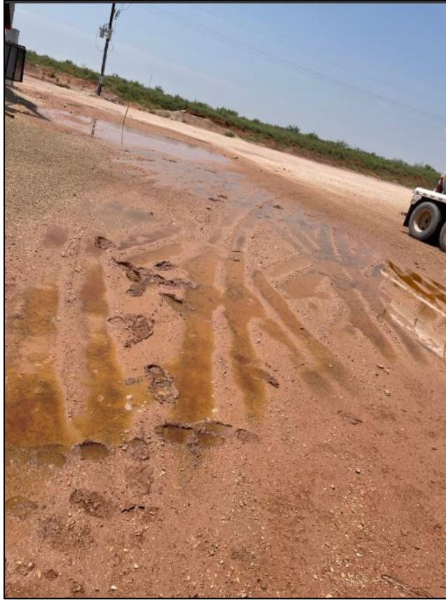
PHOTO 1: Southwestern view during initial site assessment by Devon. 6/10/2025
