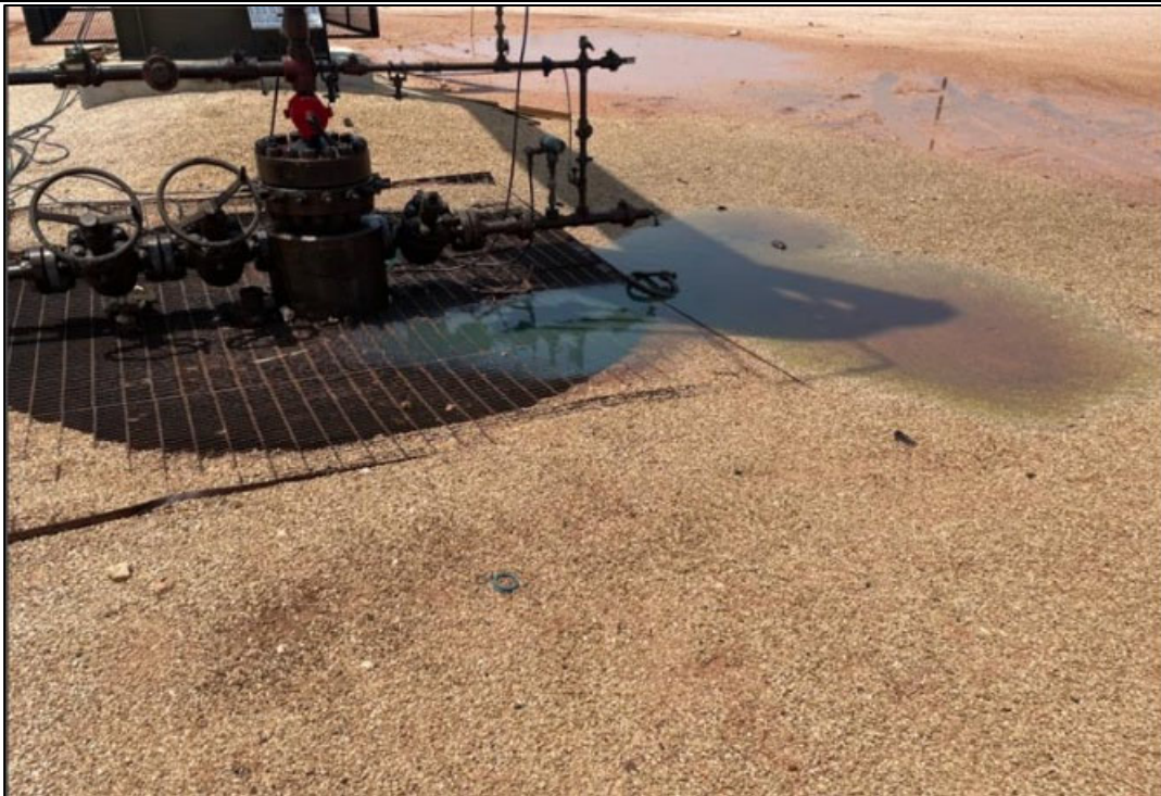
PHOTO 2: Southwestern view during initial site assessment by Devon. 6/10/2025
