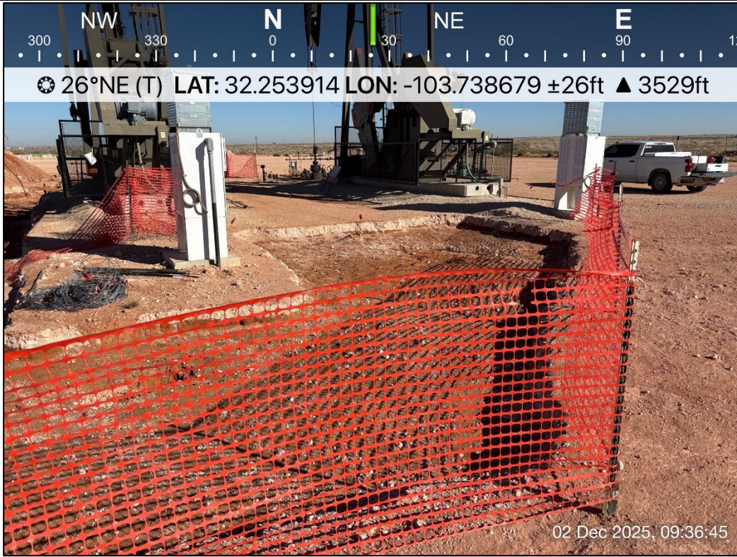
PHOTO 11: Northeastern view during excavation activities. 12/2/2025
