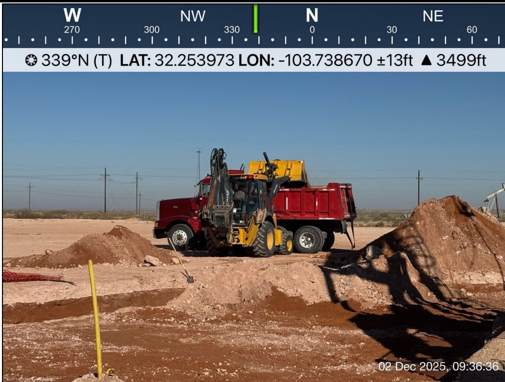
PHOTO 14: Northwestern view during excavation activities. 12/2/2025
