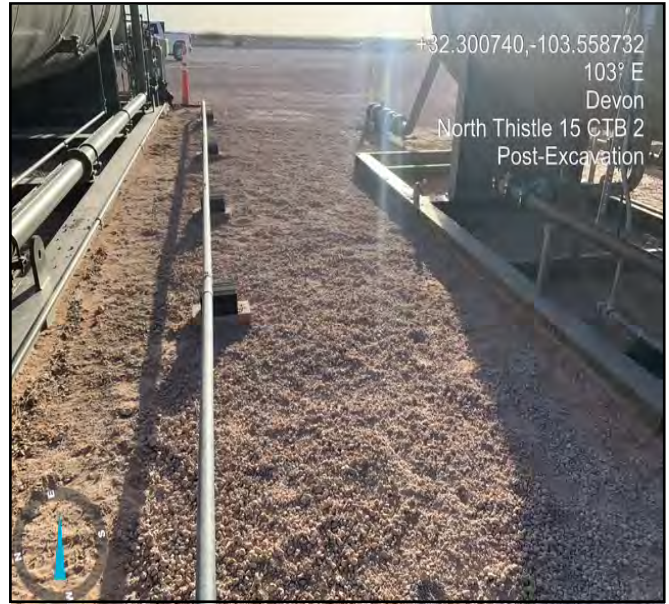
Photo taken post excavation facing east.
