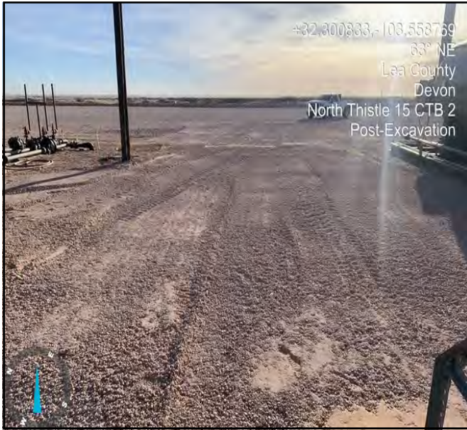
Photo taken post excavation facing northeast.
