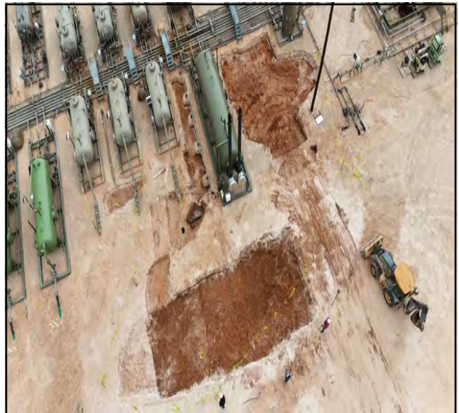
Aerial photo taken during the excavation process.
