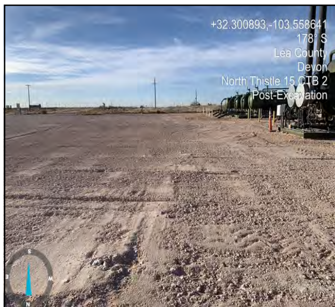
Photo taken post excavation facing south.
