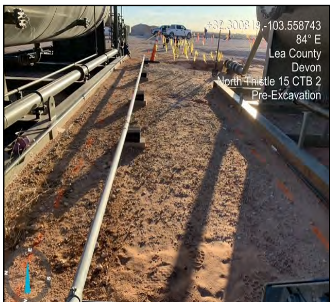
Photograph taken pre excavation process facing east.
