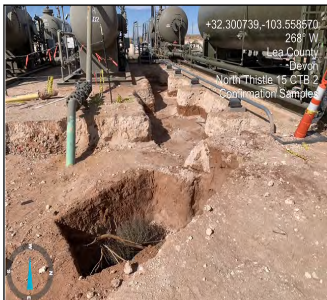
Photograph taken during confirmation sampling facing west.
