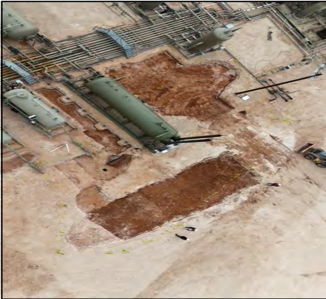
Aerial photo taken during the excavation process.
