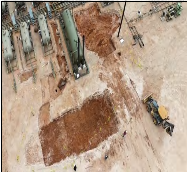
Aerial photo taken during the excavation process.
