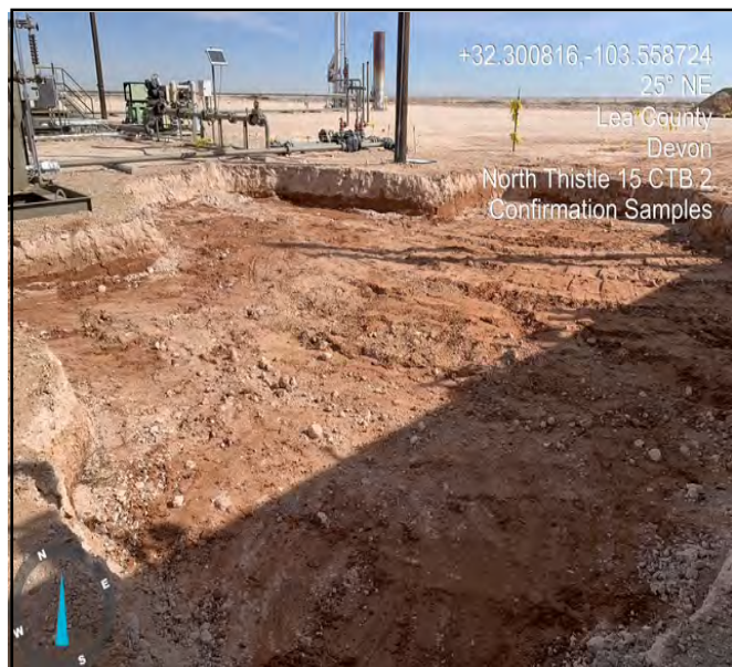
Photograph taken during confirmation sampling facing northeast.
