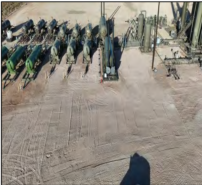
Aerial photo taken post excavation.
