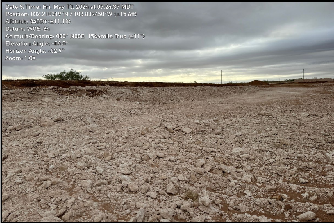
Excavated release area during remediation activities, facing northeast (05/10/2024).
