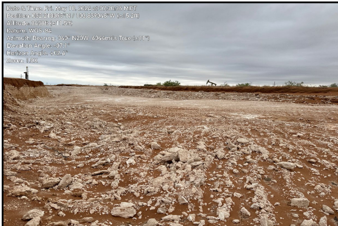
Excavated release area during remediation activities, facing northwest (05/10/2024).
