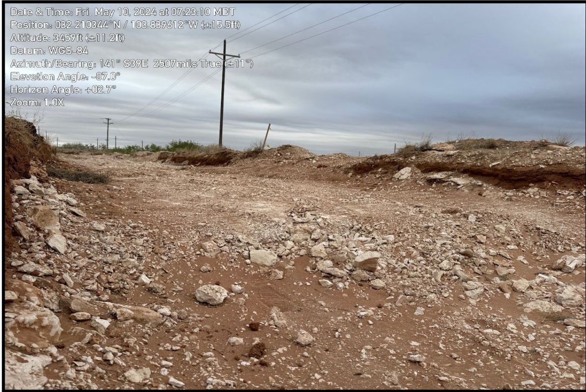
Excavated release area during remediation activities, facing southeast (05/10/2024).
