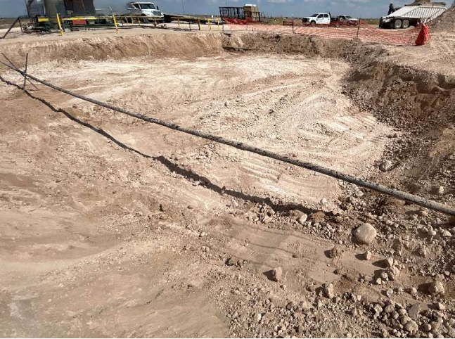
Photograph 11 Date: 08/21/2025 Description: Southeastern view of on-pad excavation activities.
