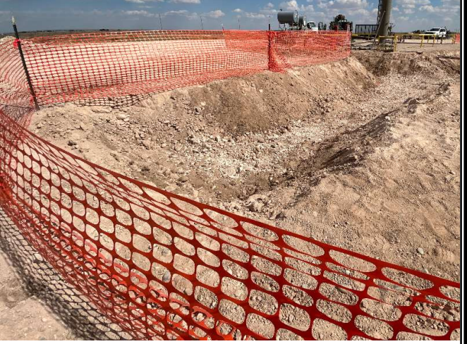
Photograph 8 Date: 08/21/2025 Description: Southeastern view of on-pad excavation activities.
