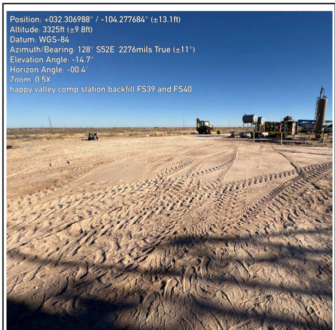
Photograph 20 Date: 11/25/2025 Description: Southeastern view of on-pad backfill.
