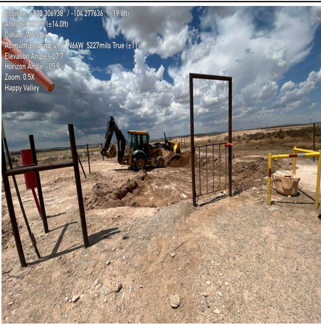
Photograph 3 Date: 08/15/2025 Description: Northwestern view of on-pad excavation activities.
