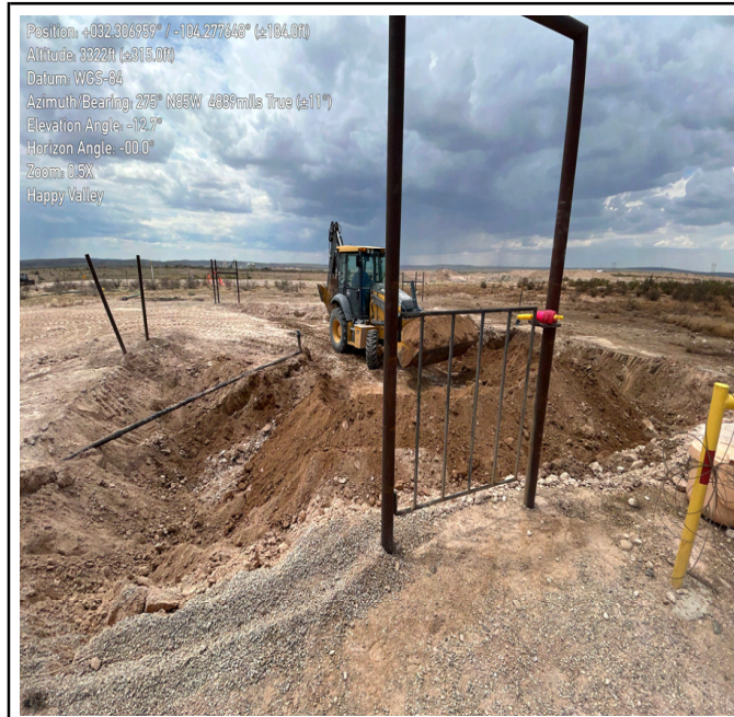
Photograph 4 Date: 08/15/2025 Description: Northwestern view of on-pad excavation activities.
