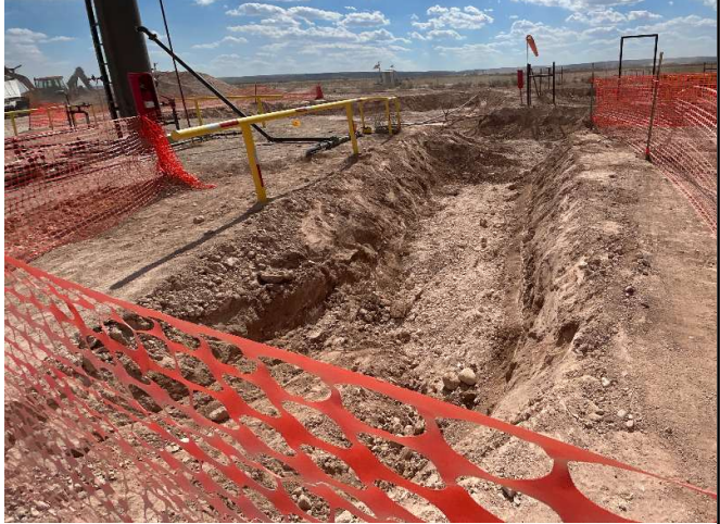
Photograph 12 Date: 08/21/2025 Description: Southwestern view of on-pad excavation activities.
