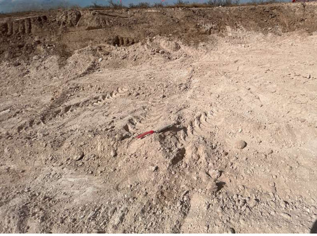
Photograph 7 Date: 08/21/2025 Description: Northeastern view of on-pad excavation activities.
