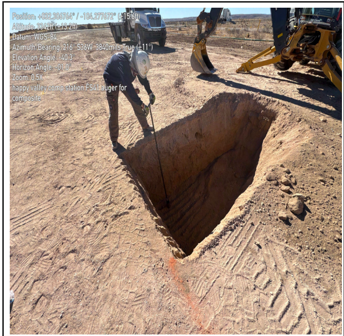
Photograph 18 Date: 11/25/2025 Description: Southwestern view of excavation confirmation sampling activities.
