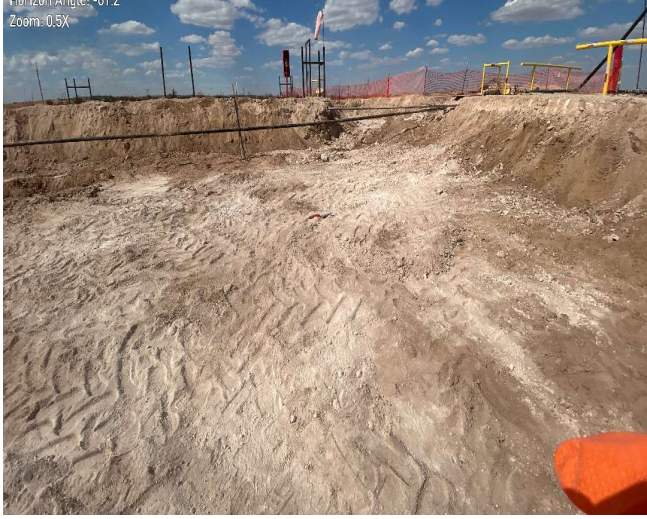
Photograph 9 Date: 08/21/2025 Description: Northeastern view of on-pad excavation activities.
