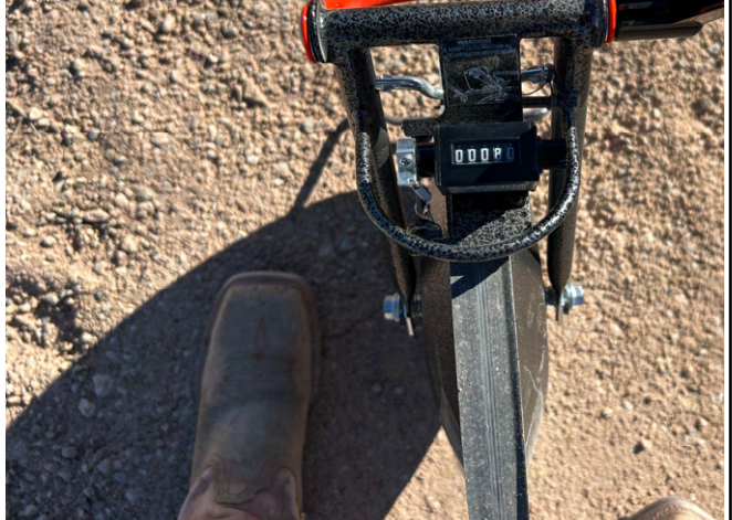
Photograph 16 Date: 11/12/2025 Description: Southeastern view of excavation measurement activities.
