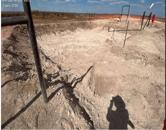
Photograph 10 Date: 08/21/2025 Description: Northeastern view of on-pad excavation activities.
