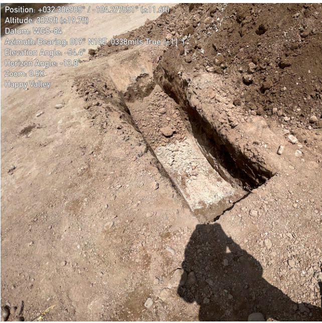
Photograph 1 Date: 08/15/2025 Description: Northeastern view of on-pad delineation activities
