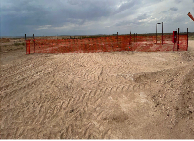
Photograph 5 Date: 08/15/2025 Description: Northwestern view of on-pad excavation activities.
