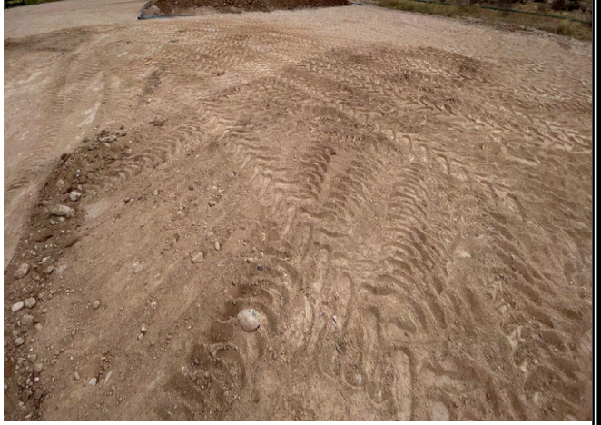
Photograph 6 Date: 08/15/2025 Description: Southwestern view of excavation backfill.
