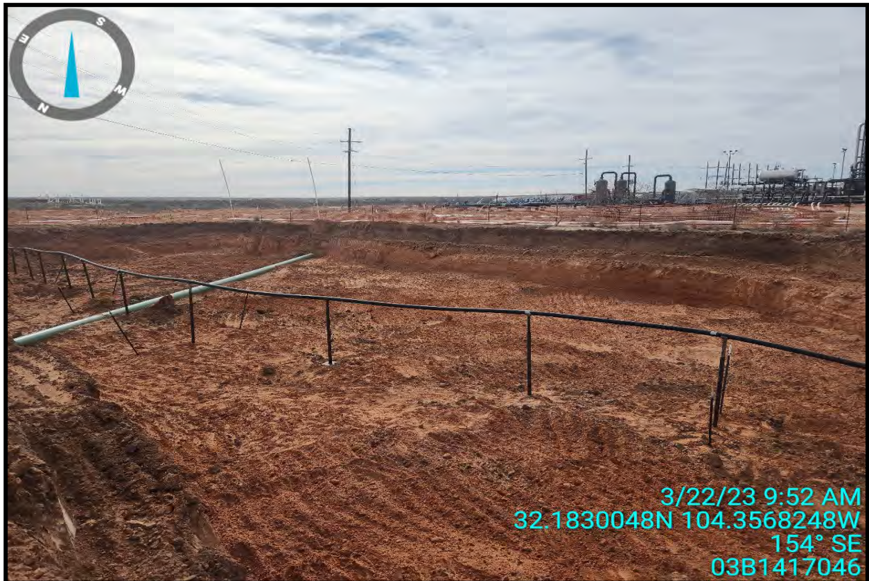
View of excavation area, facing southeast.
