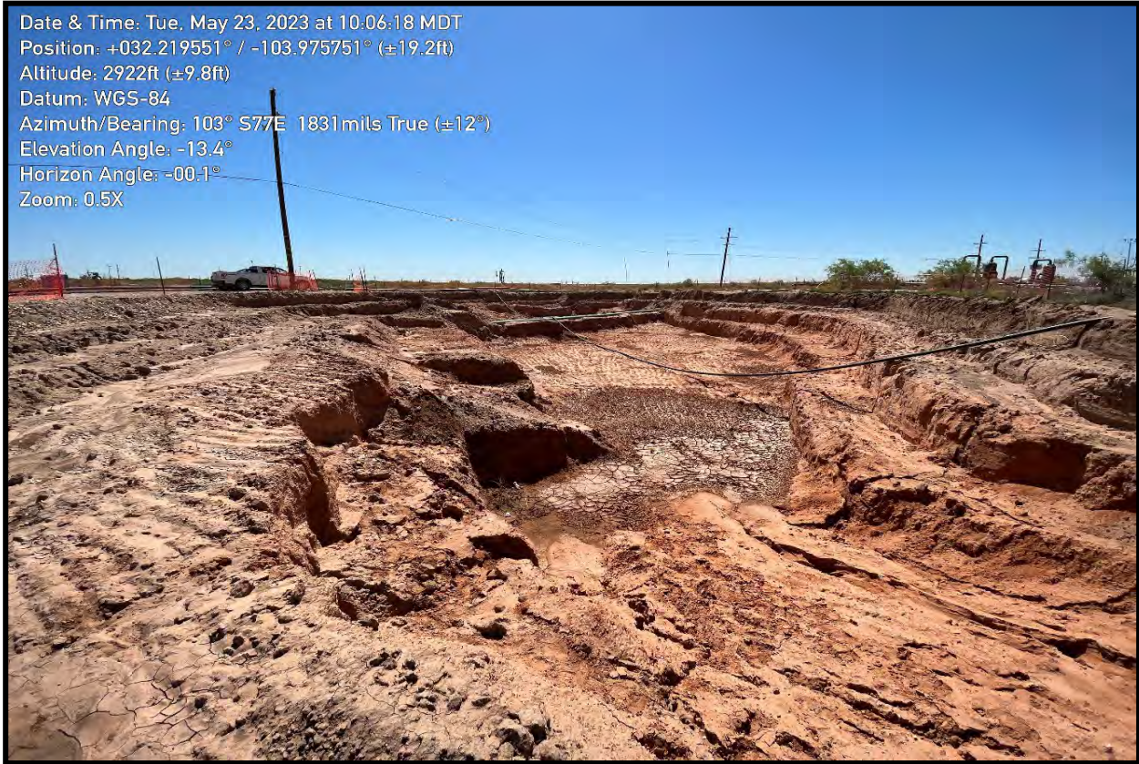
View of excavation area, facing southeast.
