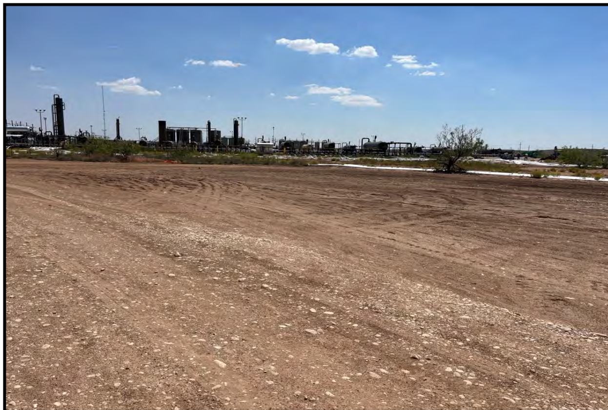
View of excavation area subsequent to backfill, facing south.
