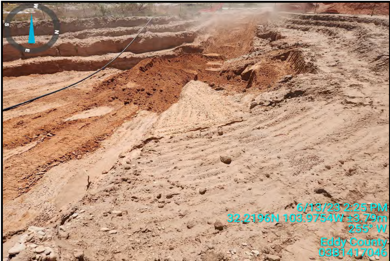
View of excavation area, facing southwest.
