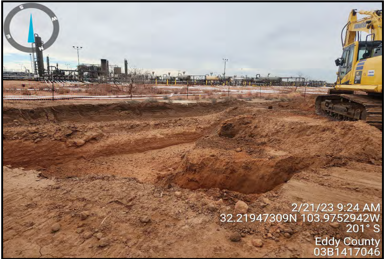
View of excavation area, facing southwest.
