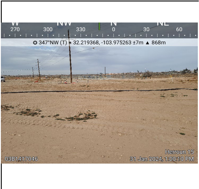
Photograph 2 Date: 1/31/2024 Description: Backfilled excavation/Reclamation area View: North
