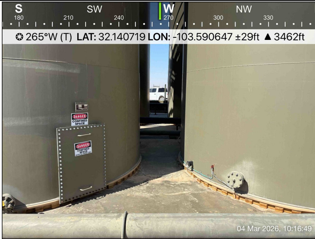
PHOTO 23: Western view during liner inspection activities. 3/4/2026
