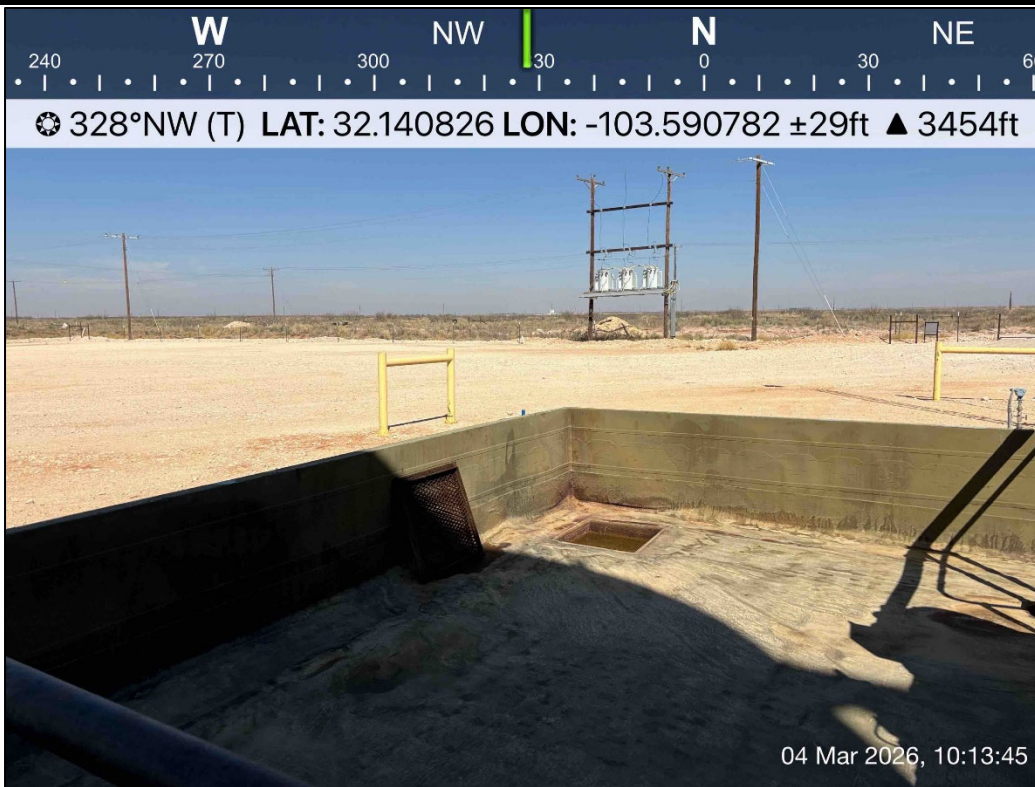
PHOTO 14: Northwestern view during liner inspection activities. 3/4/2026
