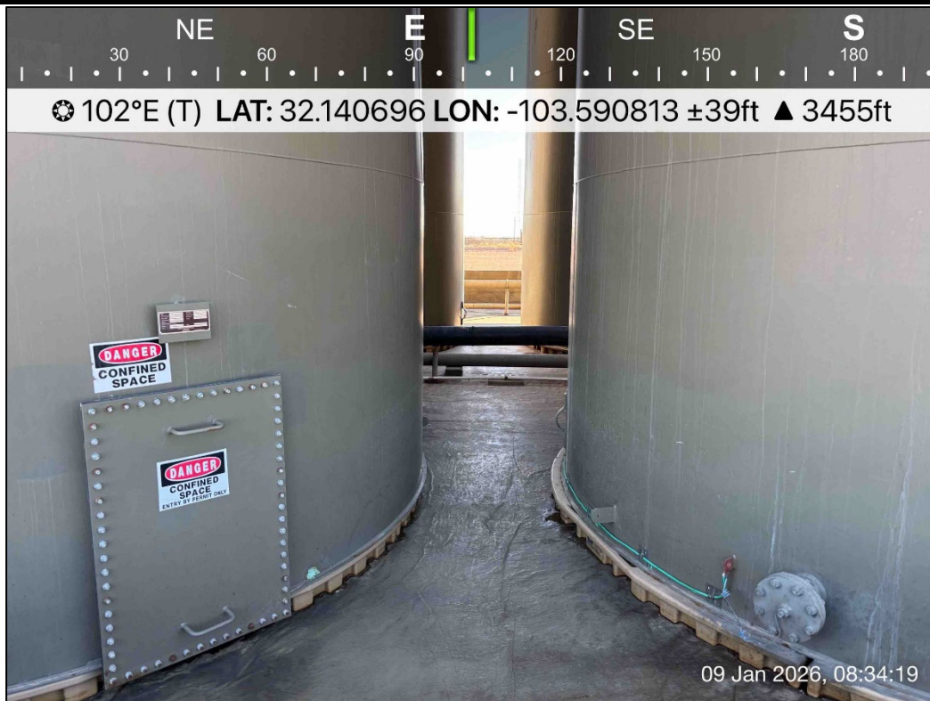
PHOTO 12: Southeastern view during liner inspection activities. 3/4/2026
