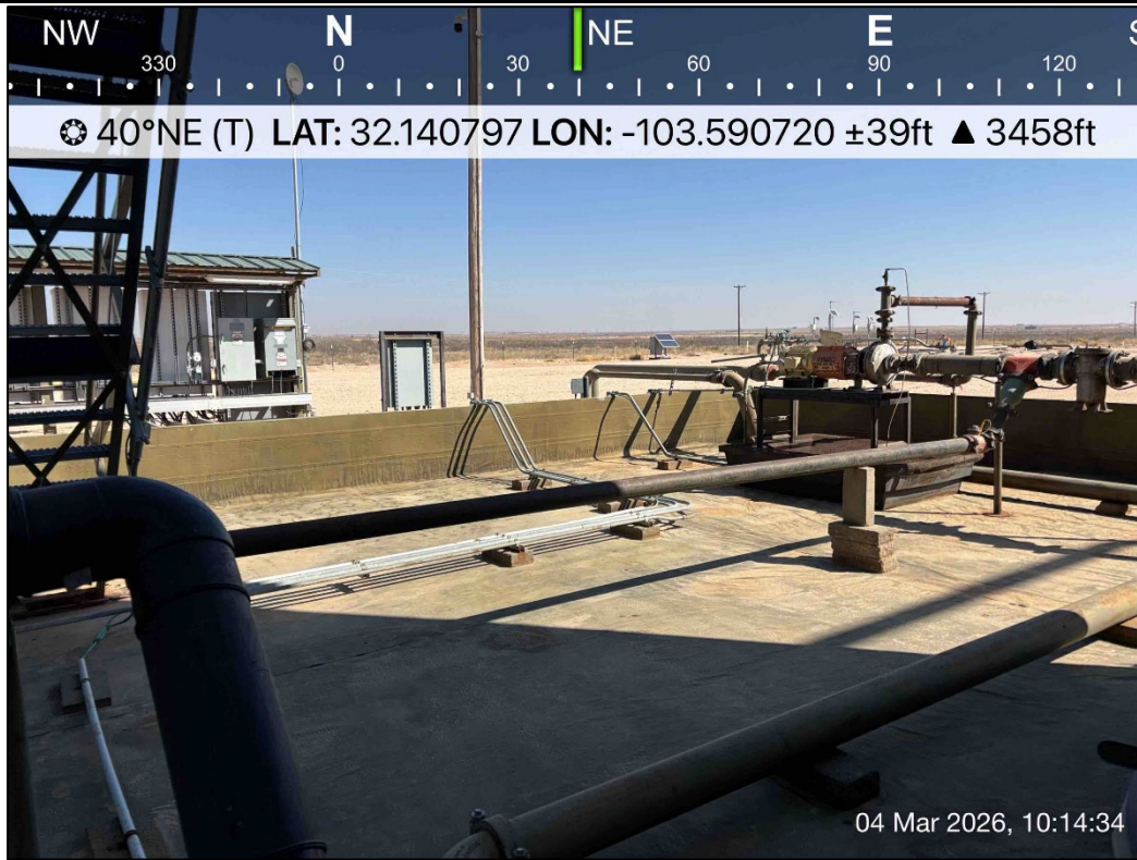
PHOTO 17: Northeastern view during liner inspection activities. 3/4/2026
