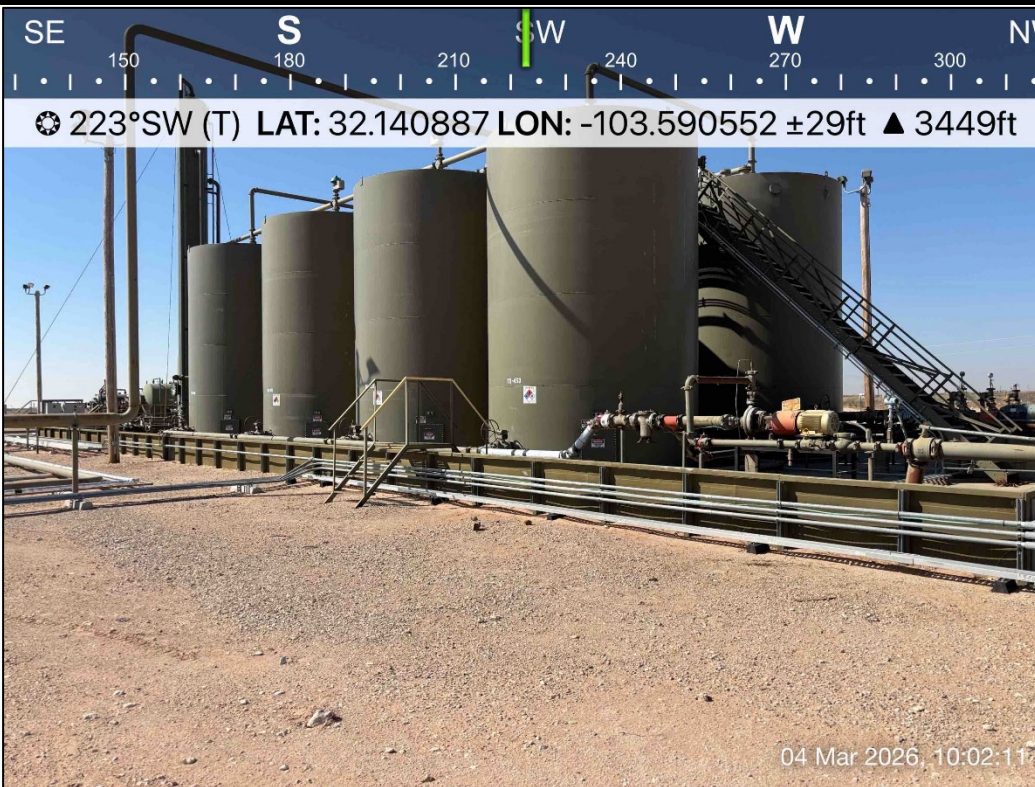
PHOTO 6: Southwestern view outside of containment during liner inspection activities. 3/4/2026
