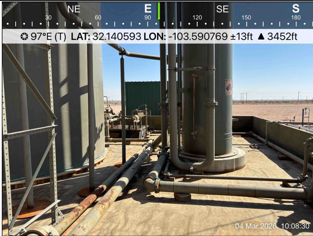
PHOTO 7: Eastern view outside of containment during liner inspection activities. 3/4/2026
