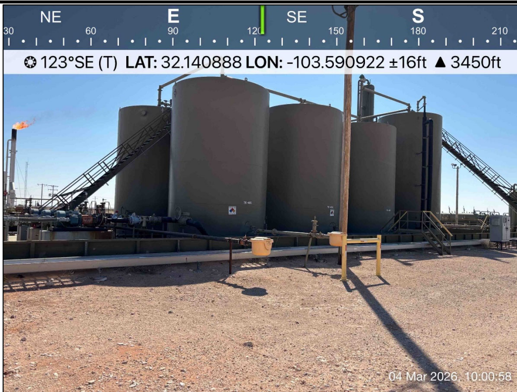
PHOTO 4: Southeastern view outside of containment during liner inspection activities. 3/4/2026
