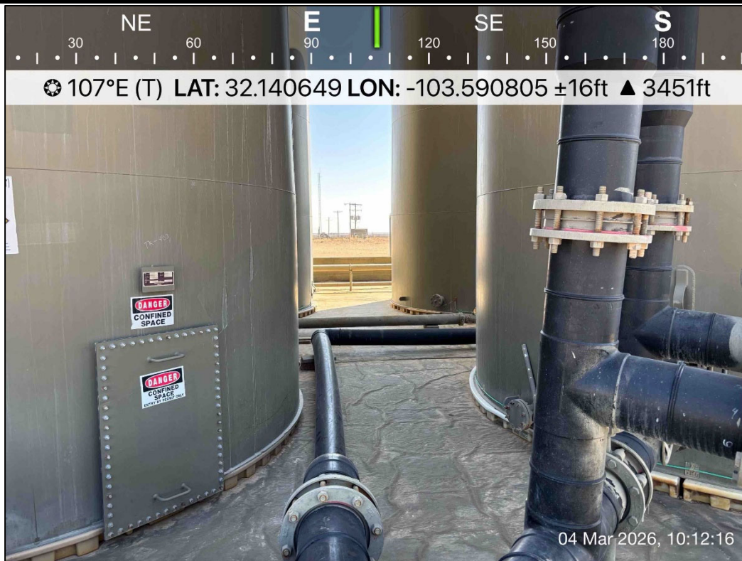
PHOTO 10: Southeastern view during liner inspection activities. 3/4/2026
