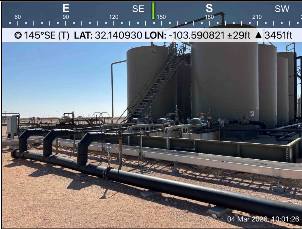
PHOTO 5: Southeastern view outside of containment during liner inspection activities. 3/4/2026
