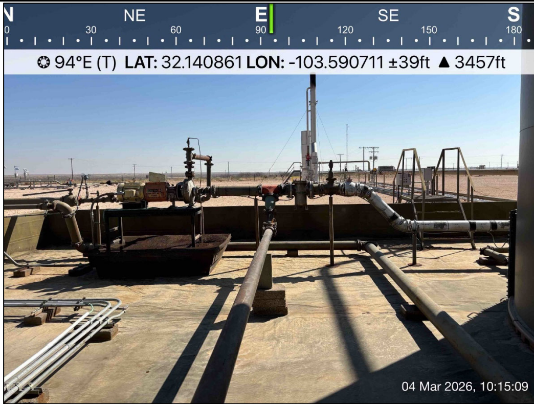
PHOTO 19: Eastern view during liner inspection activities. 3/4/2026
