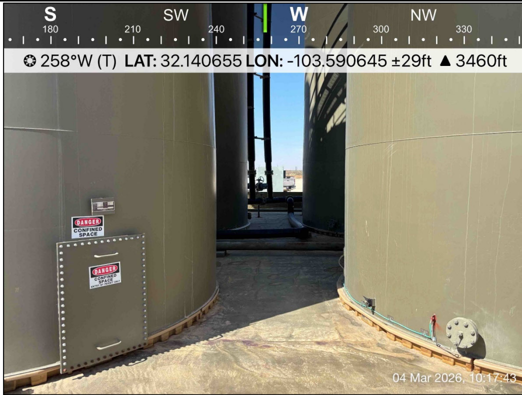
PHOTO 25: Southwestern view during liner inspection activities. 3/4/2026
