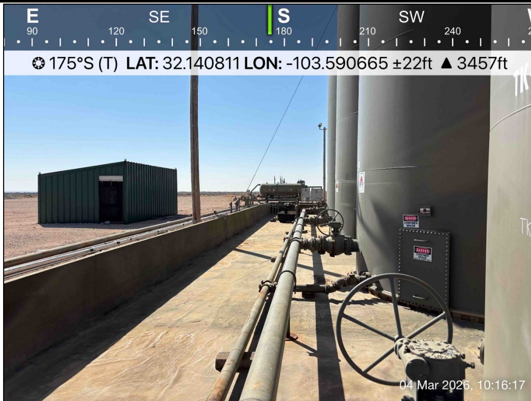
PHOTO 20: Southern view during liner inspection activities. 3/4/2026
