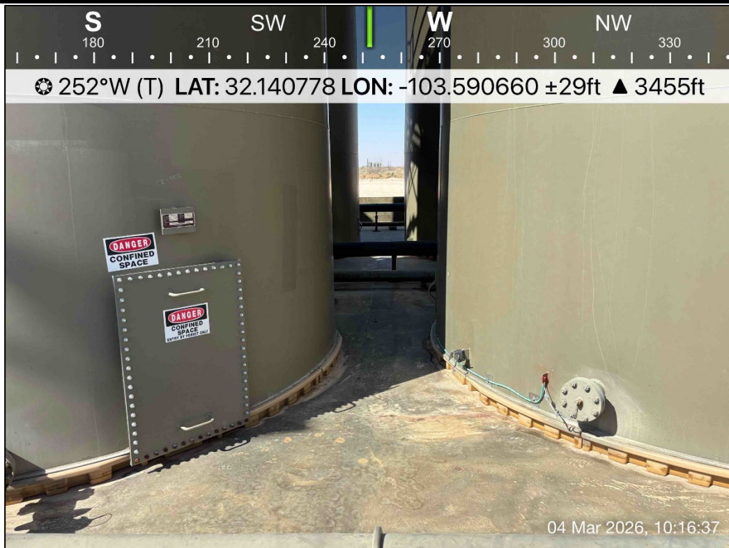
PHOTO 22: Southwestern view during liner inspection activities. 3/4/2026
