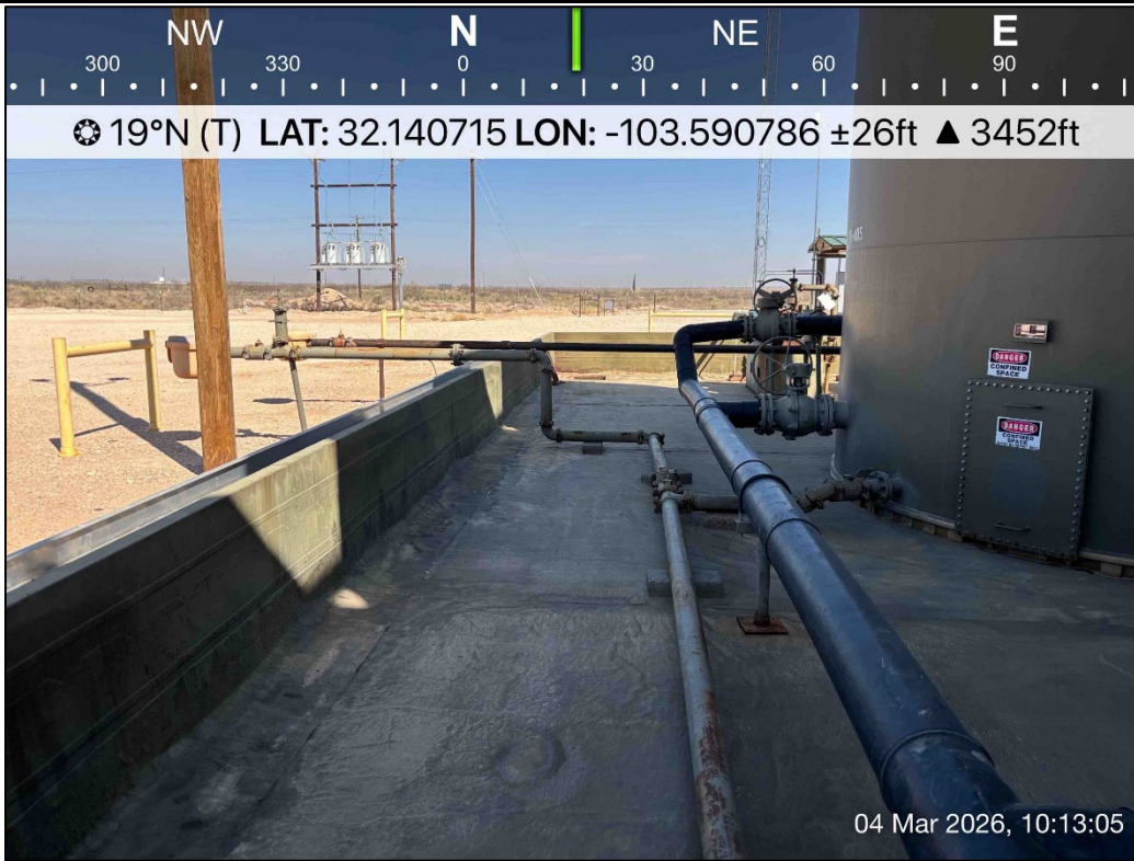
PHOTO 13: Northeastern view during liner inspection activities. 3/4/2026
