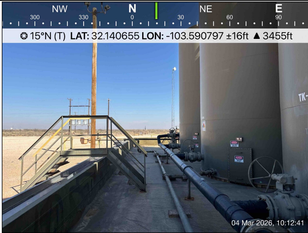
PHOTO 11: Northeastern view during liner inspection activities. 3/4/2026
