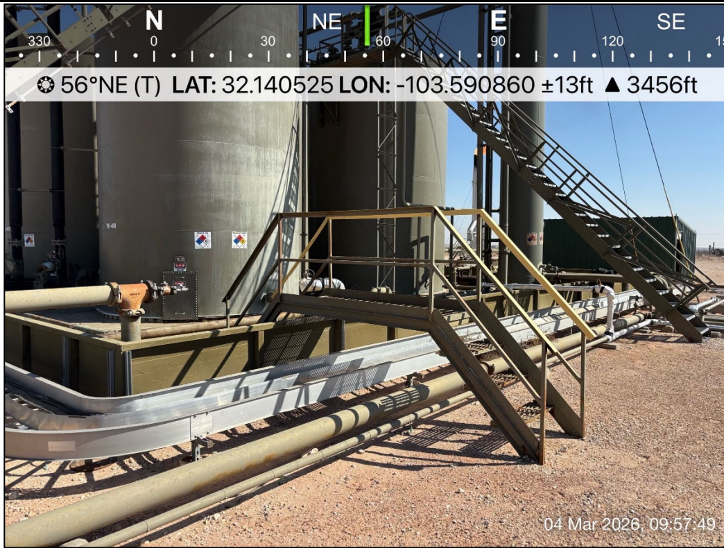
PHOTO 3: Northeastern view outside of containment during liner inspection activities. 3/4/2026
