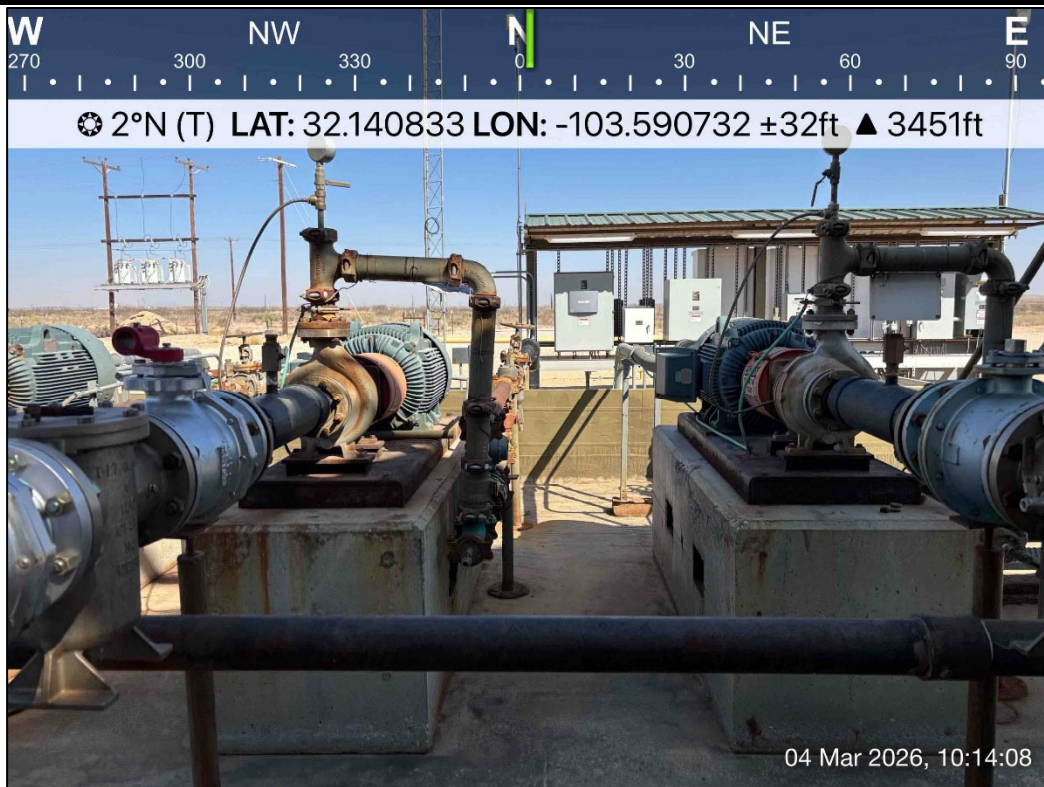
PHOTO 16: Northern view during liner inspection activities. 3/4/2026
