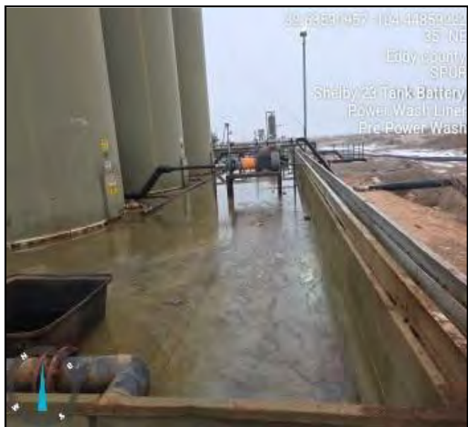
Photo taken pre powerwash facing northeast.
