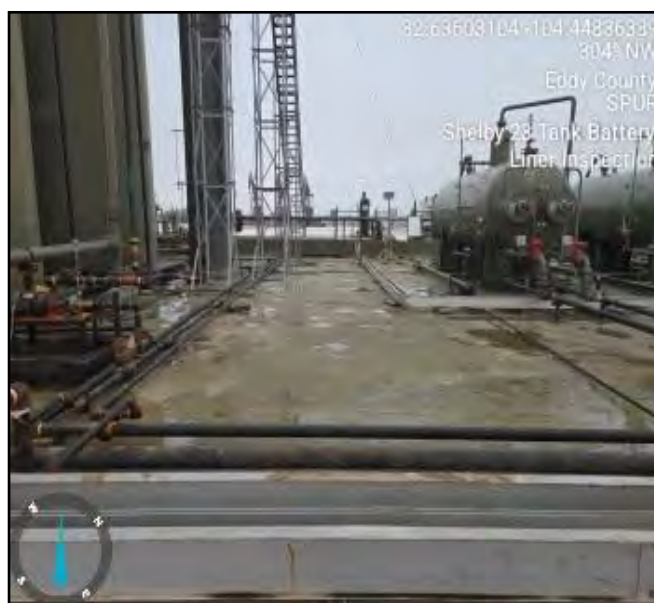
Photograph taken during liner inspection facing northwest.
