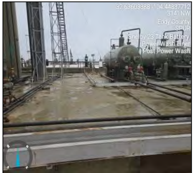
Photos taken post powerwash facing northwest.
