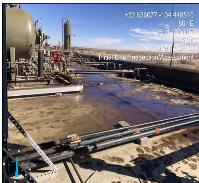
Photo taken during the initial assessment facing east.
