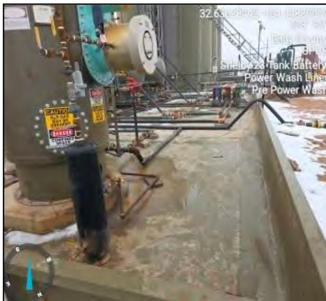
Photo taken pre powerwash facing southwest.
