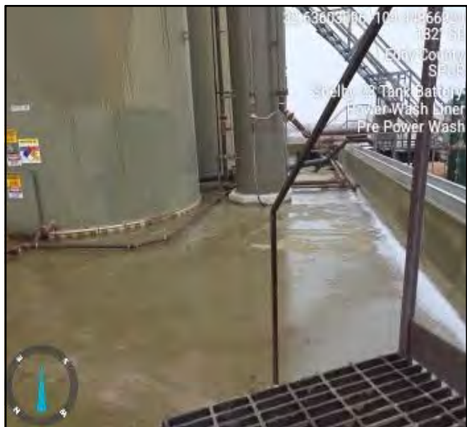
Photo taken pre powerwash facing southeast.
