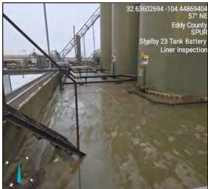
Photograph taken during liner inspection facing northeast.
