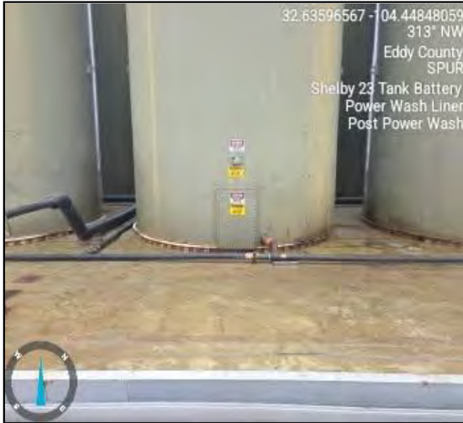
Photos taken post powerwash facing northwest.
