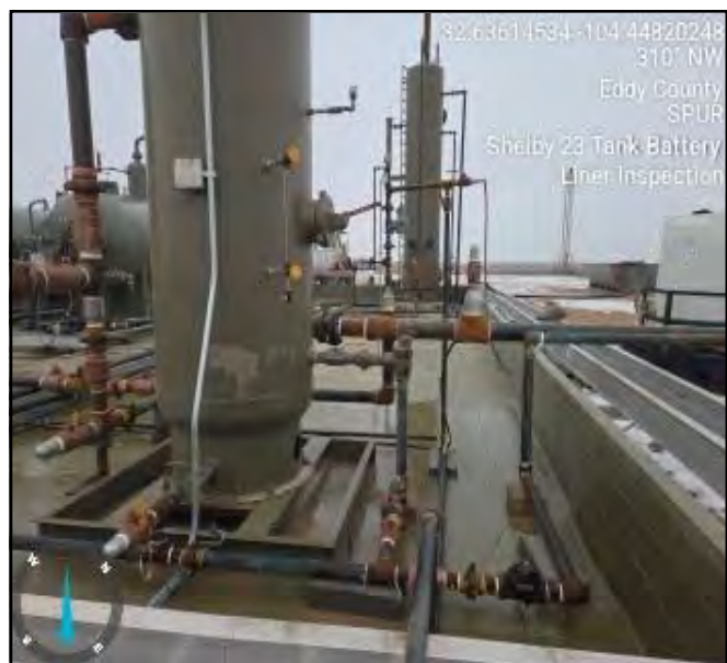
Photograph taken during liner inspection facing northwest.
