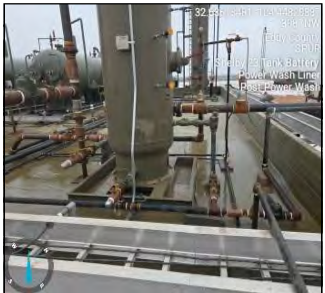
Photos taken post powerwash facing northwest.
