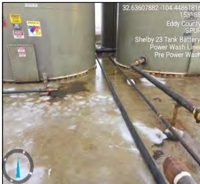
Photo taken pre powerwash facing southeast.
