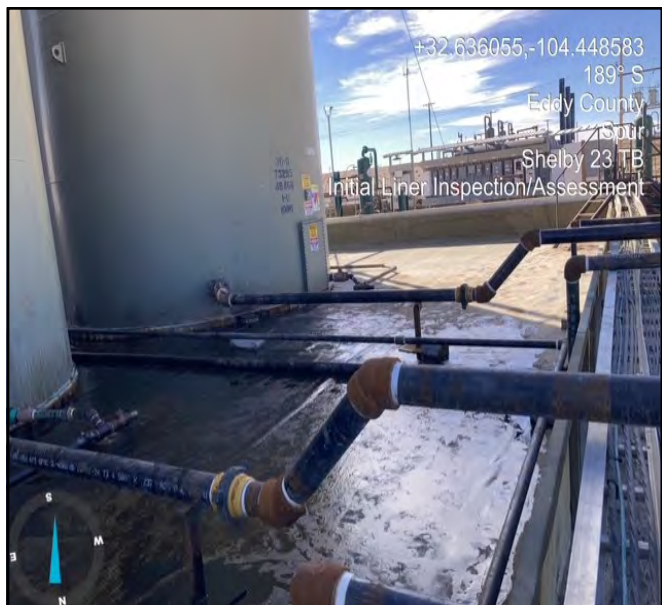
Photo taken during the initial assessment facing south.
