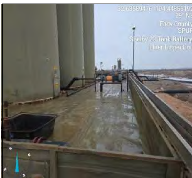
Photograph taken during liner inspection facing northeast.
