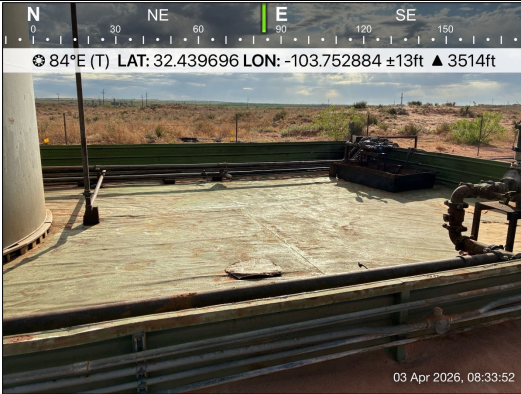
PHOTO 11: Eastern view during liner inspection activities. 4/3/2026
