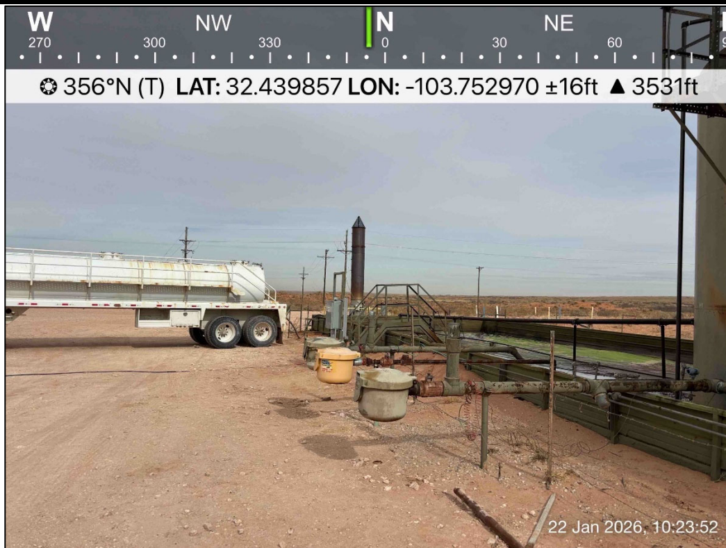
PHOTO 4: Northern view during initial pressure washing activities. 1/22/2026
