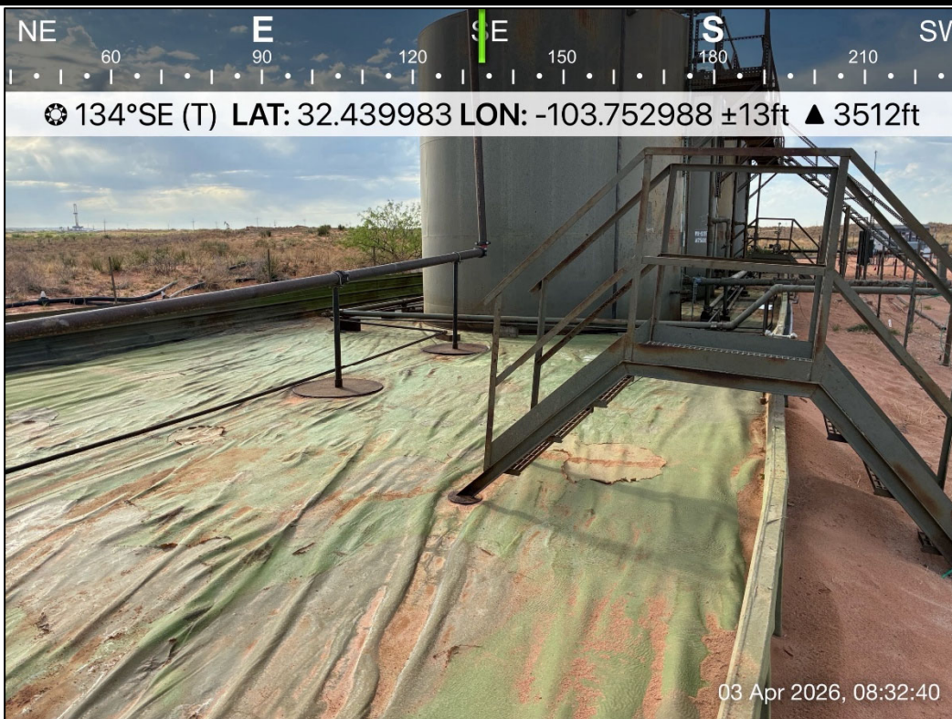
PHOTO 12: Southeastern view during liner inspection activities. 4/3/2026
