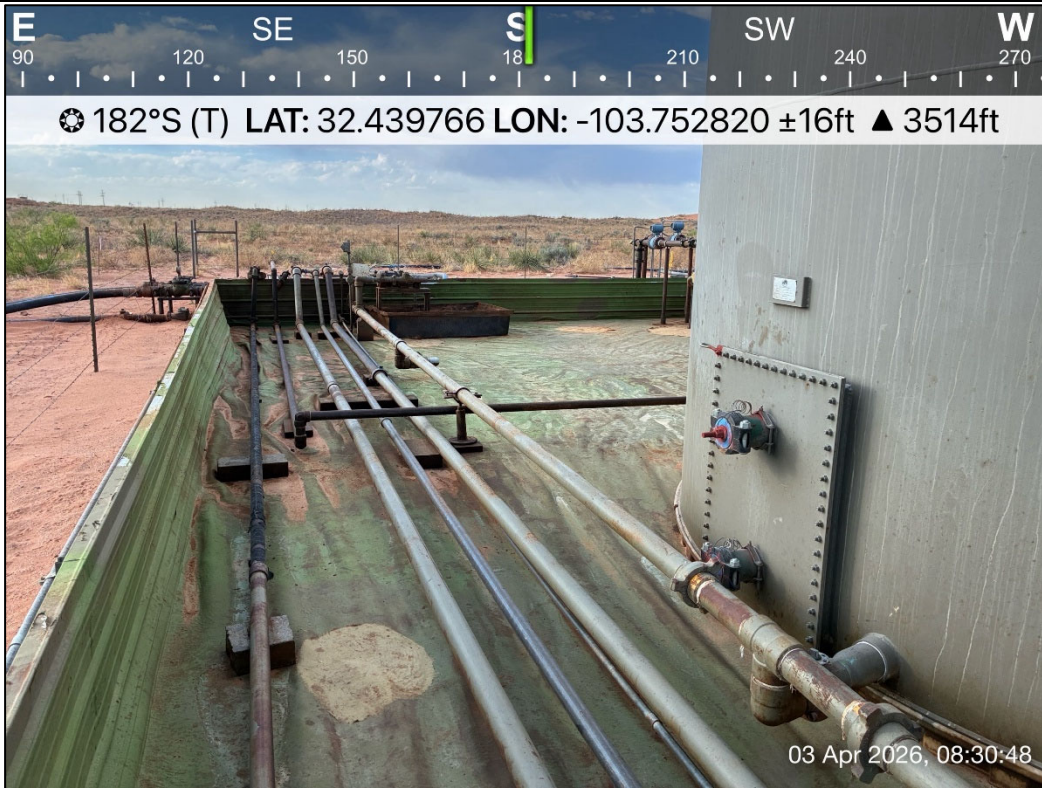
PHOTO 15: Southern view during liner inspection activities. 4/3/2026
