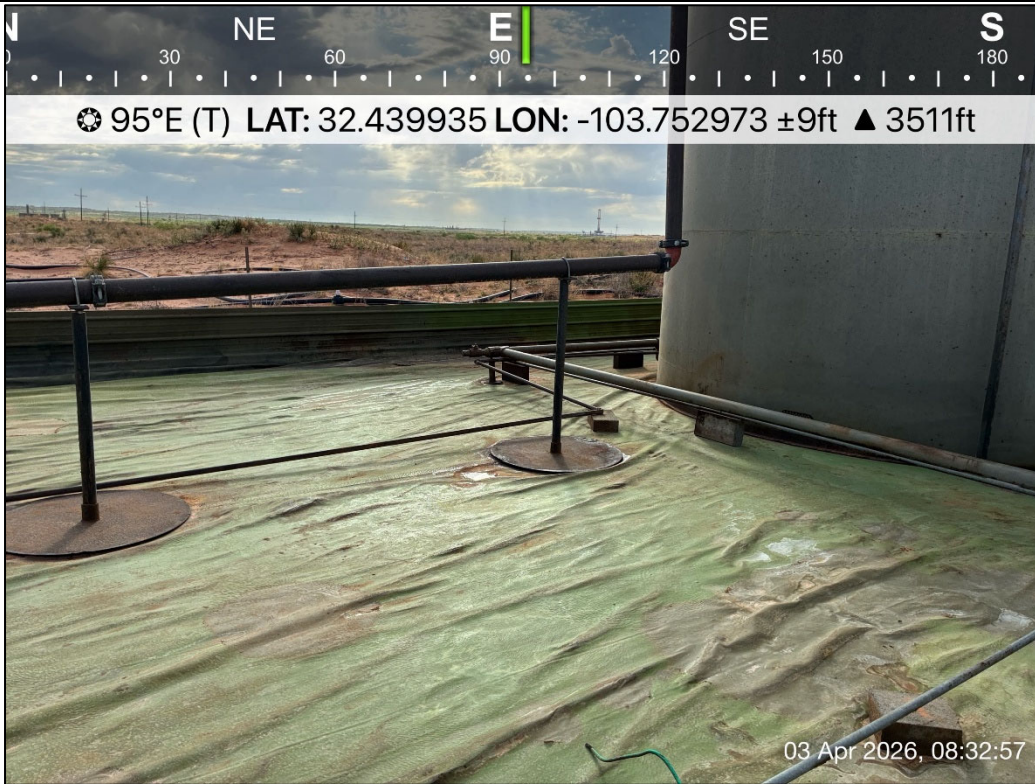
PHOTO 13: Eastern view during liner inspection activities. 4/3/2026
