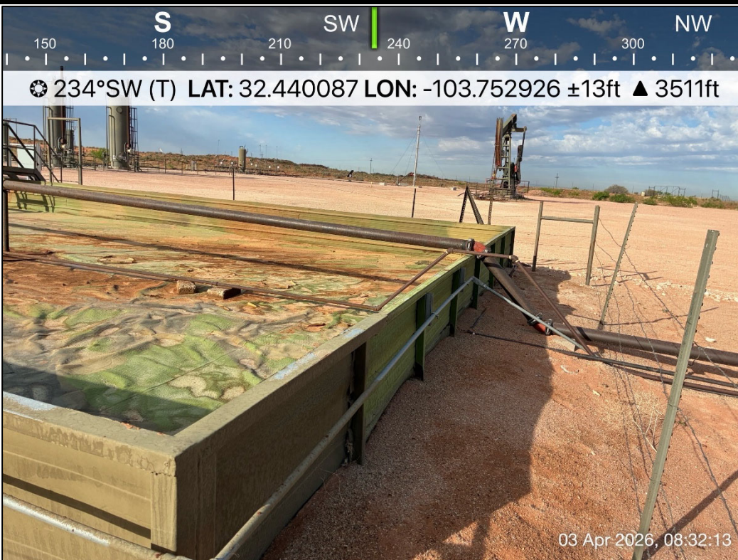
PHOTO 10: Southwestern view outside of containment during liner inspection activities. 4/3/2026
