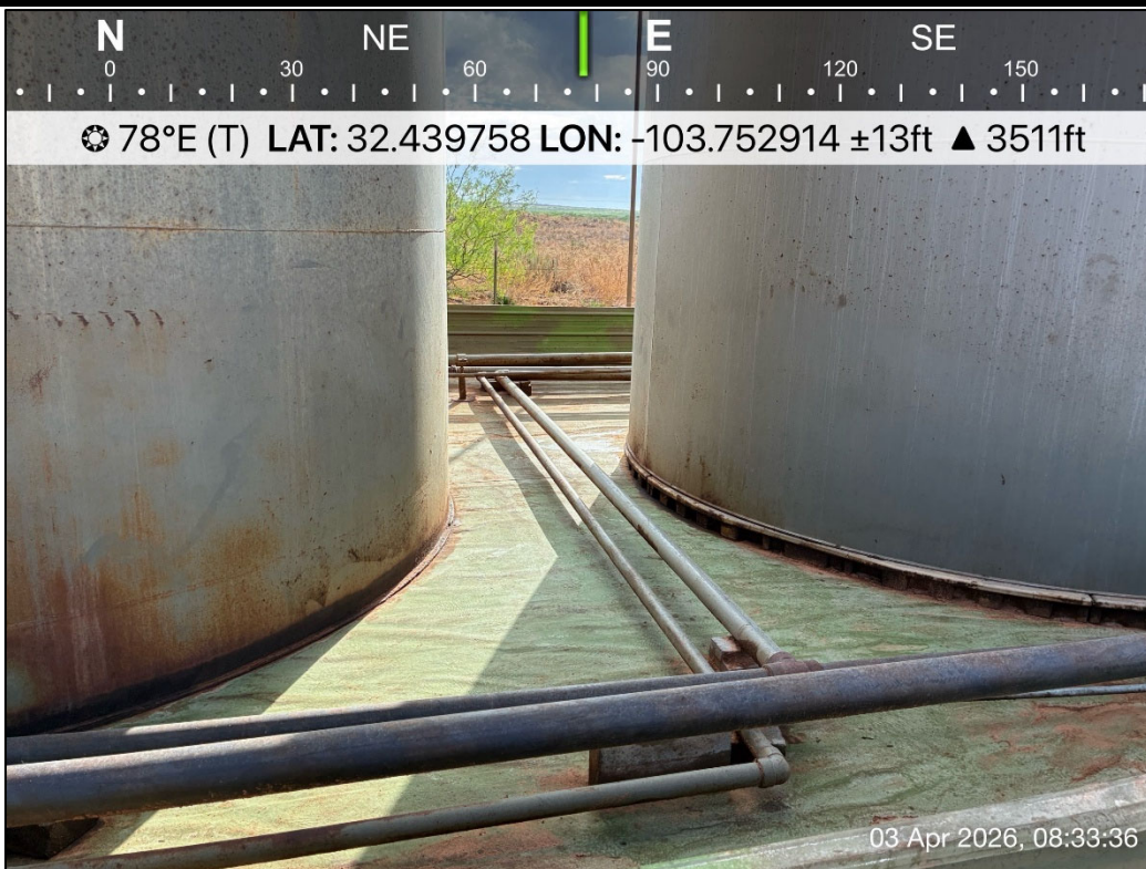
PHOTO 14: Eastern view during liner inspection activities. 4/3/2026
