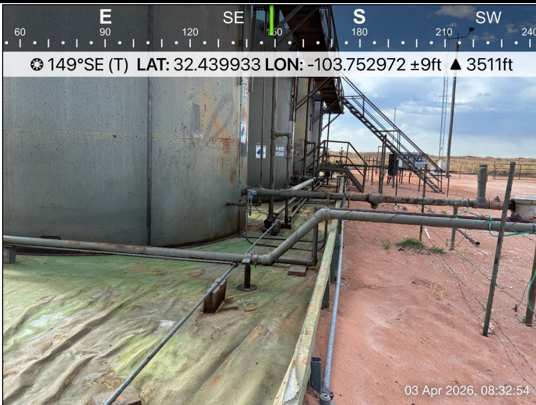
PHOTO 16: Southeastern view during liner inspection activities. 4/3/2026
