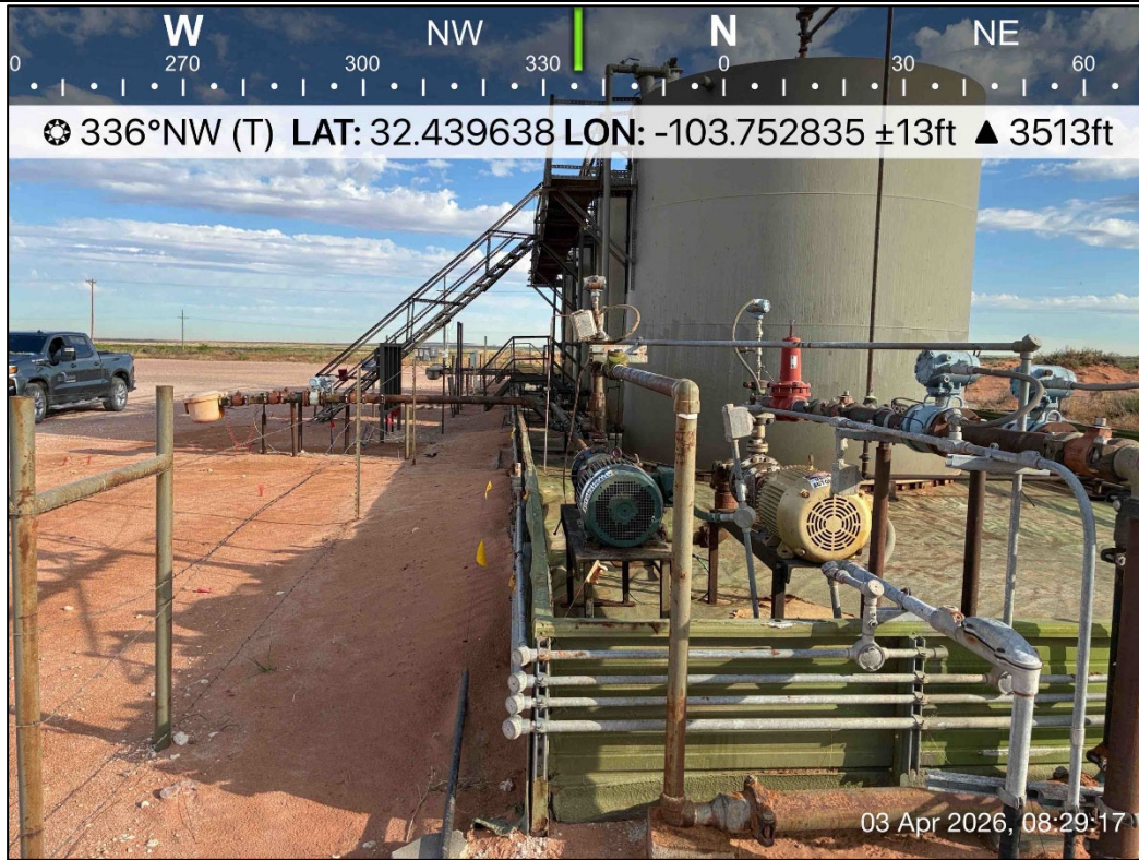
PHOTO 7: Northwestern view outside of containment during liner inspection activities. 4/3/2026
