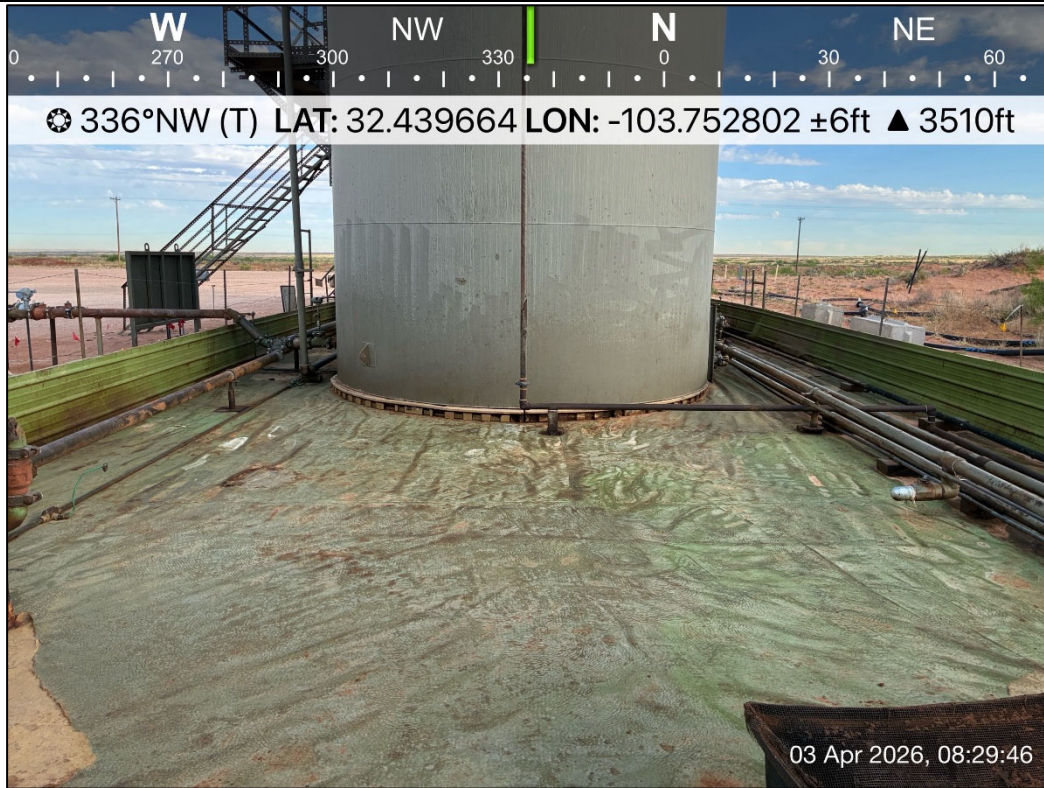
PHOTO 17: Northwestern view during liner inspection activities. 4/3/2026
