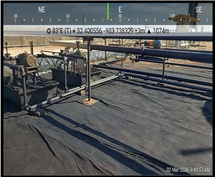
View of Secondary Containment
