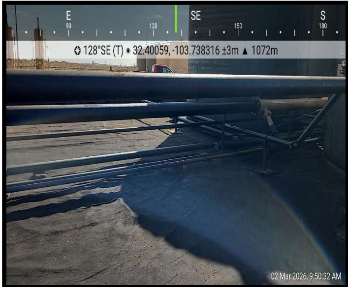
View of Secondary Containment
