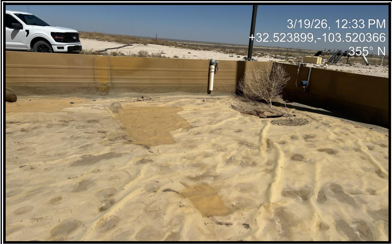
View of the site following the liner repair.
