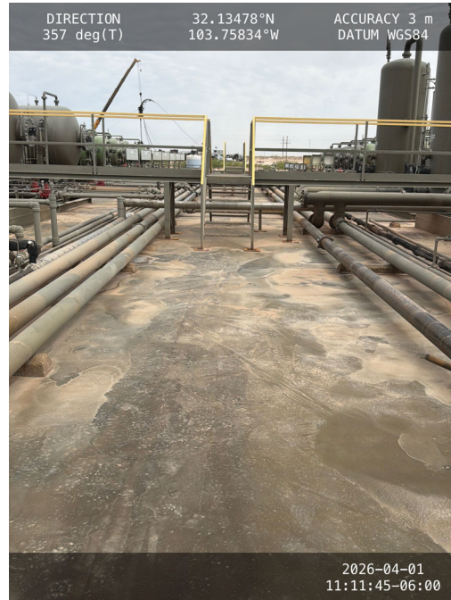
Photo 10 Photo of containment towards north.
