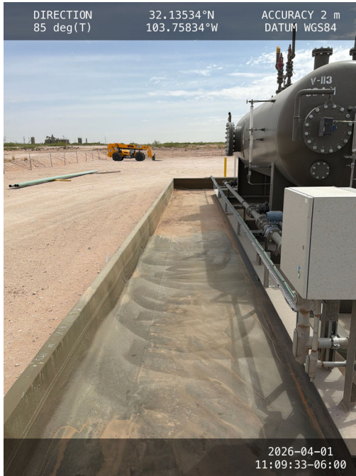
Photo 9 Photo of containment towards east.
