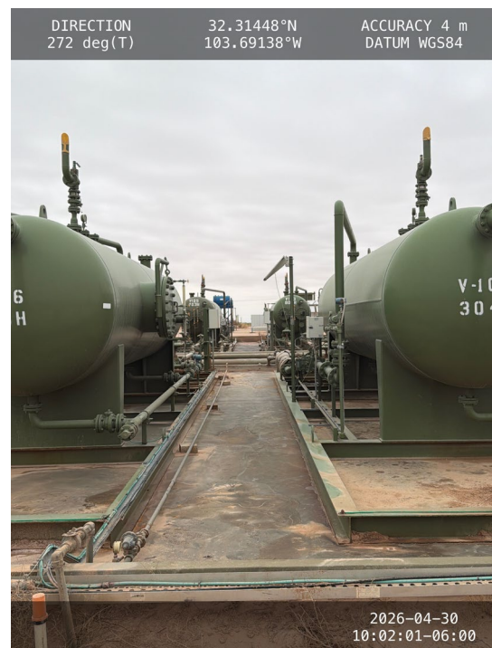
Photo 12 View of the central area of the secondary containment towards west.
