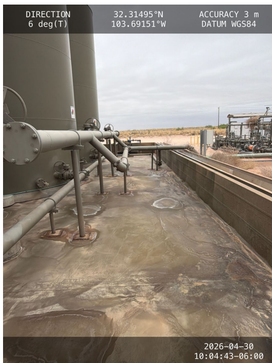
Photo 11 View of containment towards north.
