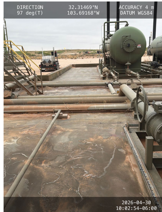
Photo 8 View of containment towards east.
