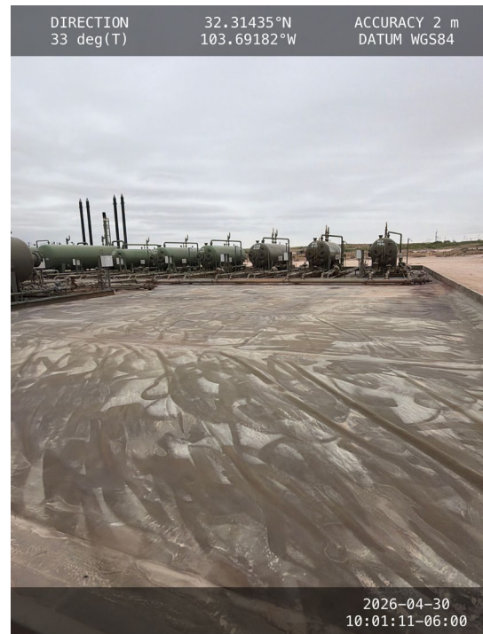
Photo 2 View of north-northeast side of containment.
