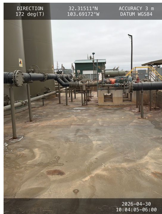
Photo 4 View of containment towards south.
