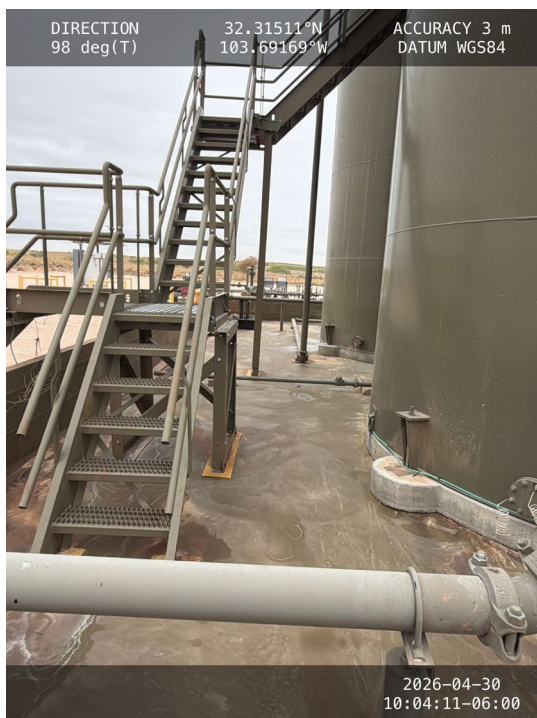
Photo 3 View of containment towards east.
