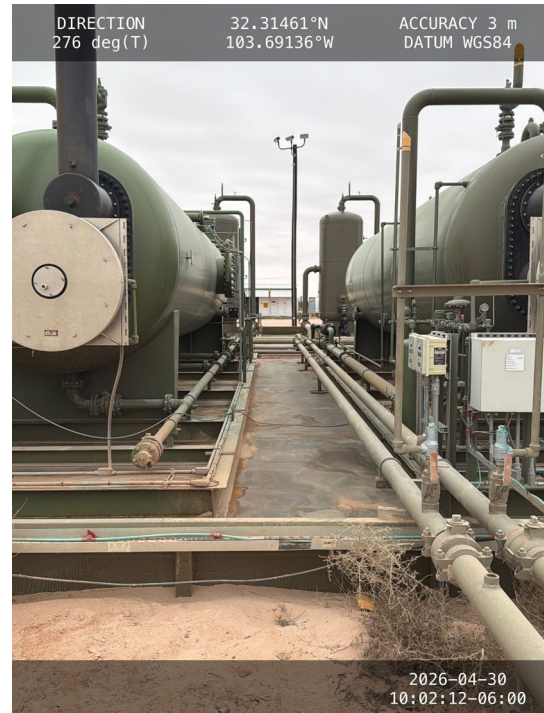
Photo 13 View of the secondary containment towards west.
