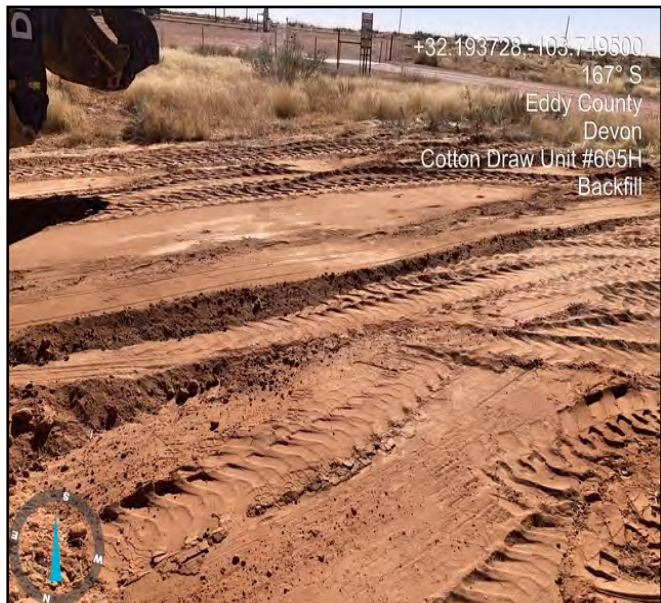
Photo taken post backfill.
