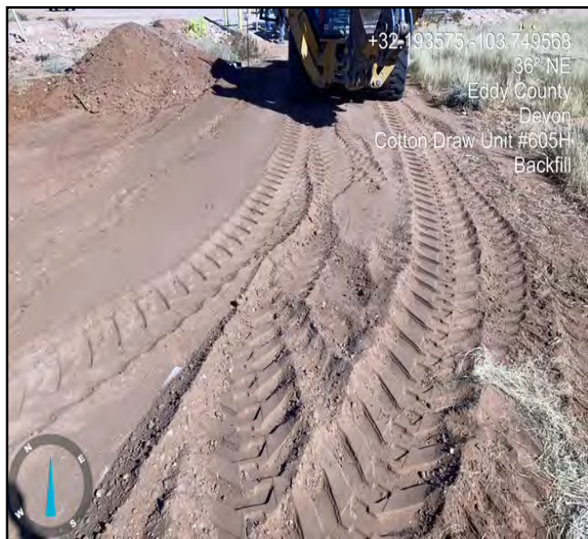
Photo taken post backfill.
