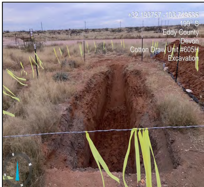
Photo taken during excavation process facing south.
