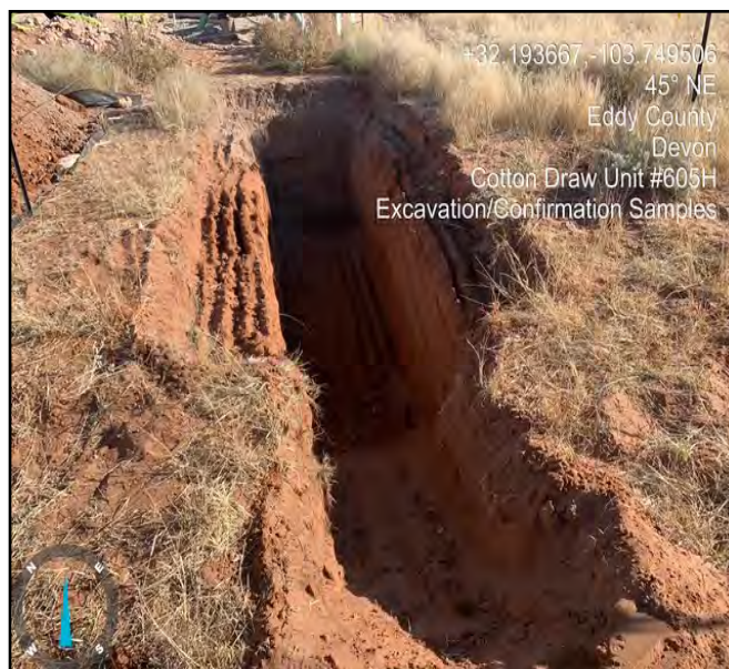
Photo taken during excavation process facing northeast.
