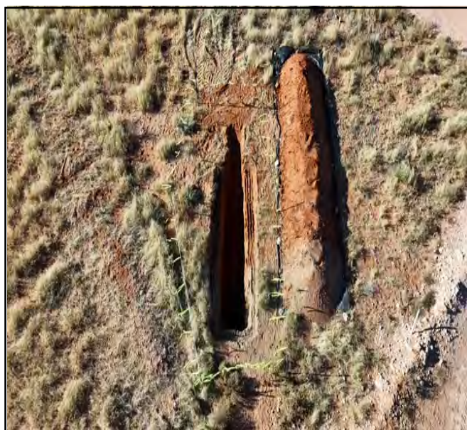
Photo taken during excavation process.
