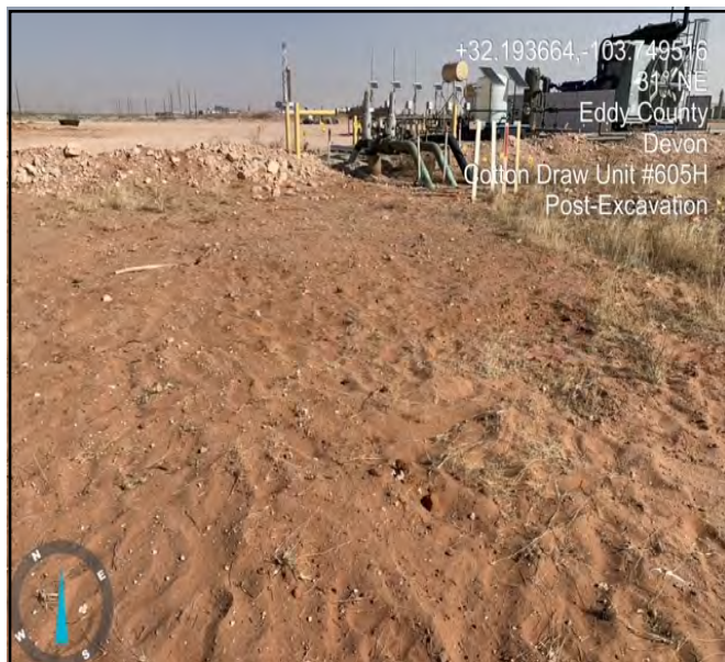
Photo taken post backfill.
