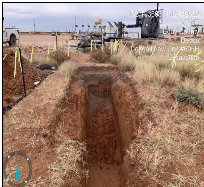
Photo taken during excavation process facing northeast.
