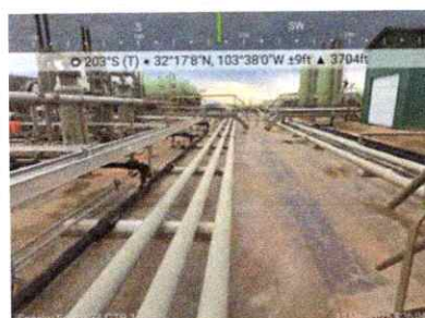
Secondary containment — berm top, south view
