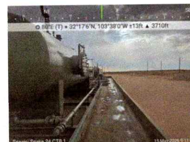
Secondary containment — east berm, long view 09:11:05 80°E 32°17'6"N 103°38'0"W
