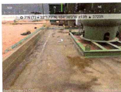
Secondary containment — berm walkway, north view 08:38:22 7°N 32°17'7"N 103°38'0"W
