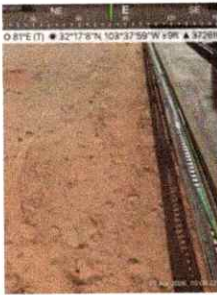
Exterior perimeter — east side, berm base at ground level
