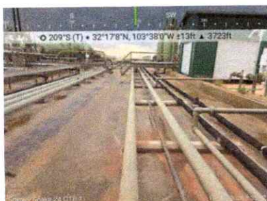
Secondary containment — berm top, SSW view
