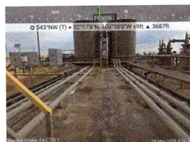
Secondary containment — berm top, NW view toward storage tanks
