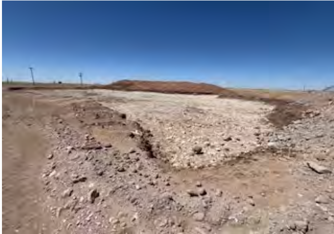
View to NW of excavation (4/28/26).
