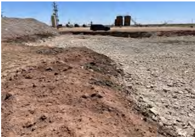
View to S of E end of excavation (4/28/26).
