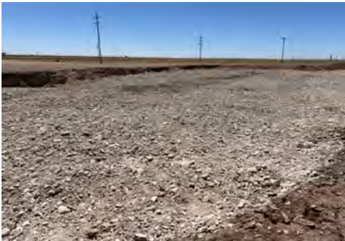
View to SW of excavation (4/28/26).
