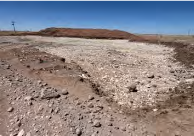
View to NW of excavation (4/28/26).
