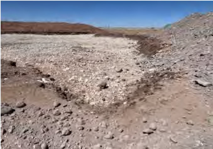
View to N of E end of excavation (4/28/26).
