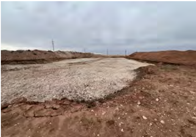
View to NE of excavation (11/19/25).
