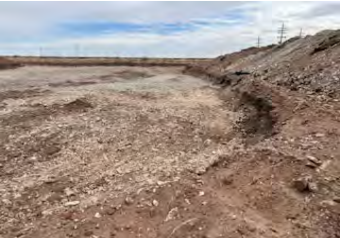
View to W of N side of excavation (11/19/25).
