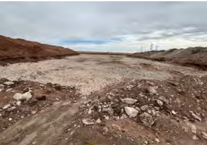
View to W of excavation (11/19/25) with clean Stockpile to N and impacted stockpile to S.
