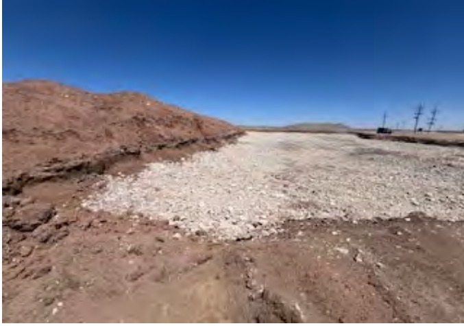
View to E of N wall of excavation and clean stockpile to N (4/28/26).
