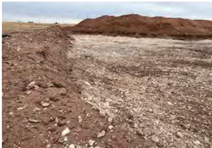
View to N at W end of excavation (11/19/25).
