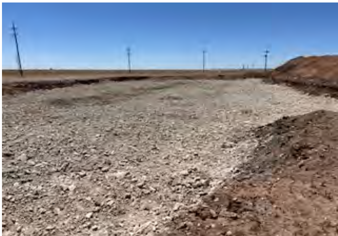
View to W of excavation (4/28/26).
