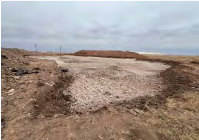
View to SE of excavation (11/19/25).
