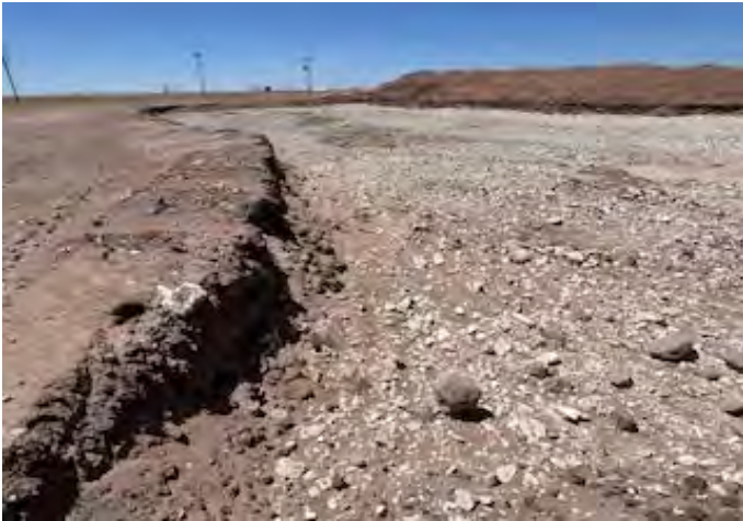
View to NW of S wall of excavation (4/28/26).
