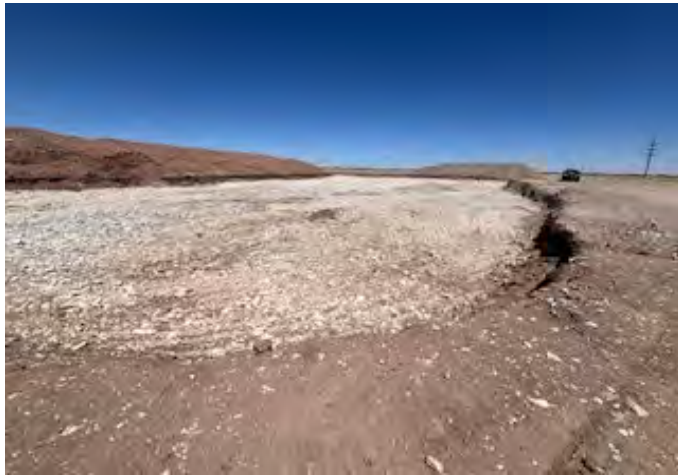
View to E of S wall of excavation (4/28/26).
