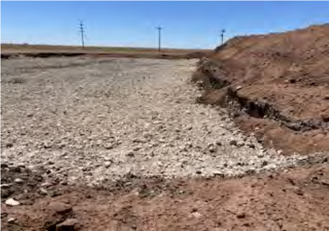
View to SW of excavation (4/28/26) with clean stockpile to N.
