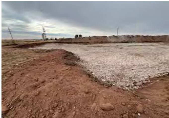
View to N of excavation (11/19/25).
