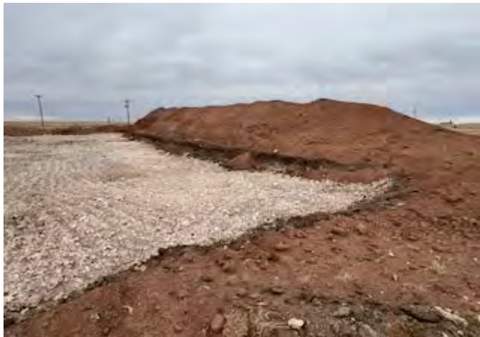
View to NW of excavation with stockpile to N (11/19/25).
