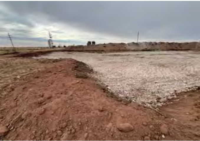
View to NW of excavation (11/19/25).
