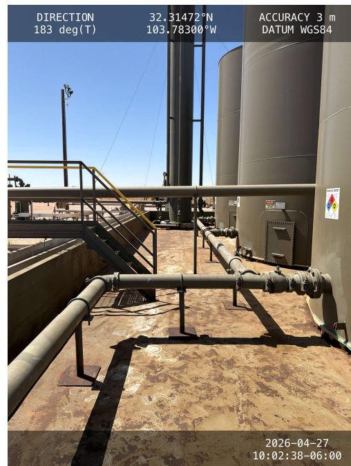
Photo 8 View of containment towards south.
