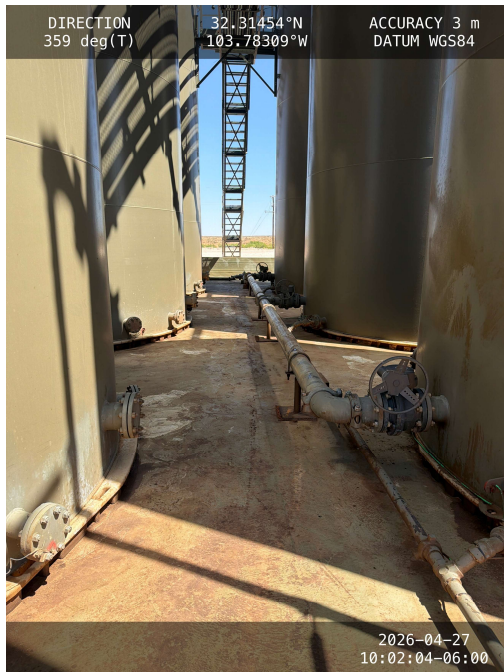
Photo 5 View of containment towards north.
