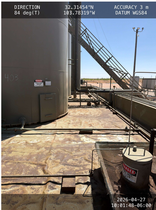
Photo 3 View of containment towards east.
