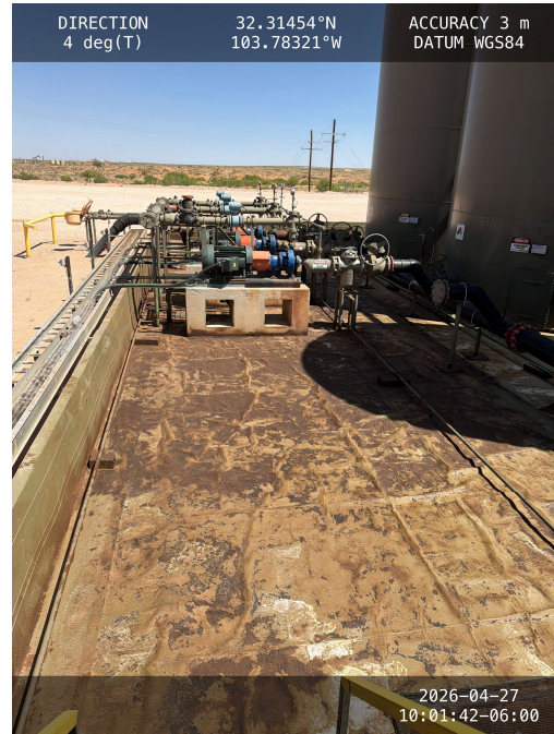
Photo 2 View of containment towards north.
