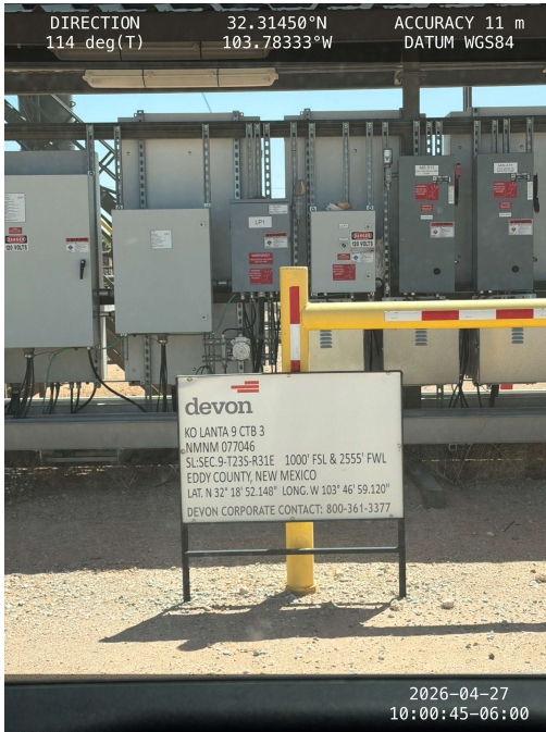
Photo 1 View of facility sign.
