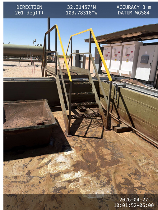
Photo 4 View of southwest corner of containment.
