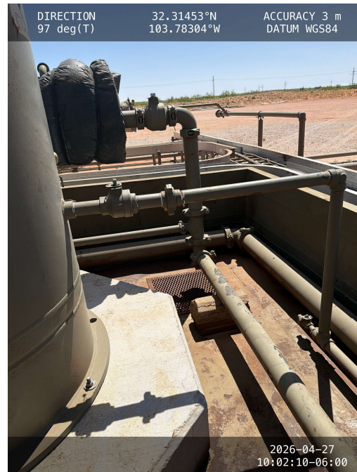
Photo 6 View of southeast corner of containment.
