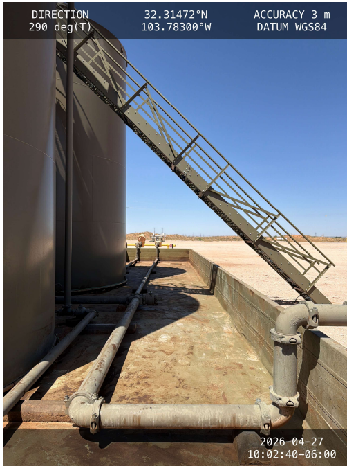
Photo 9 View of containment towards west.
