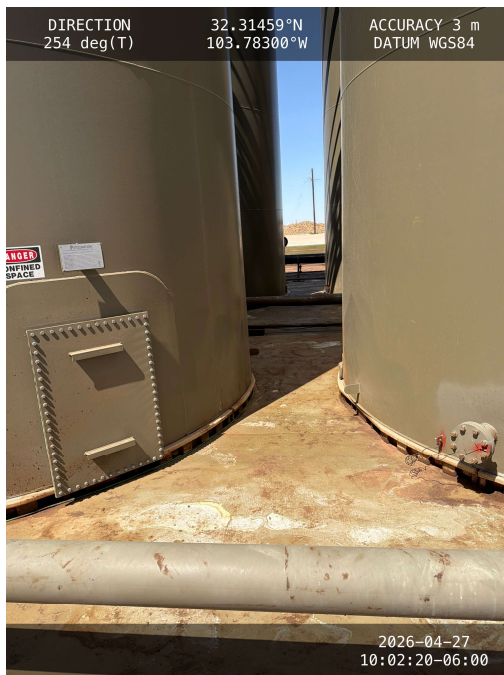
Photo 7 View of containment towards west.
