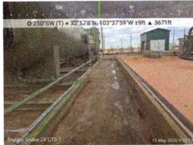
#44 Secondary containment — west berm edge, SW view
