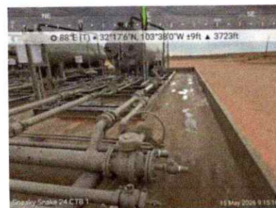
#40 Secondary containment — east berm edge, ball valve 09:15:16 88°E 32°17'6"N 103°38'0"W
