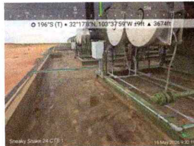
#45 Secondary containment — south berm edge, compressor skid
