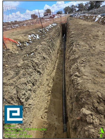
Photograph: 2 Date: 2/26/2026 Description: MPLX LP pipeline trench. Observe the narrow width of trench. View: East
