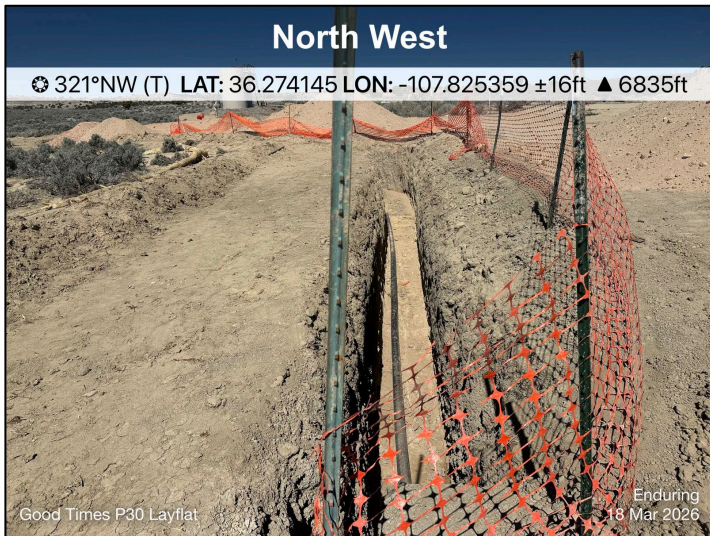
Photograph: 3 Date: 3/6/2026 Description: MPLX LP pipeline trench. The pipeline across the floor limits the effectiveness of a backhoe. View: Northwest
