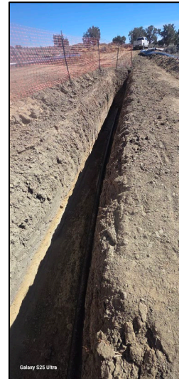
Photograph: 2 Date: 2/26/2026 Description: MPLX pipeline trench View: East
