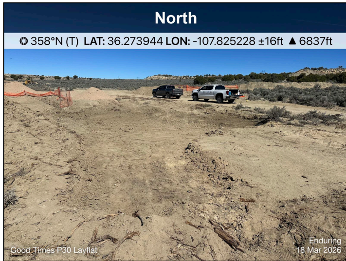
Photograph: 5 Date: 3/18/2026 Description: Final excavation extent. Observe the shallow and non-distinct sidewalls. View: North
