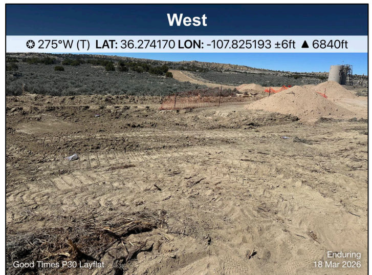
Photograph: 6 Date: 3/18/2026 Description: Final excavation extent. Observe the shallow and non-distinct sidewalls. View: West
