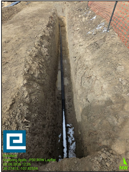
Photograph: 1 Date: 3/6/2026 Description: View of the MPLX LP pipeline trench. The pipeline across the floor limits the effectiveness of a backhoe. View: Northwest
