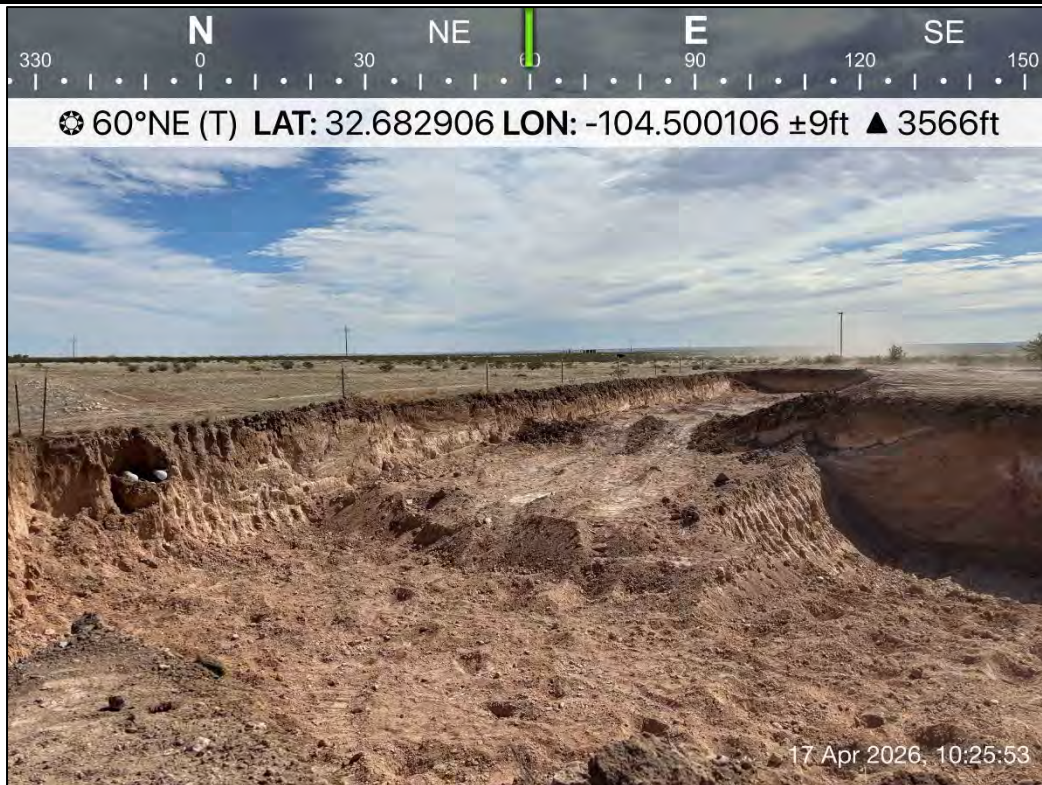
PHOTO 18: Northeastern view of excavation extent. 4/17/2026
