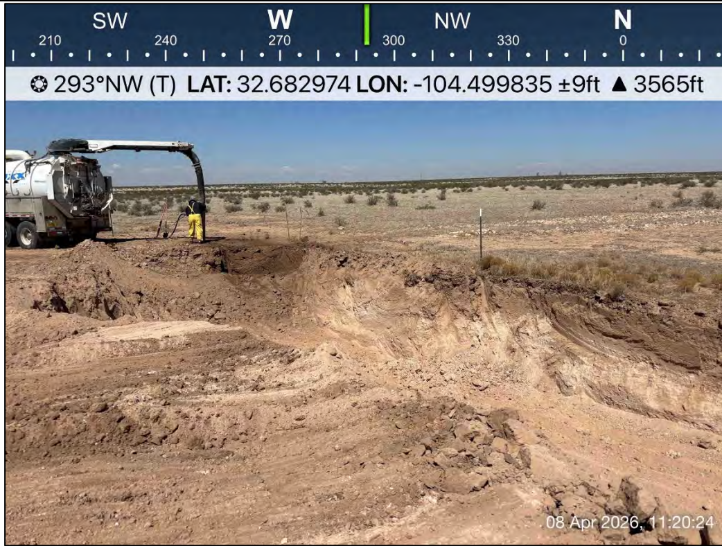
PHOTO 7: Northwestern view during excavation activities. 4/8/2026
