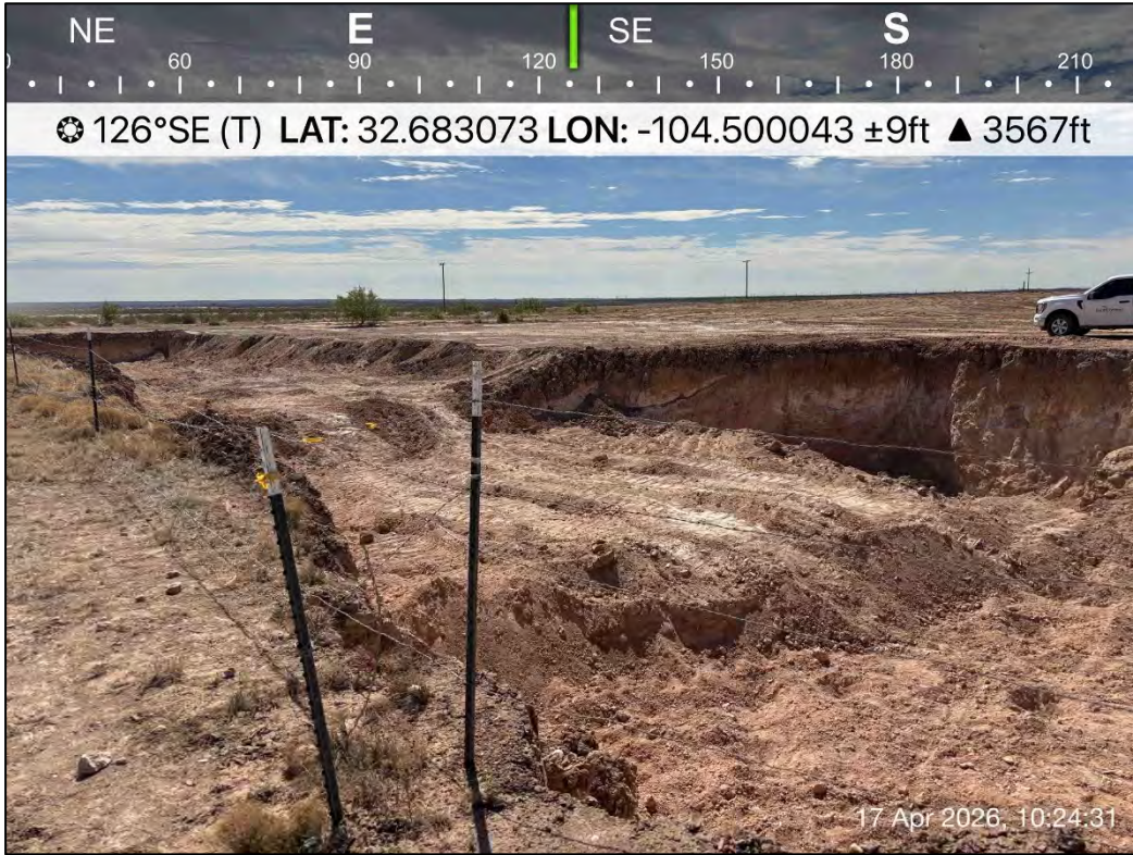
PHOTO 17: Southeastern view of excavation extent. 4/17/2026
