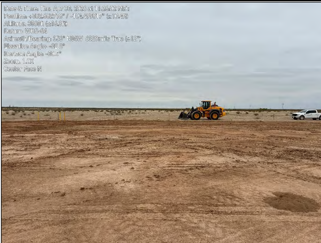
PHOTO 24: Northwestern view following restoration activities. 4/30/2026
