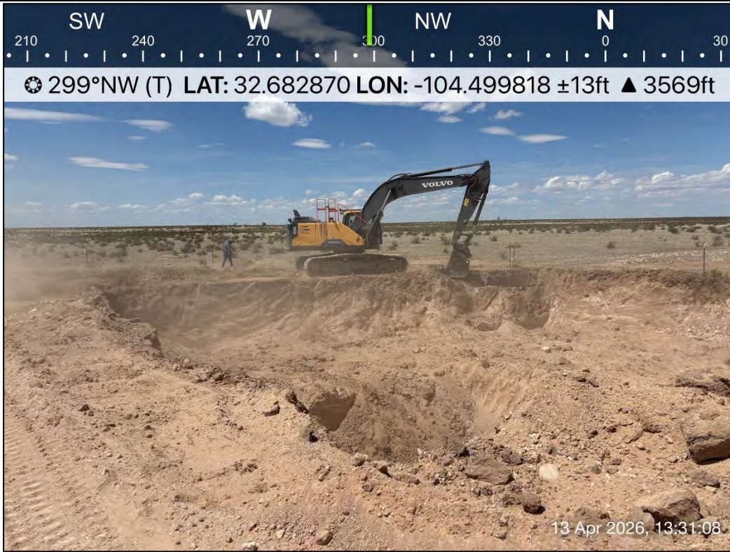
PHOTO 13: Northwestern view during excavation activities. 4/13/2026
