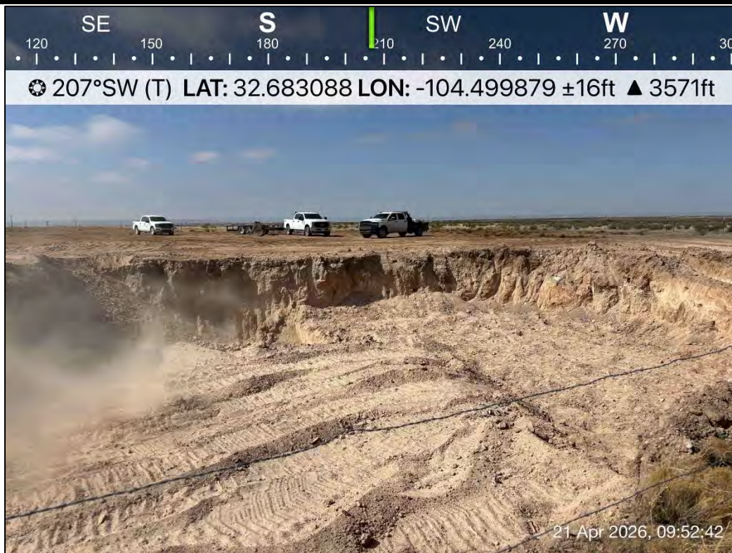
PHOTO 20: Southwestern view during restoration activities. 4/21/2026
