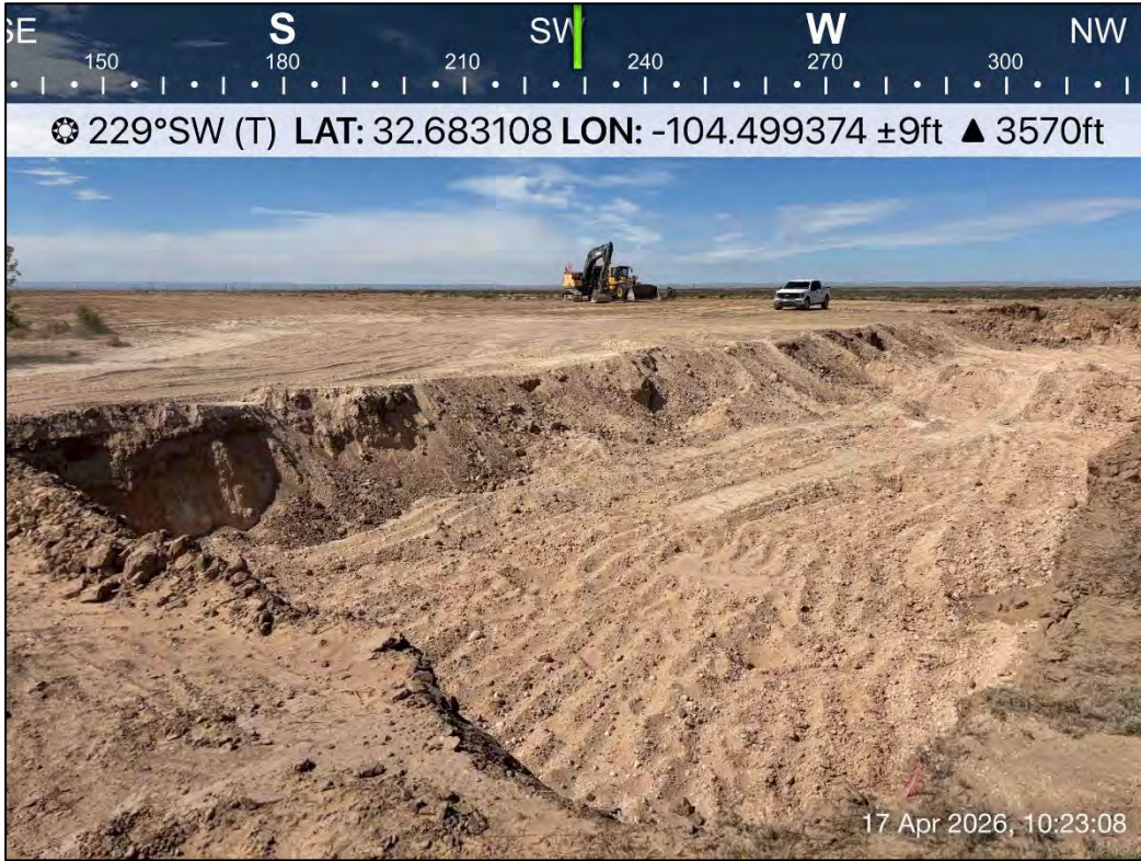
PHOTO 15: Southwestern view of excavation extent. 4/17/2026
