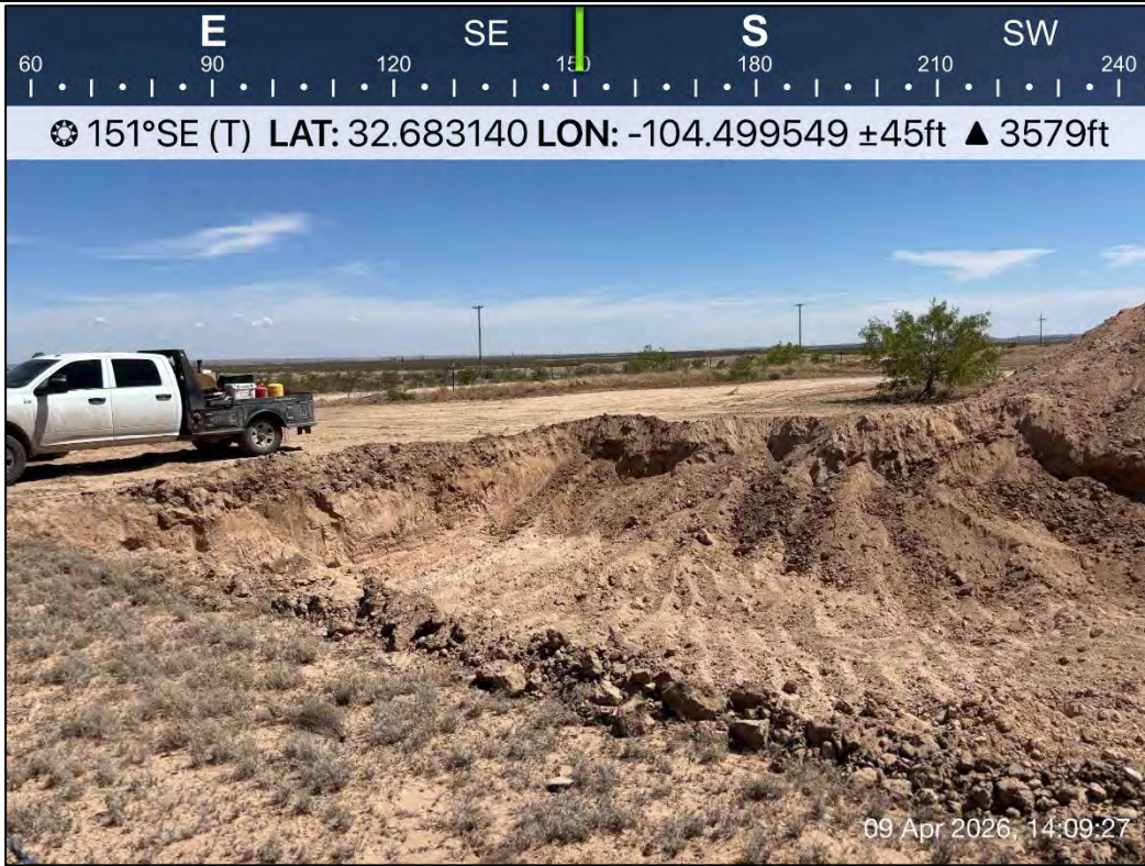
PHOTO 9: Southeastern view during excavation activities. 4/9/2026
