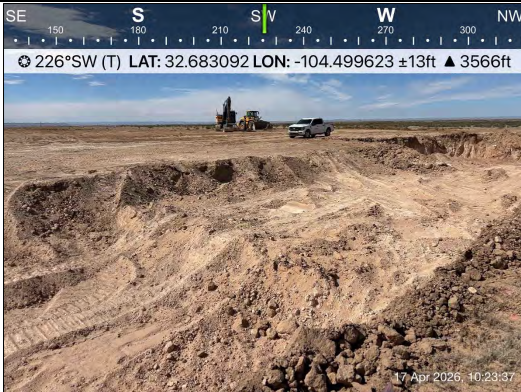
PHOTO 16: Southwestern view of excavation extent. 4/17/2026
