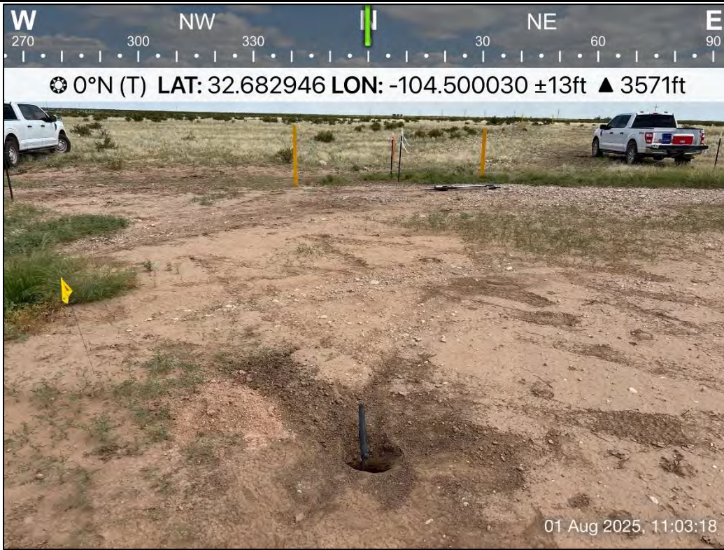
PHOTO 5: Northern view during initial delineation activities. 8/01/2025
