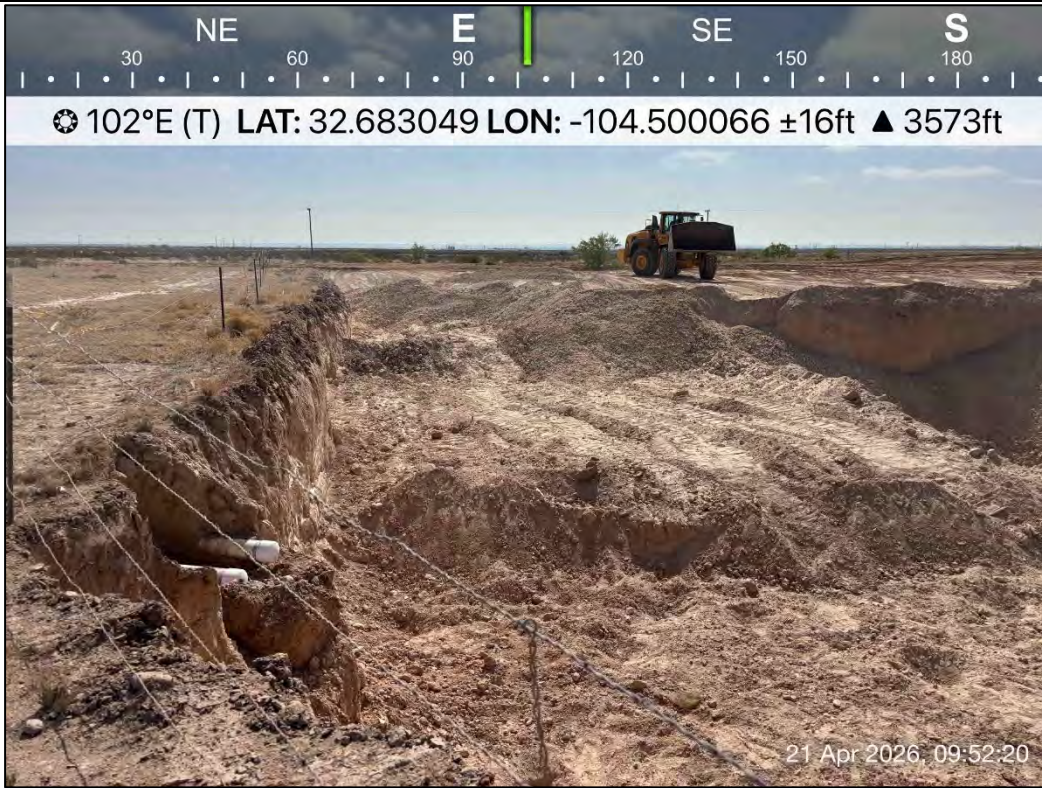
PHOTO 19: Southeastern view during restoration activities. 4/21/2026
