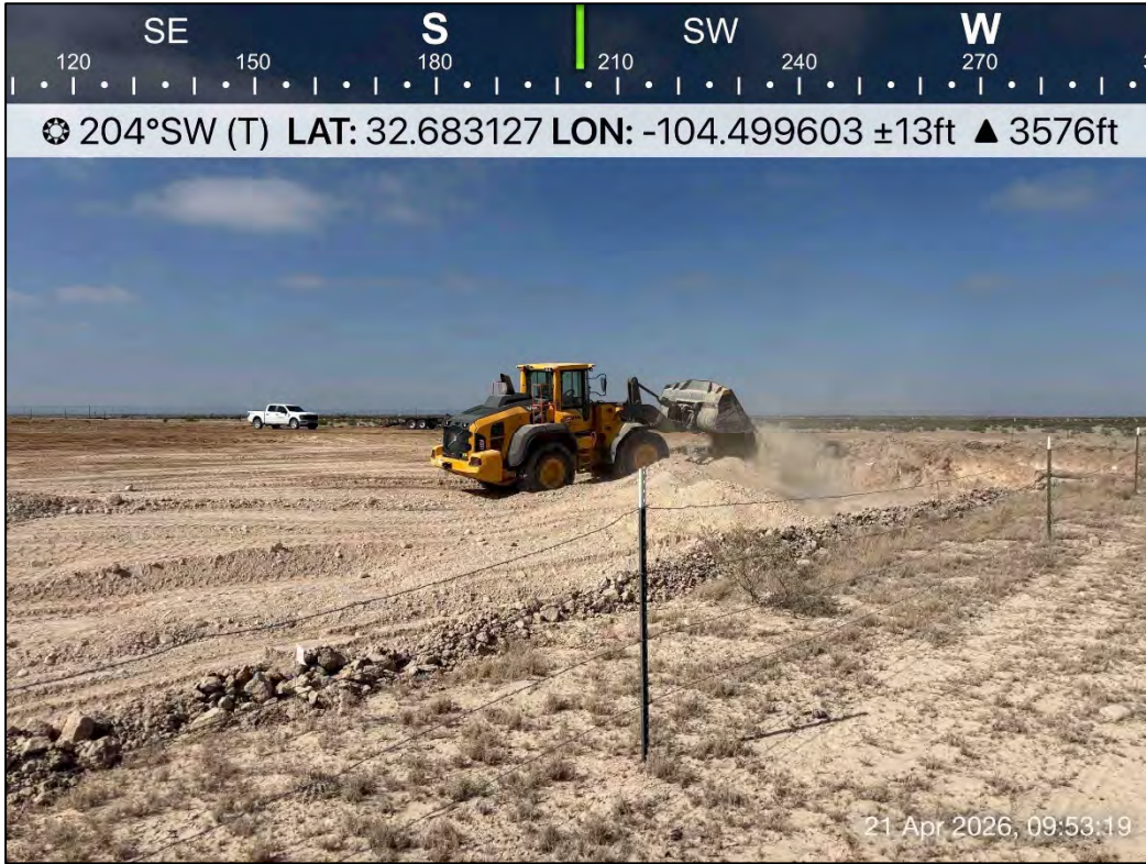
PHOTO 21: Southwestern view during restoration activities. 4/21/2026
