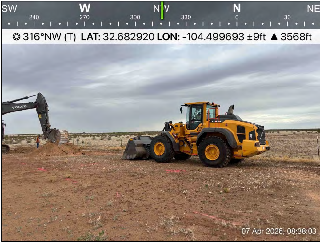
PHOTO 3: Northwestern view during excavation activities. 4/7/2026
