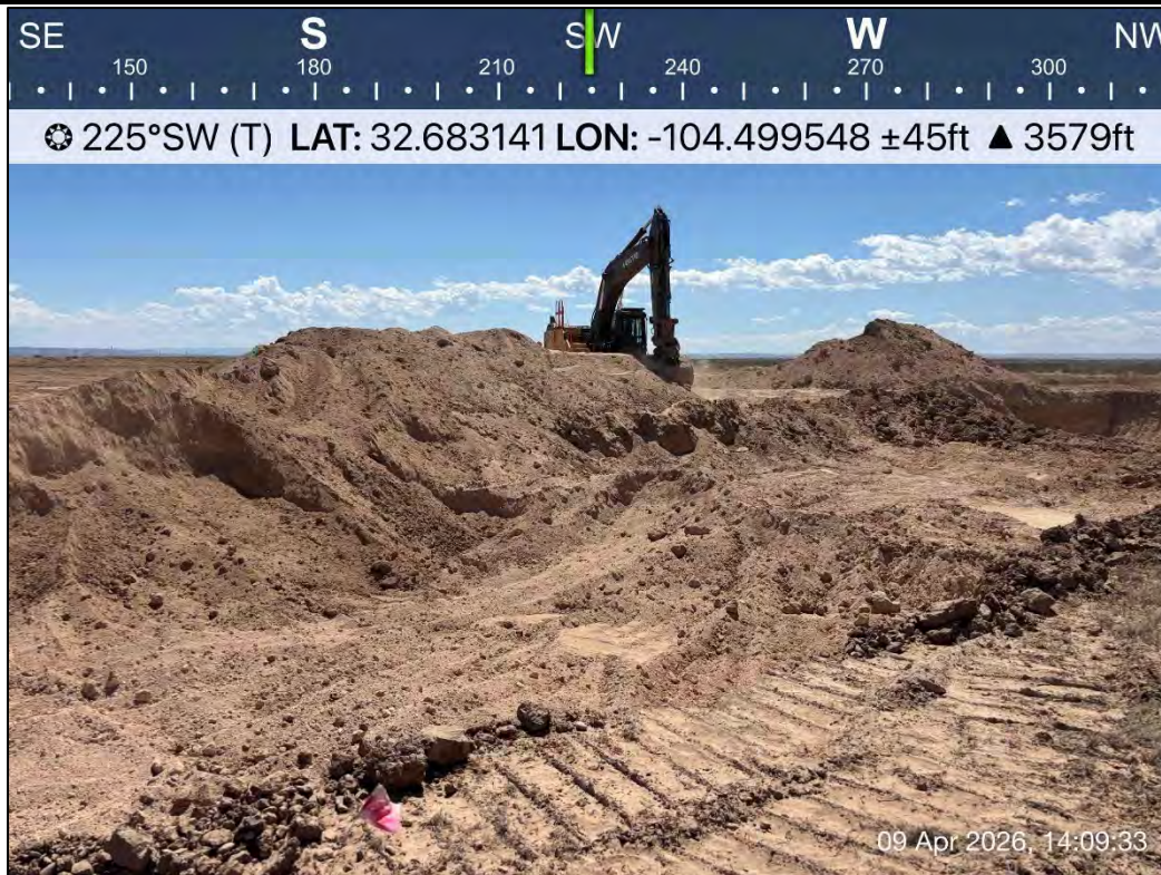
PHOTO 10: Southwestern view during excavation activities. 4/9/2026
