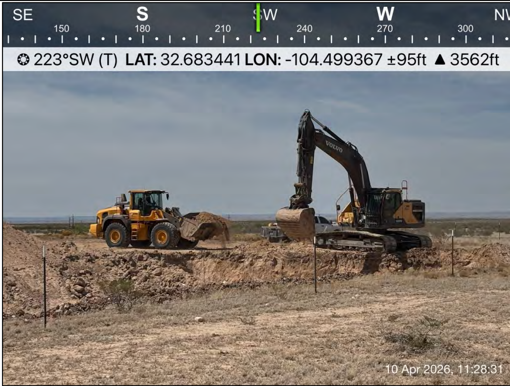
PHOTO 11: Southwestern view during excavation activities. 4/10/2026
