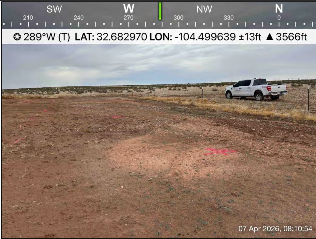
PHOTO 1: Northwestern view during preparation for excavation activities. 4/7/2026
