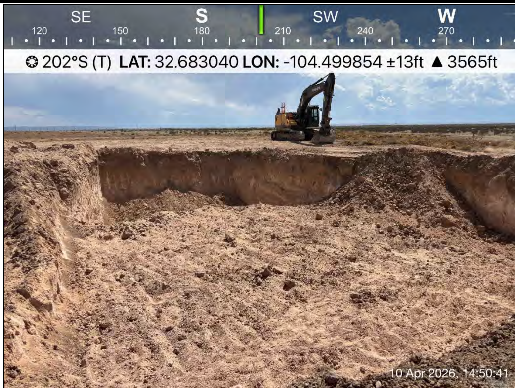
PHOTO 12: Southwestern view during excavation activities. 4/10/2026
