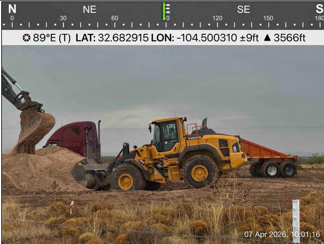
PHOTO 4: Eastern view during excavation activities. 4/7/2026
