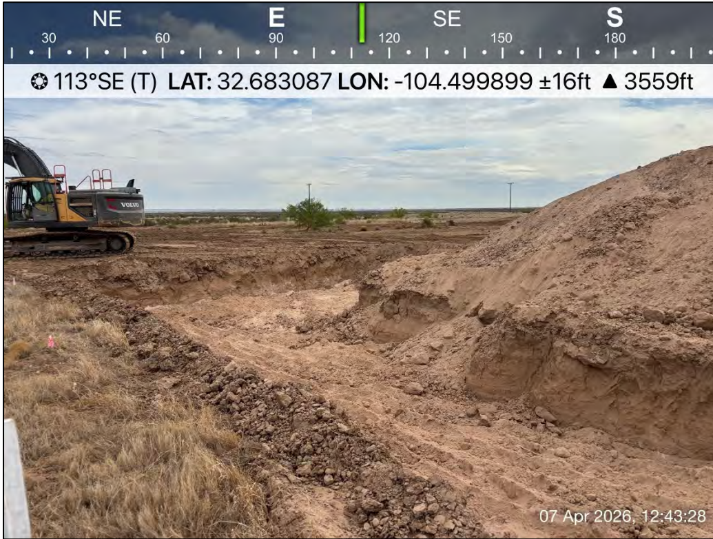
PHOTO 5: Southeastern view during excavation activities. 4/7/2026
