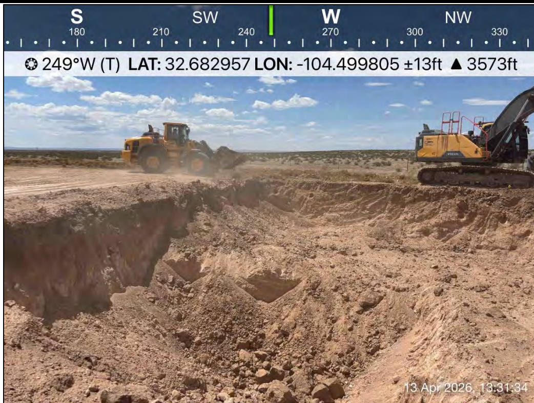
PHOTO 14: Southwestern view during excavation activities. 4/13/2026
