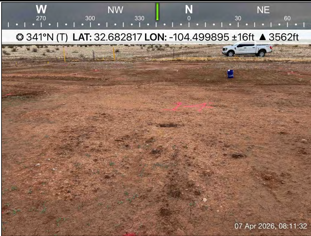
PHOTO 2: Northwestern view during preparation for excavation activities. 4/7/2026
