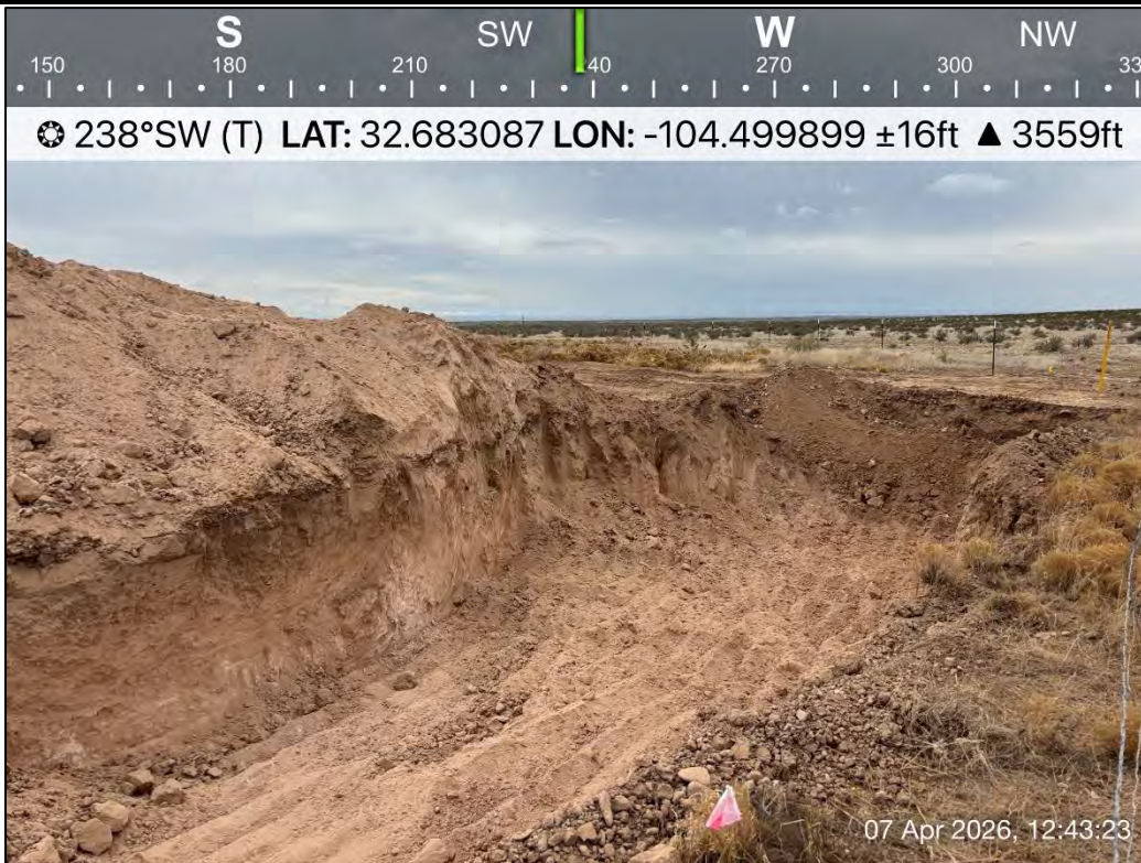
PHOTO 6: Southwestern view during excavation activities. 4/7/2026
