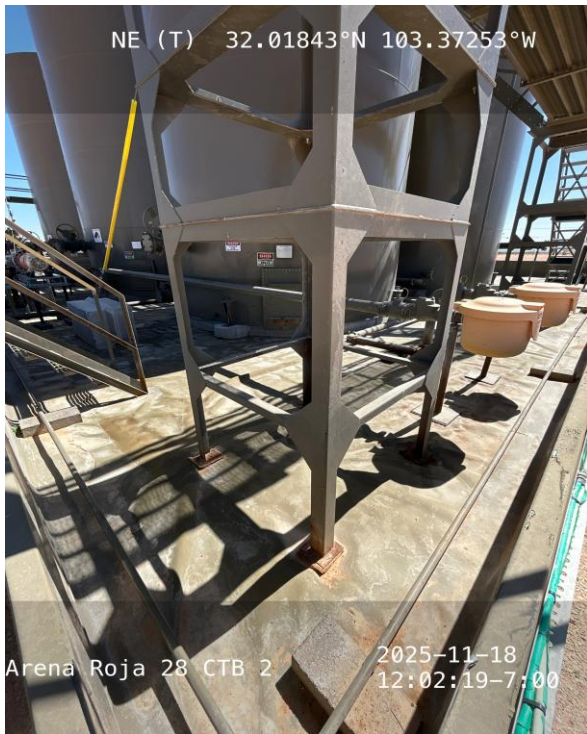
Photo 5 View of southwest corner of secondary containment.
