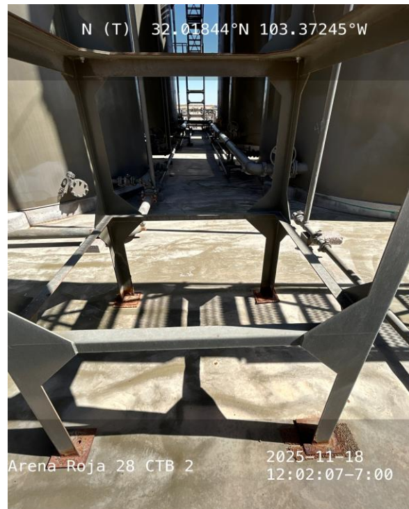
Photo 4 View of central portion of secondary containment towards north.
