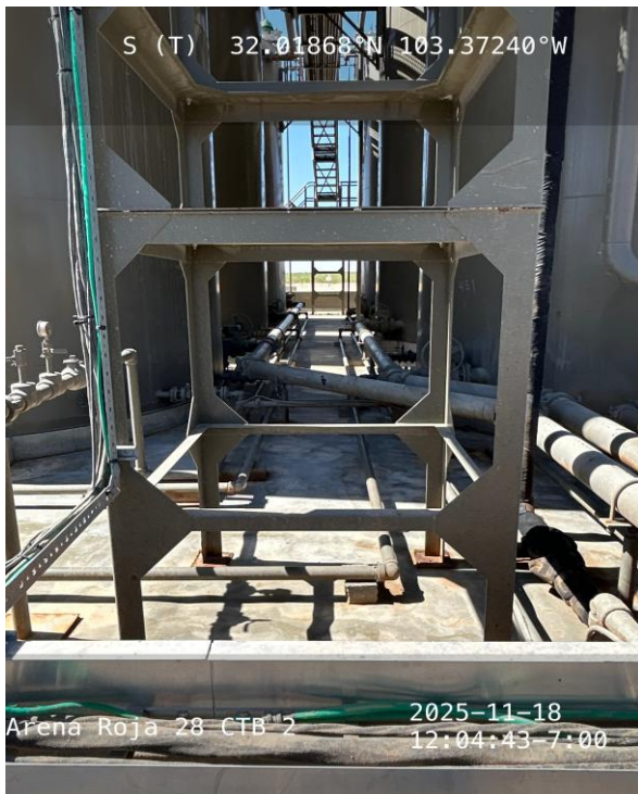
Photo 7 View of central portion of secondary containment towards south.
