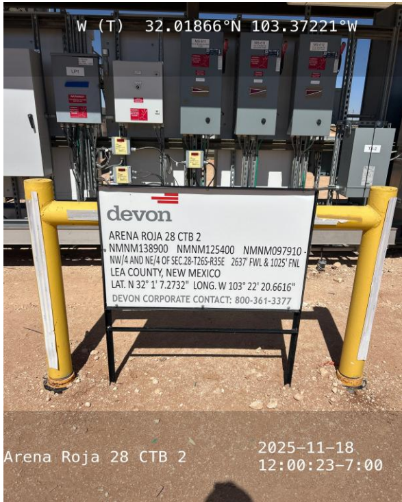
Photo 1 View of facility sign.
