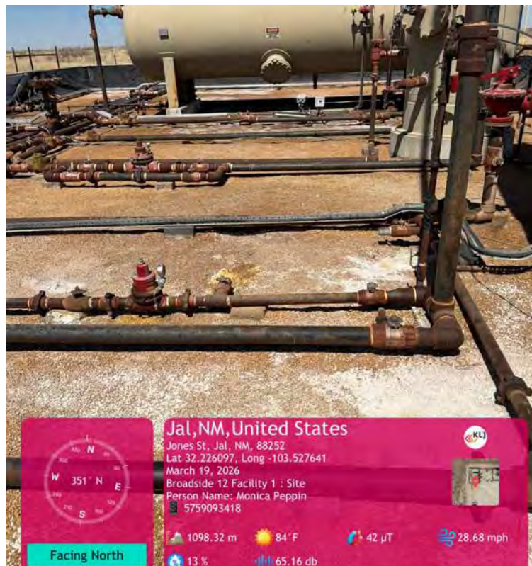
Middle area of containment.
