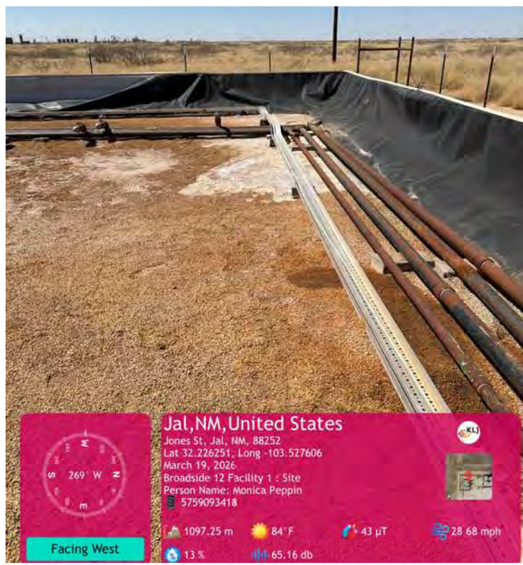
North wall area.
