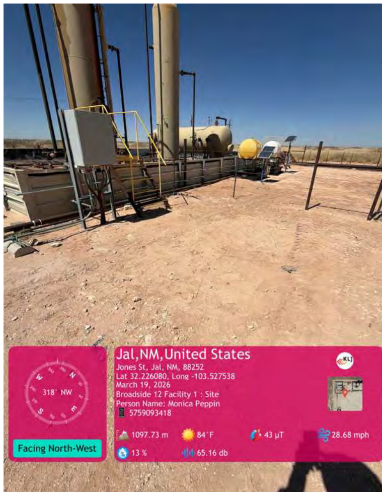
East wall of containment.
