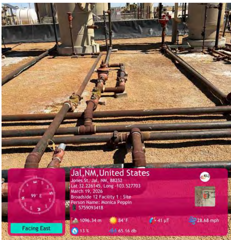
Gravel under piping.
