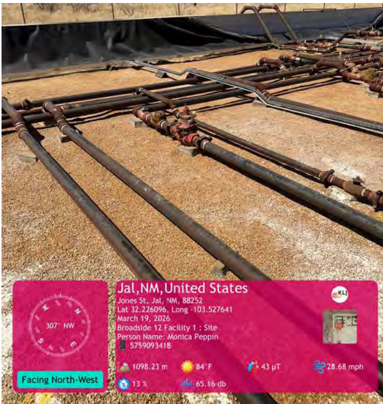
Gravel under piping.
