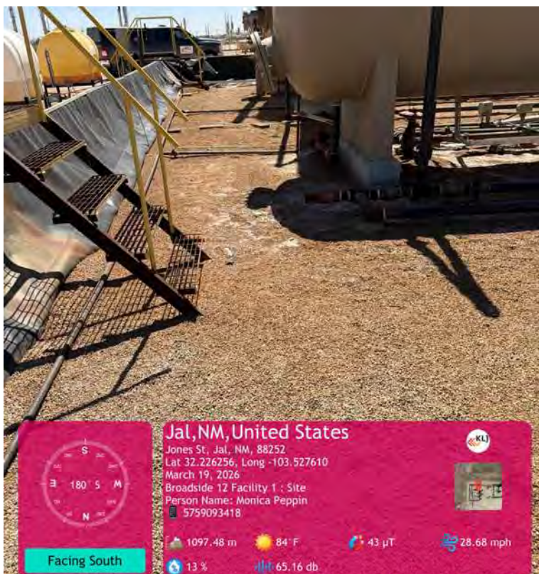
East wall area.
