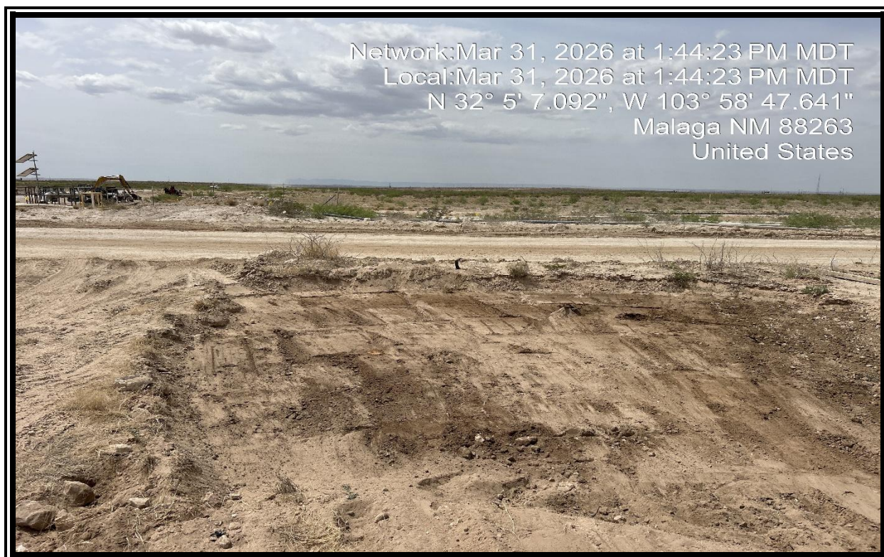
View of the site during excavation activities.
