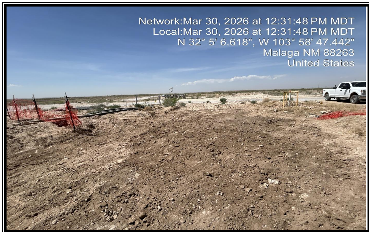
View of the site during excavation activities.
