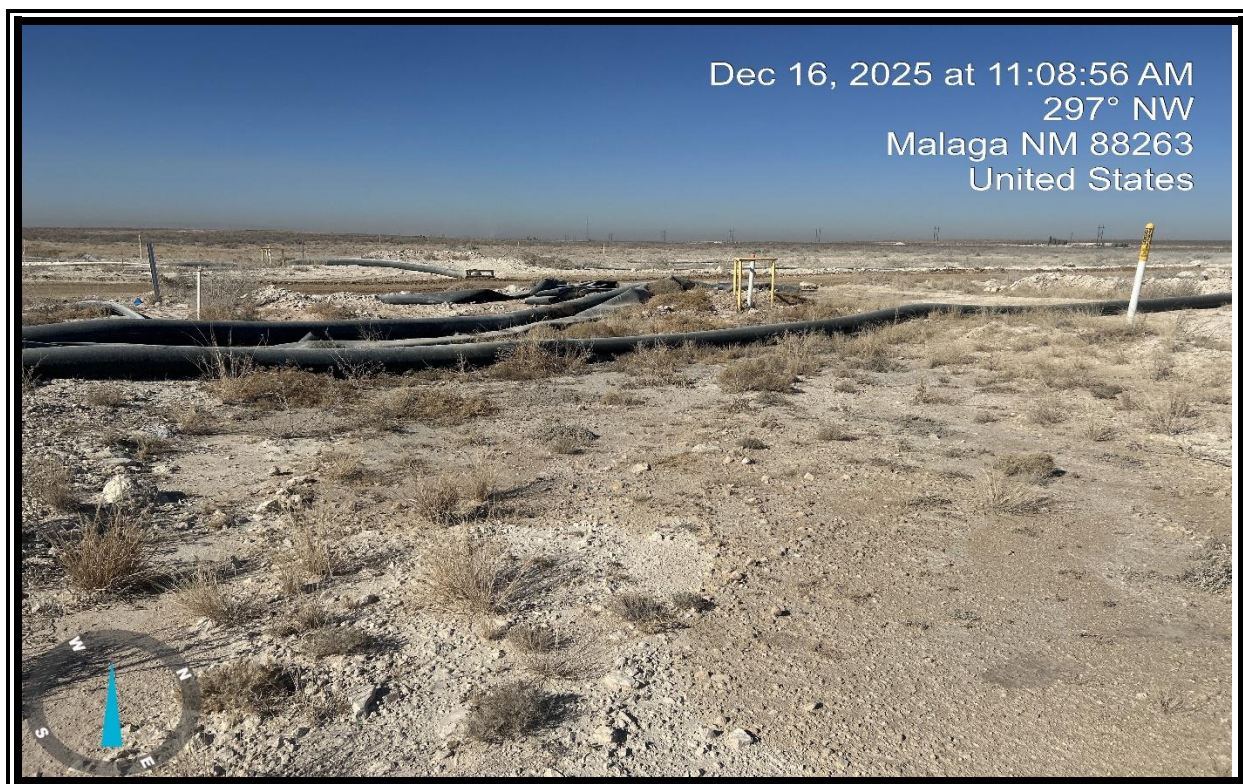
View of the site during assessment activities.
