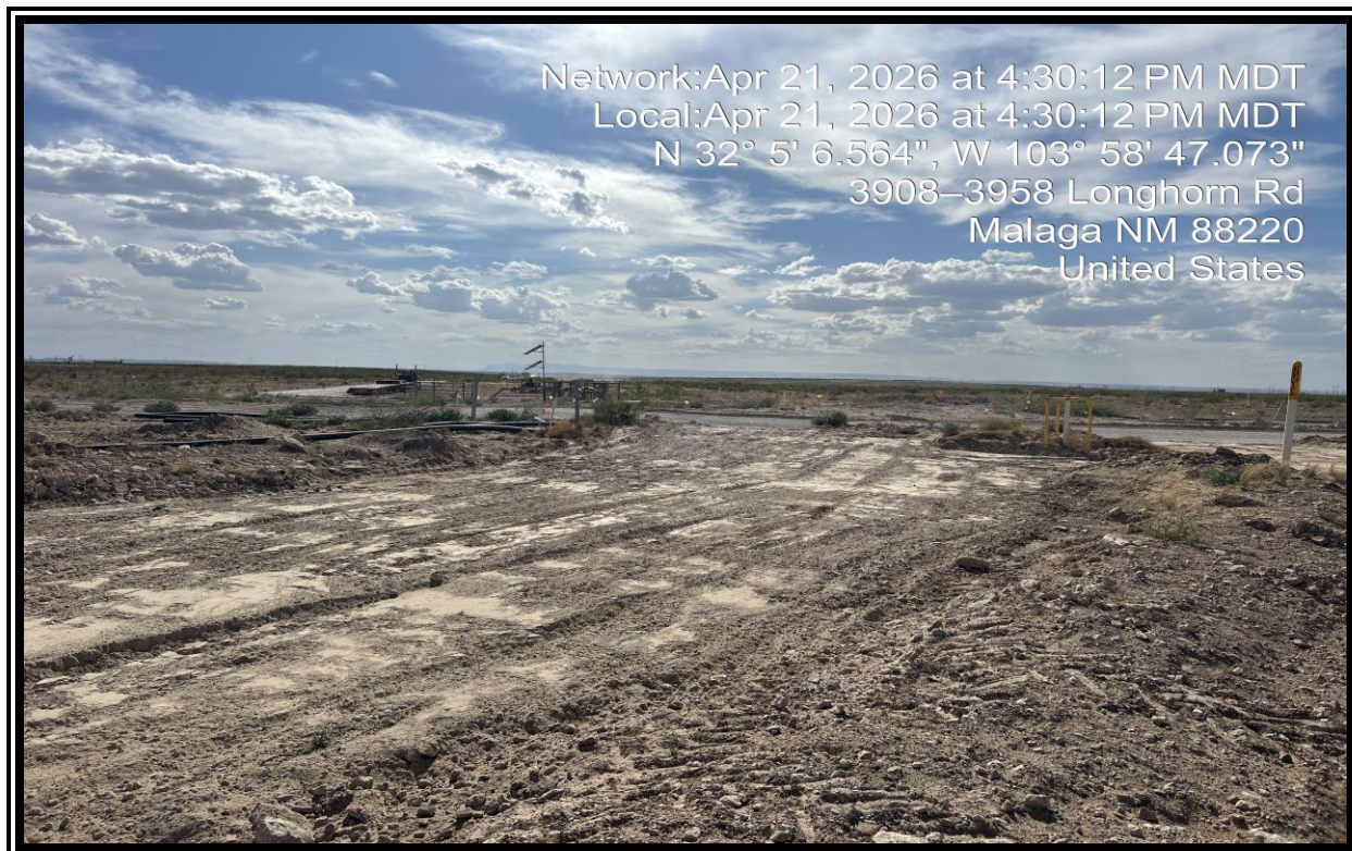
View of the site following backfill activities.
