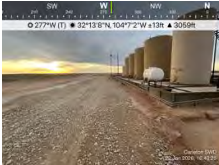
Project Site view on the backside of the SWD looking West from the East
