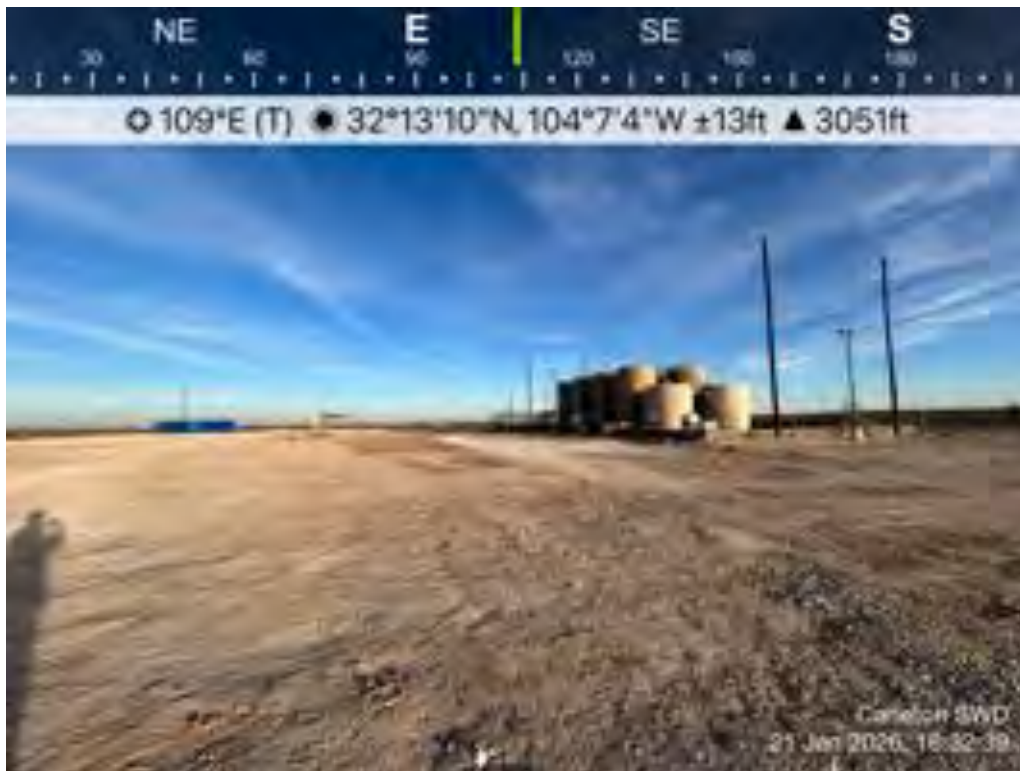
Project Site view from the Northwest looking Southeast
