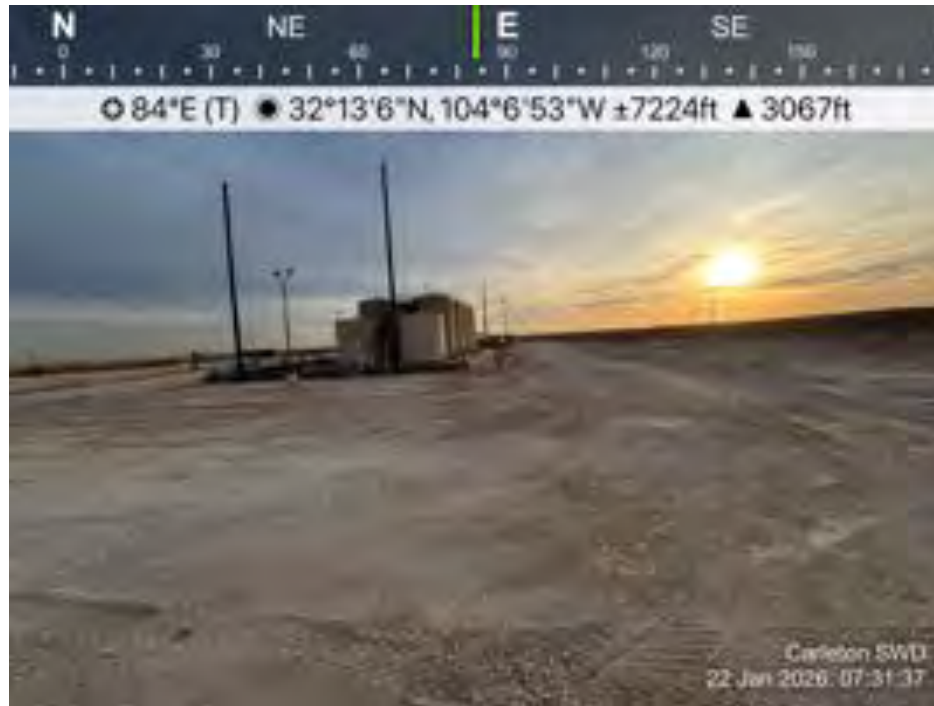
Project Site view from the West looking East
