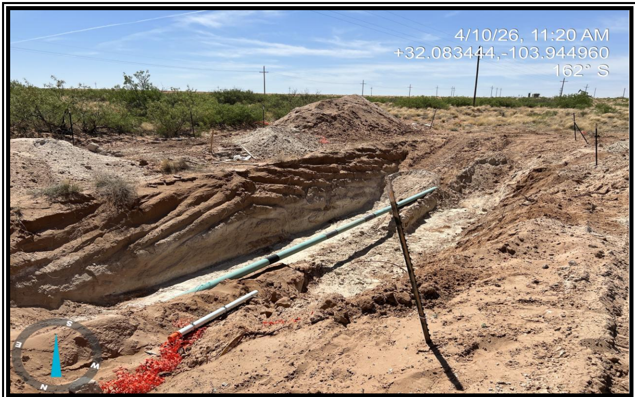
View of the site following excavation activities.
