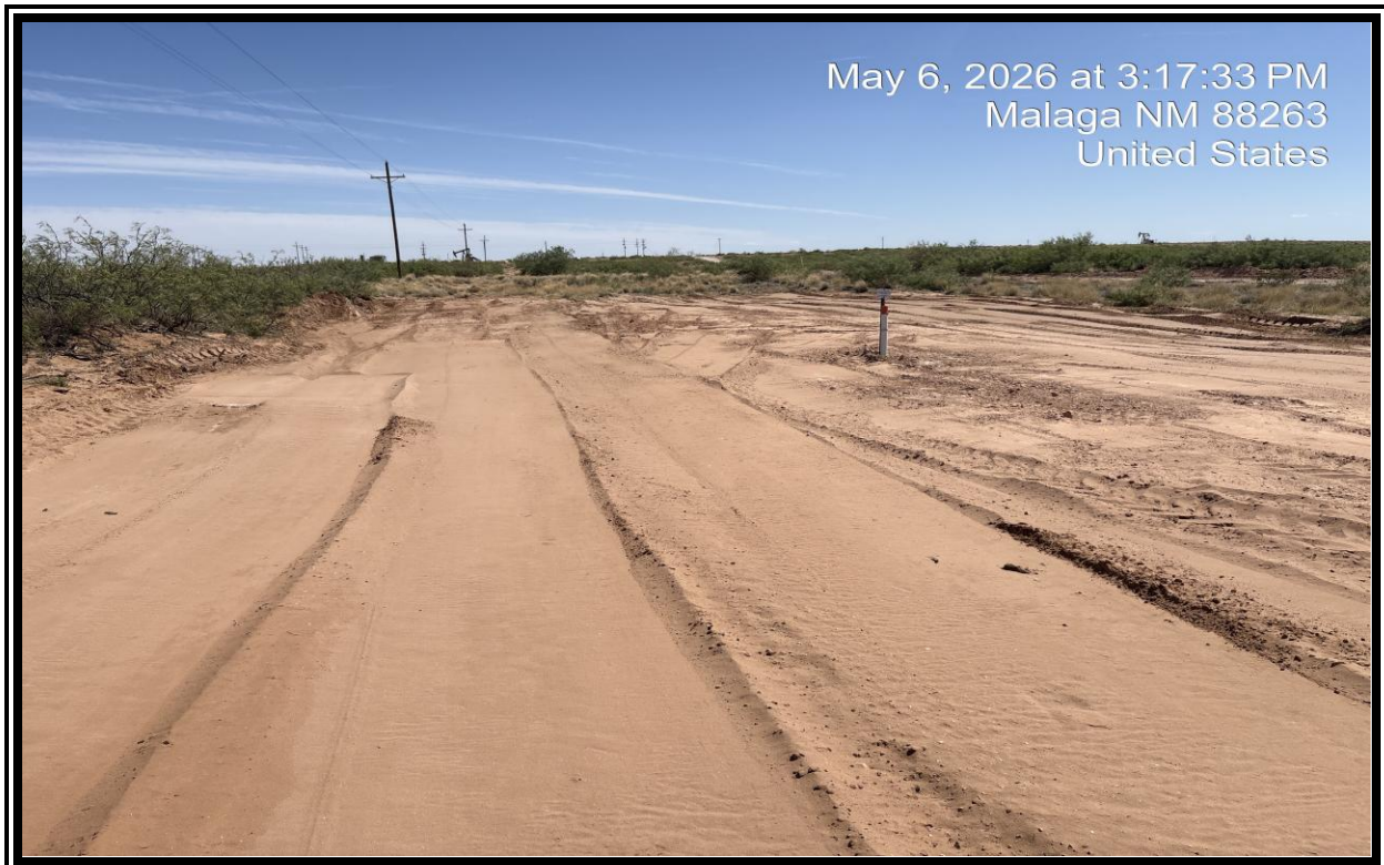
View of the site following backfill activities.
