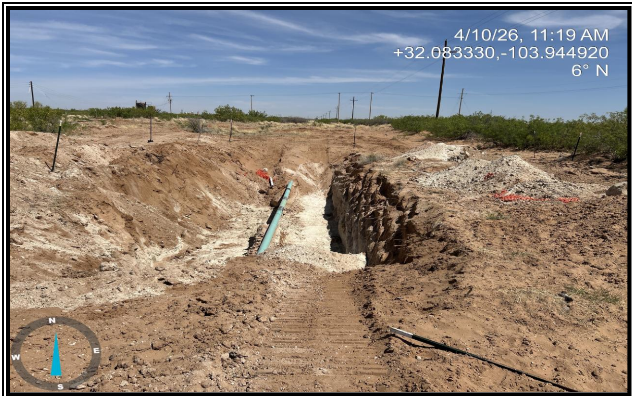
View of the site following further excavation activities.
