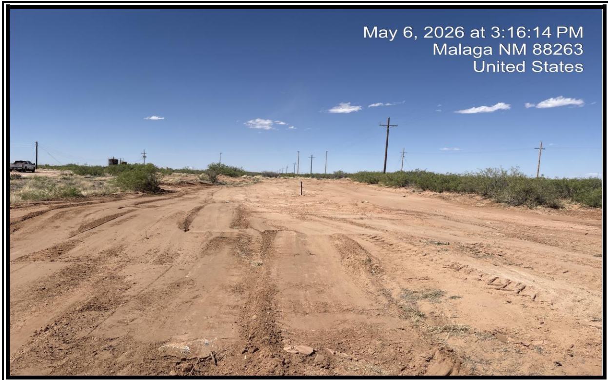
View of the site following backfill activities.
