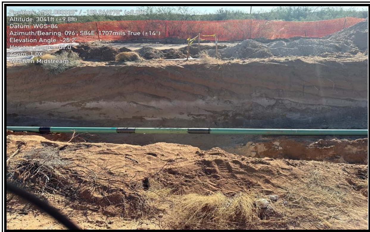
View of the site during the initial site assessment.
