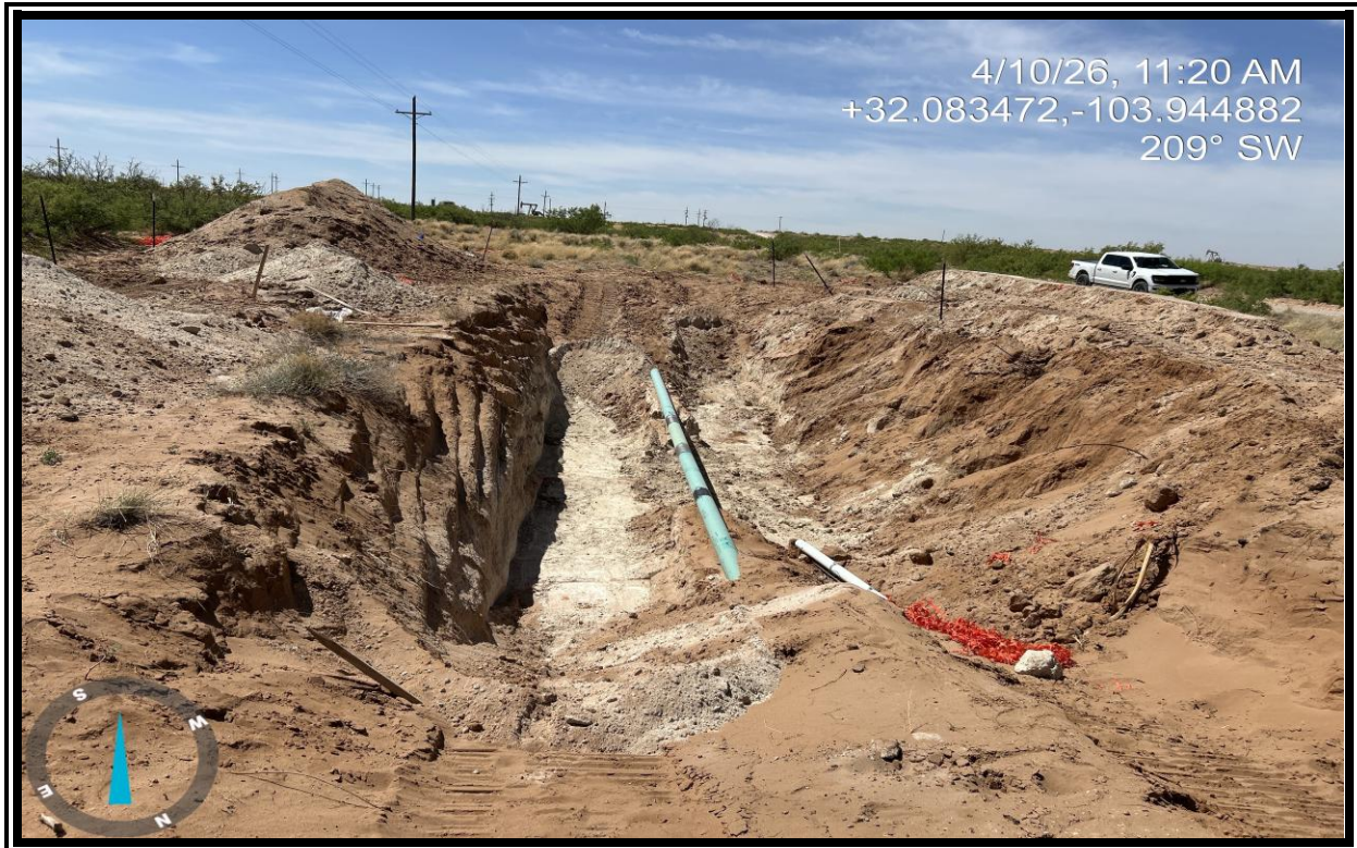
View of the site following excavation activities.
