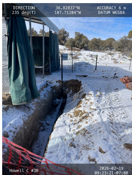
Photograph: 1 Date: 02/19/2026 Description: Excavation around leaking pipeline View: Southwest
