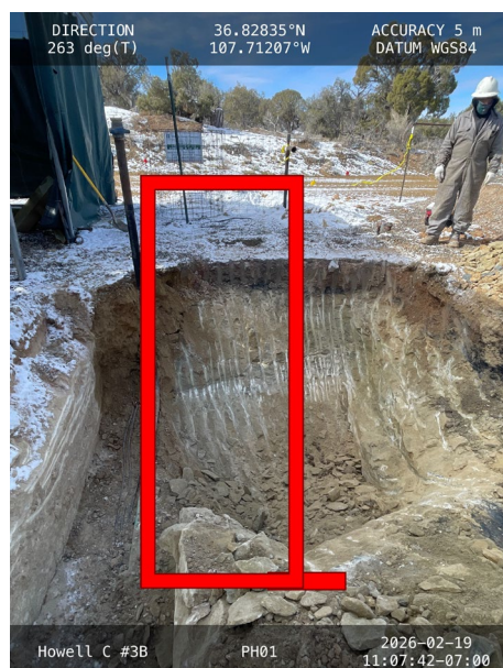
Photograph: 3 Date: 02/19/2026 Description: Location of PH01 in excavation View: West
