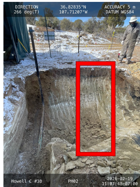
Photograph: 4 Date: 02/19/2026 Description: Location of PH02 in excavation View: West
