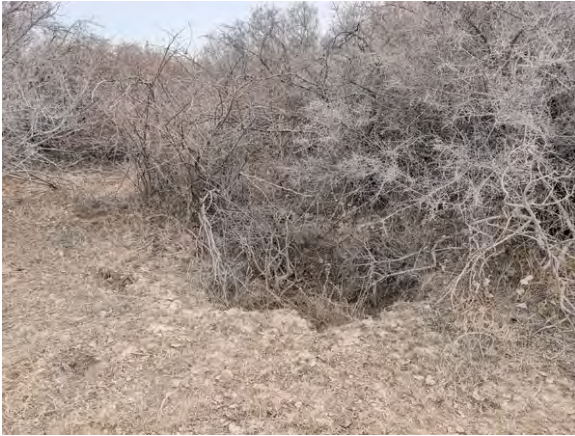
Feature KF-01, sinkhole
