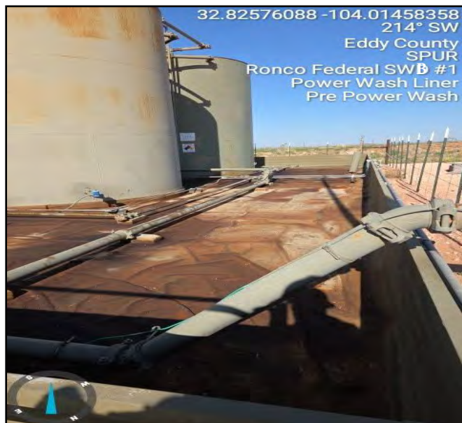
Photo taken pre powerwash process facing southwest.
