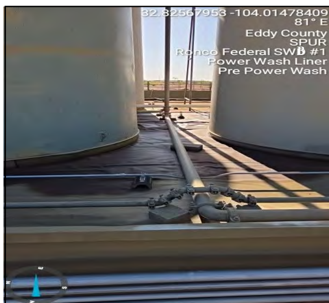
Photo taken pre powerwash process facing east.
