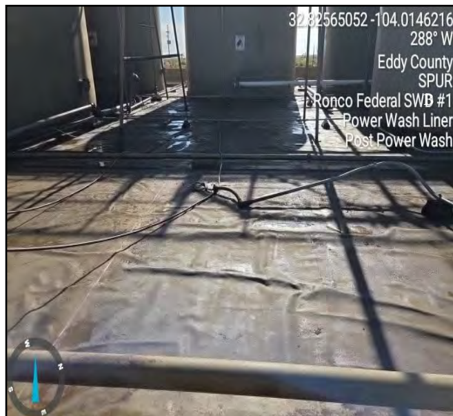
Photo taken post powerwash facing west.
