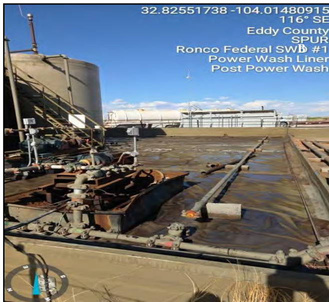
Photo taken post powerwash facing southeast.
