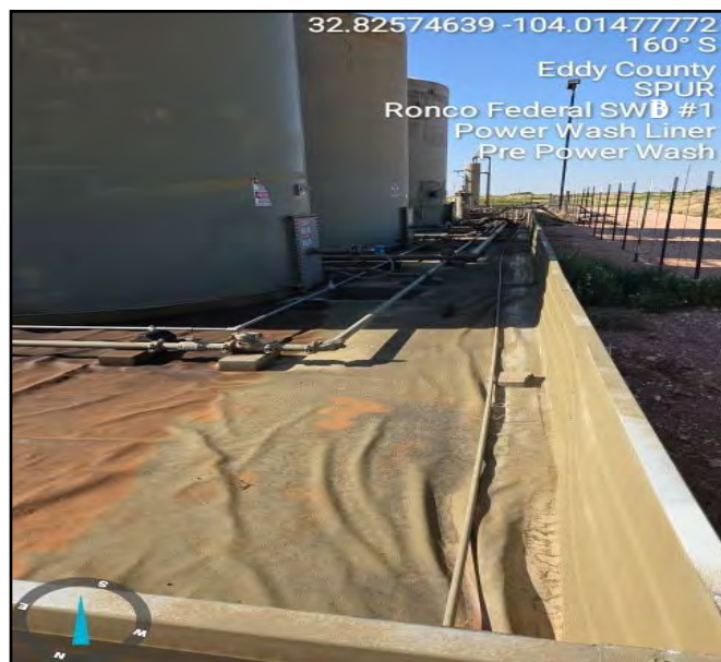
Photo taken pre powerwash process facing south.
