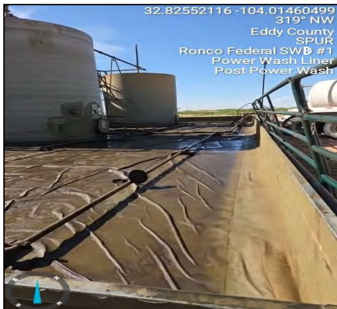
Photo taken post powerwash facing northwest.
