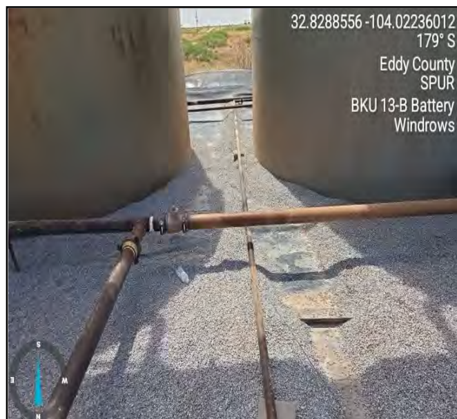
Photograph taken post windrows facing south.
