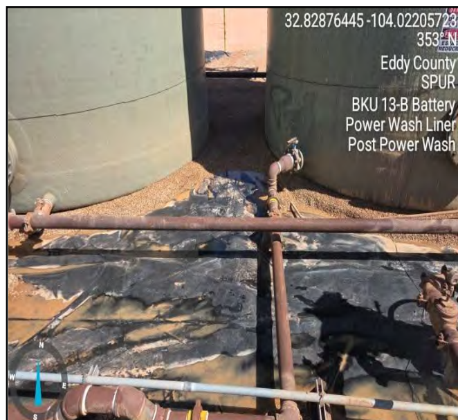
Photograph taken post powerwash process facing north.
