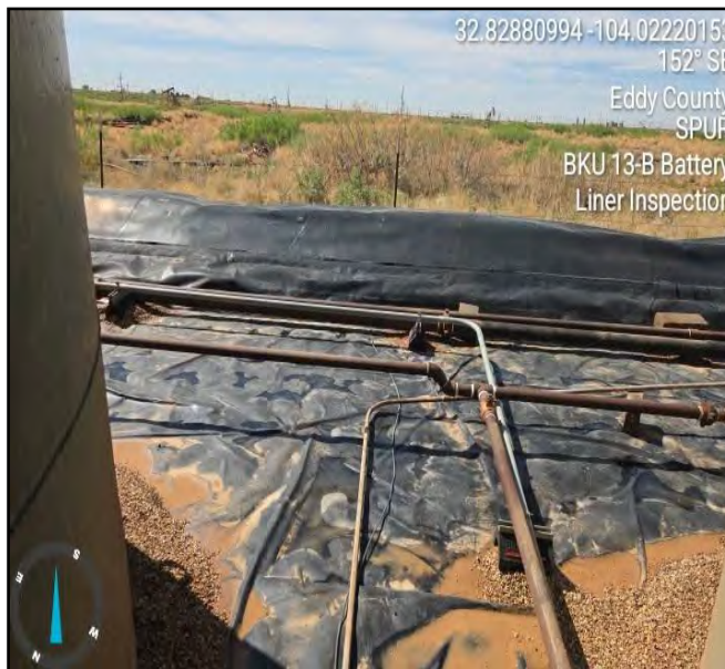
Photograph taken during liner inspection facing southeast.
