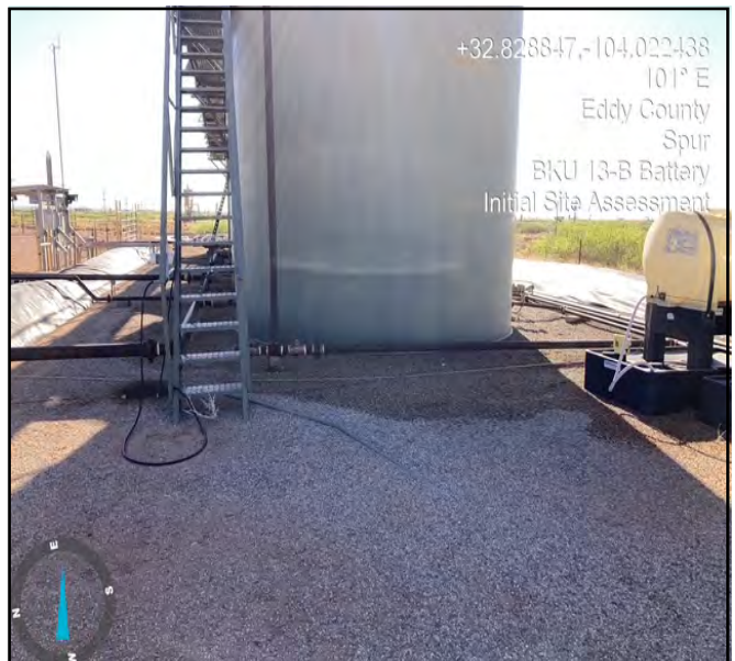
Photograph taken during initial site assessment facing east.
