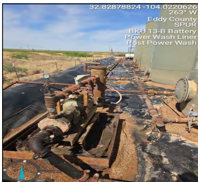
Photograph taken post powerwash process facing west.
