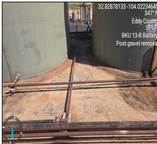
Photograph taken pre powerwash facing north.
