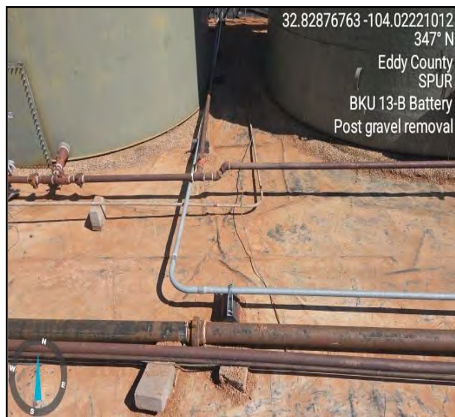
Photograph taken pre powerwash facing north.
