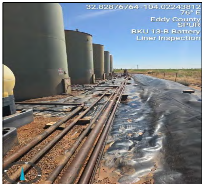
Photograph taken during liner inspection facing east.
