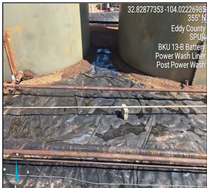
Photograph taken post powerwash process facing north.
