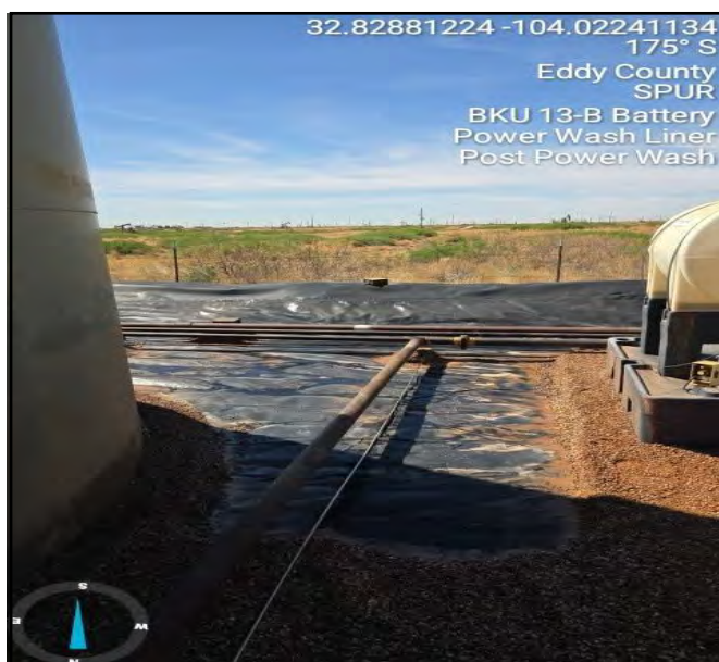
Photograph taken post powerwash process facing south.
