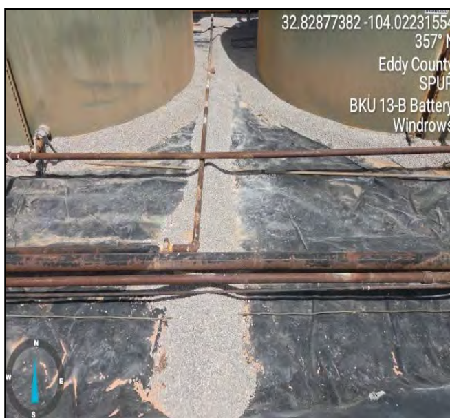
Photograph taken post windrows facing north.
