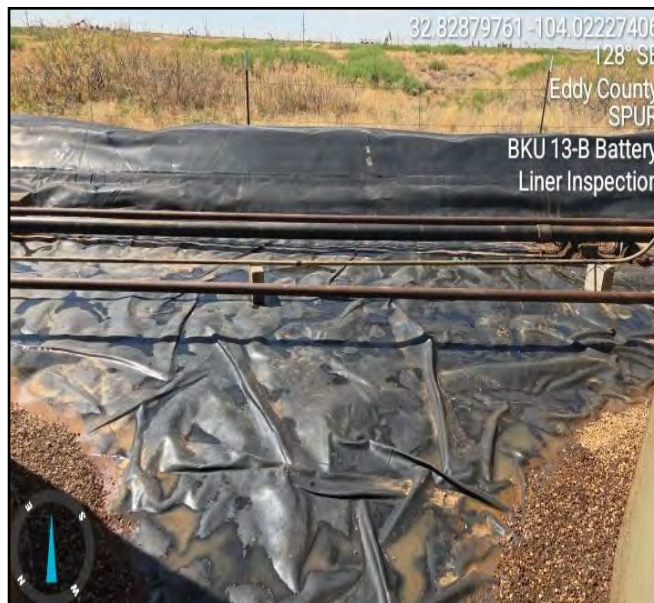
Photograph taken during liner inspection facing southeast.
