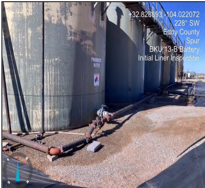
Photograph taken during initial site assessment facing southwest.
