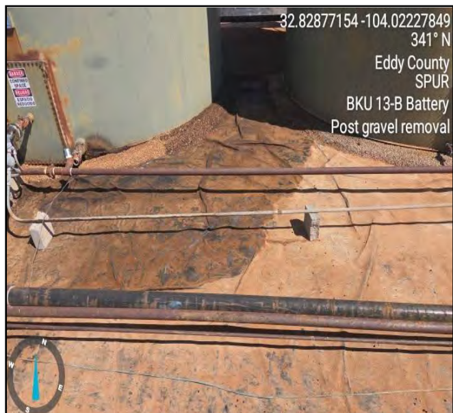
Photograph taken pre powerwash facing north.
