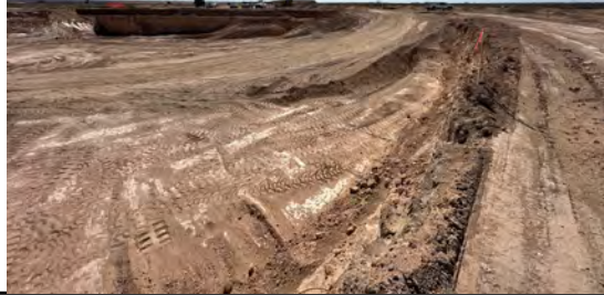
Overview of excavation
