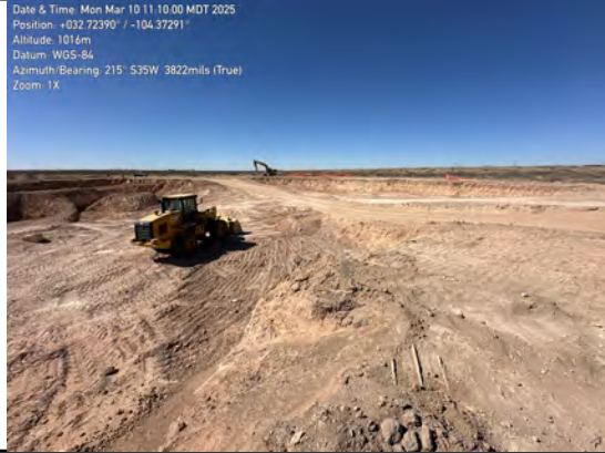
Overview of excavation
