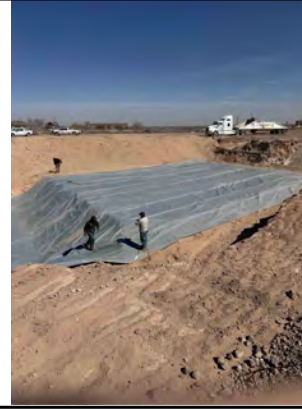
Liner Installation
