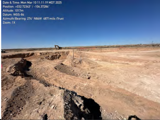
Overview of excavation
