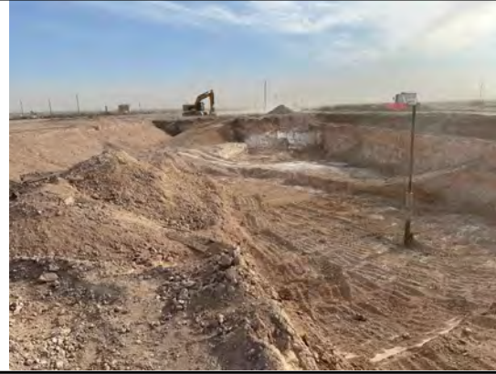
Overview of excavation
