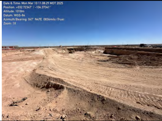
Overview of excavation
