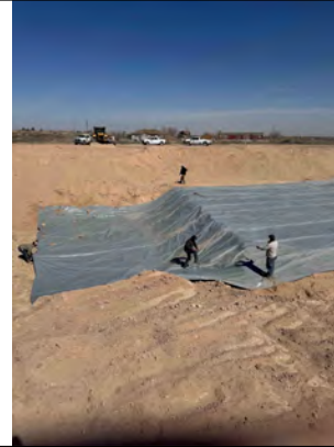
Overview of liner placement
