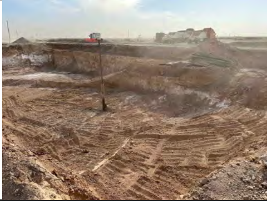
Overview of excavation
