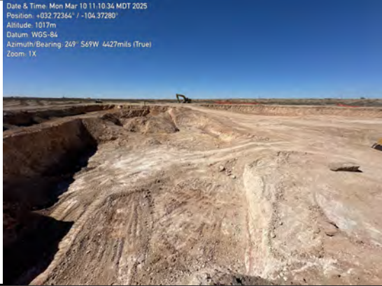
Overview of excavation
