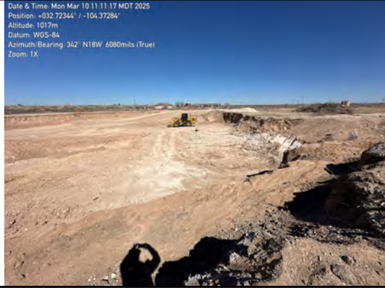
Overview of excavation
