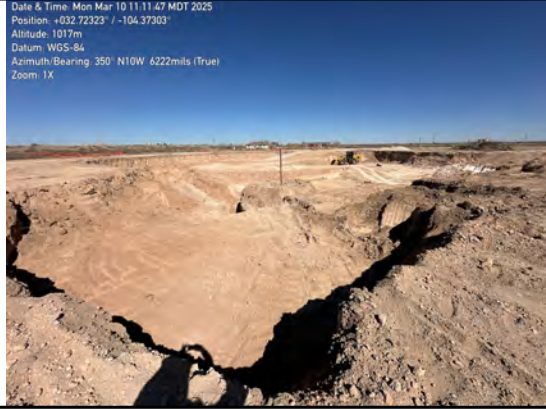
Overview of excavation
