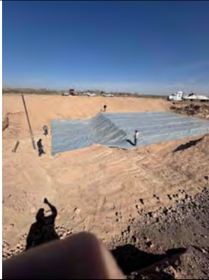
Overview of liner placement
