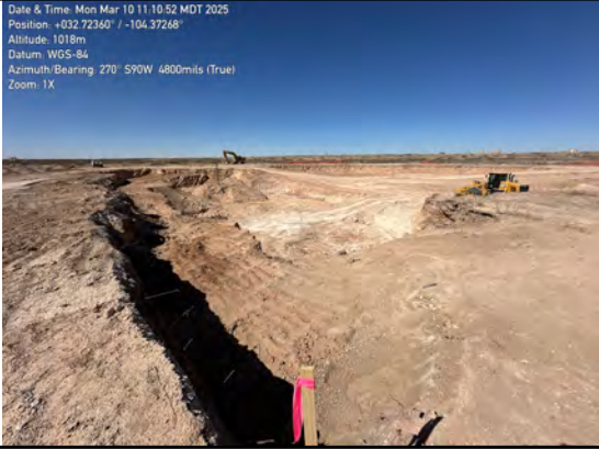
Overview of excavation
