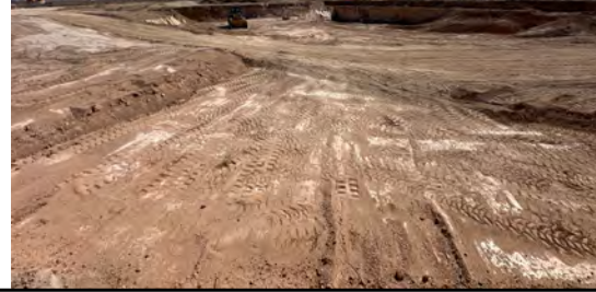
Overview of excavation
