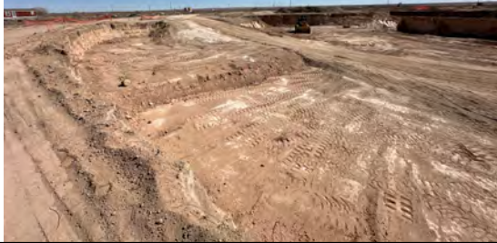
Overview of excavation
