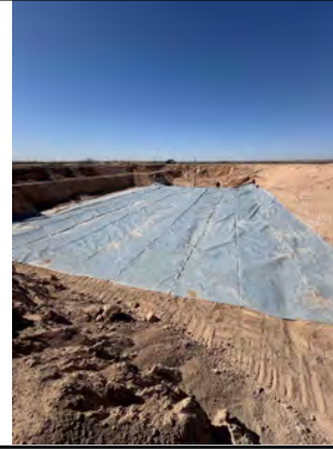
Overview of liner placement
