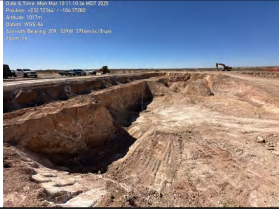
Overview of excavation
