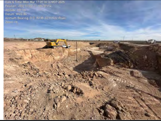
Overview of excavation
