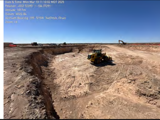
Overview of excavation
