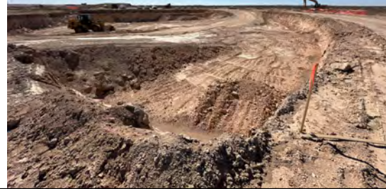
Overview of excavation
