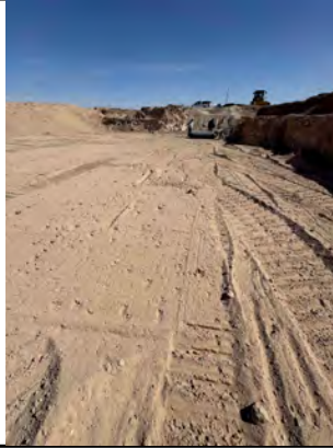
Areas backfilled to 10ft BGS before liner placement
