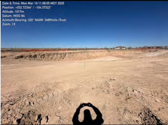
Overview of excavation
