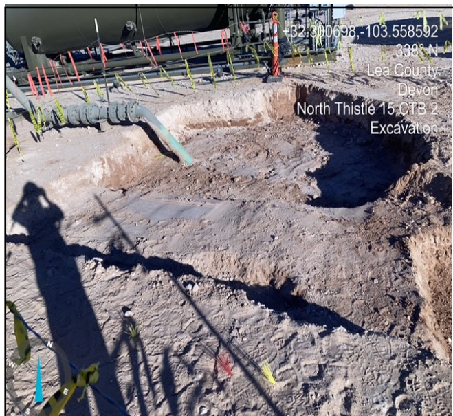
Excavation facing northwest.
