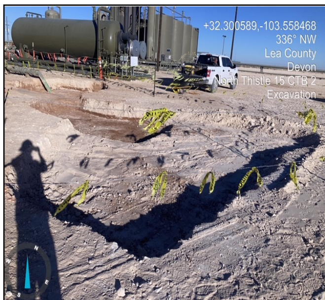
Excavation facing northwest.
