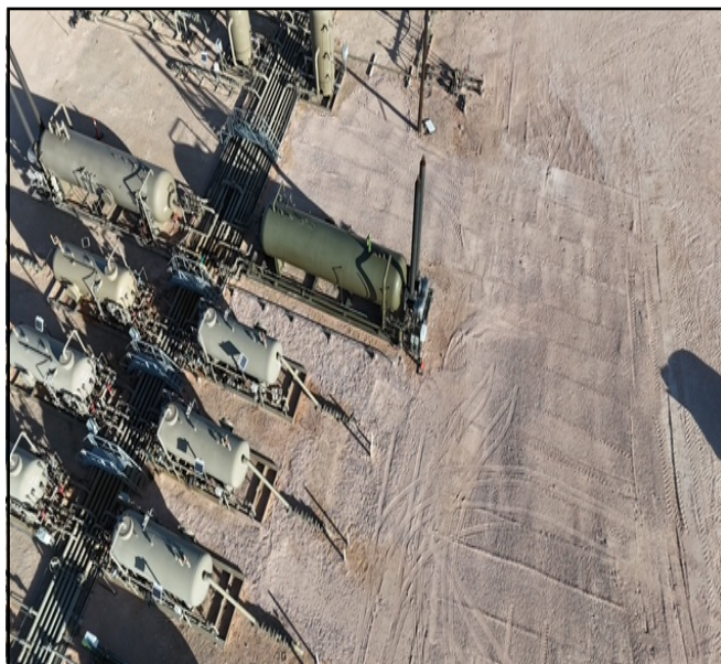
Post excavation aerial view.
