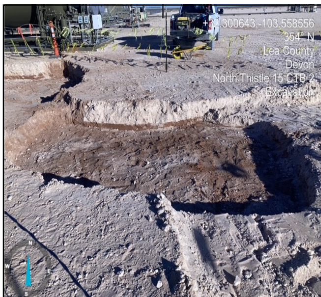
Excavation facing north.
