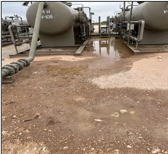
Photograph taken during assessment facing west.
