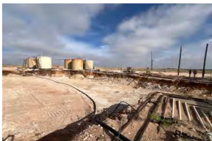
View to NW of excavation (4/22/26).
