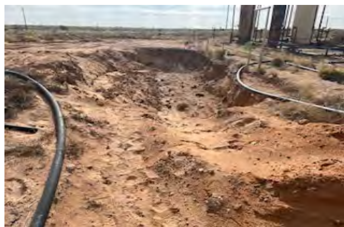
View to E of excavation N of TB (4/22/26).
