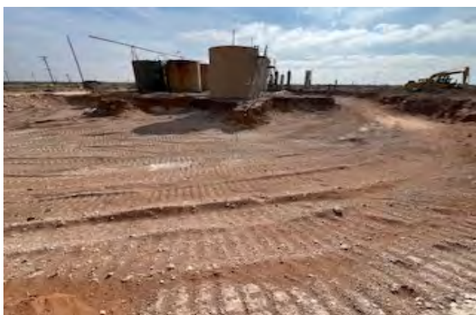
View to E of excavation W of tanks (4/22/26).
