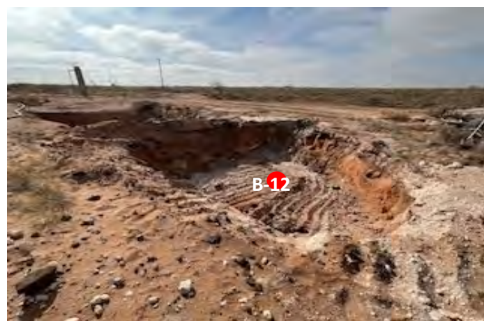
View to E of excavation S of TB (4/22/26).
