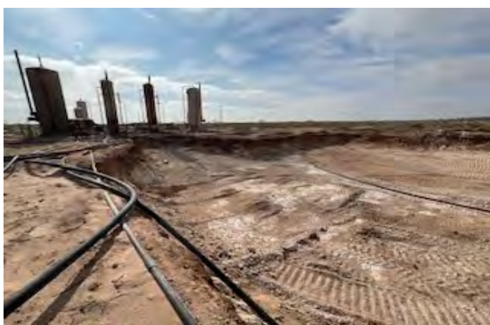
View to E of excavation (4/22/26).
