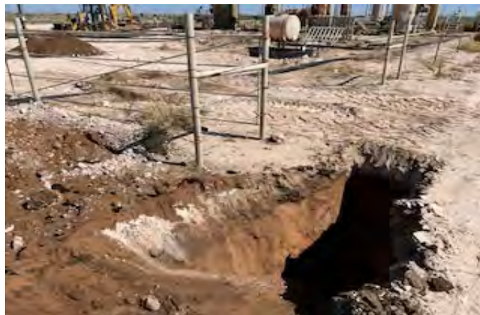
View to NE of test hole TH-17 (10/16/25).
