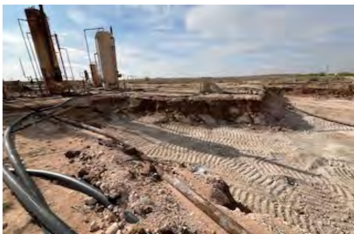
View to SE of excavation (4/22/26).
