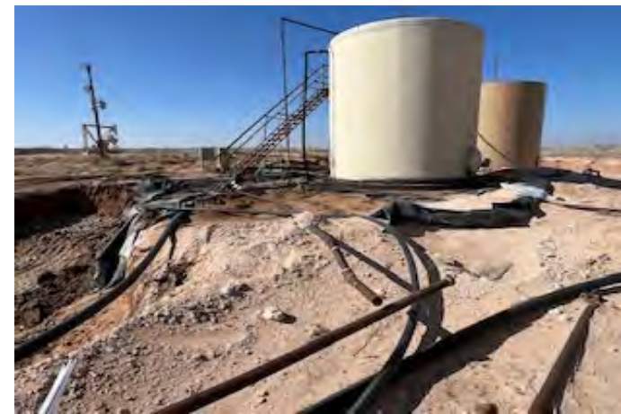
View to SW of excavation around tanks (3/2/26).
