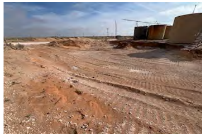
View to NE of excavation W of tanks (4/22/26).
