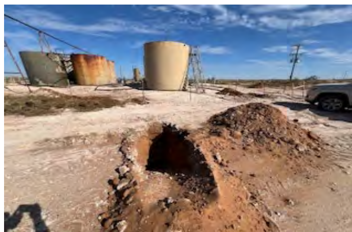
View to E of test hole TH-32 (10/16/25).
