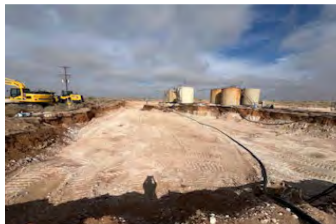
View to W of excavation (4/22/26).
