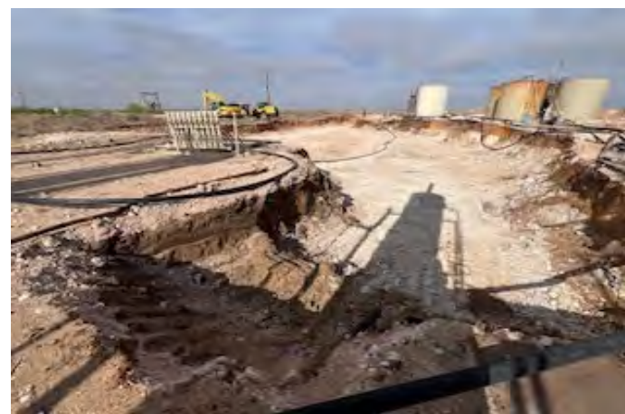
View to W of excavation (4/22/26).
