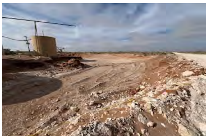
View to E of excavation S of tanks (4/22/26).
