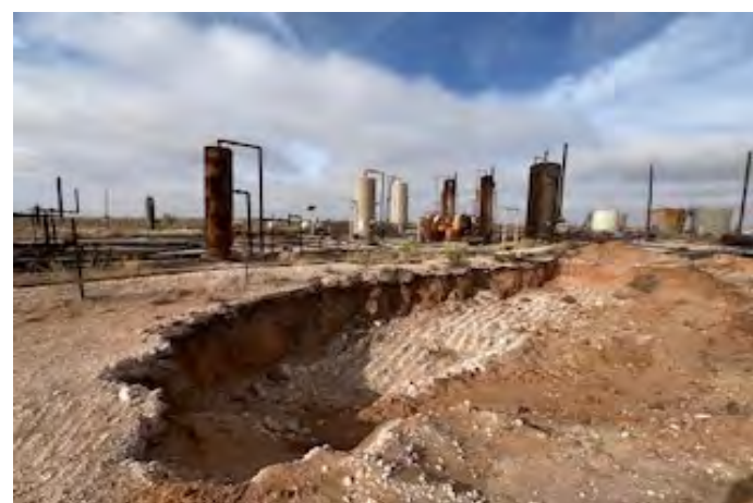
View to W of excavation N of TB (4/22/26).
