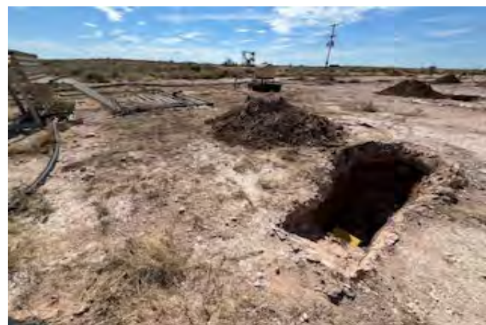
View to SW of test hole TH-22 (10/16/25).
