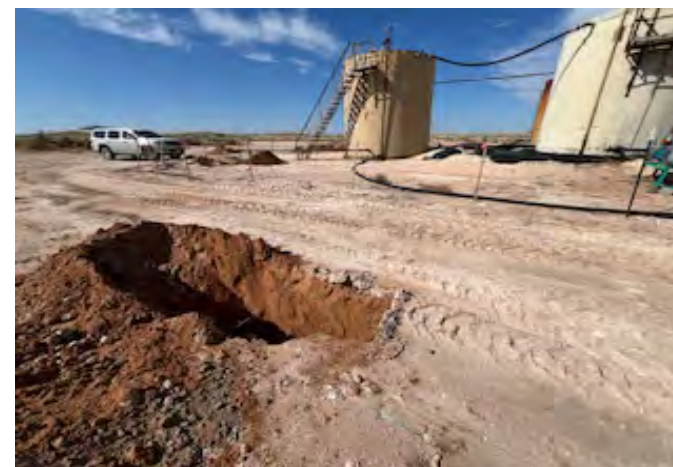
View to NW of test hole TH-28 (10/16/25).
