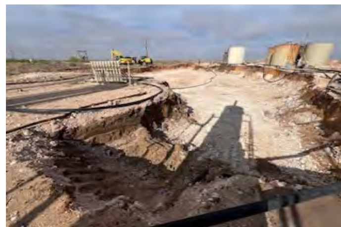
View to W of excavation (4/22/26).
