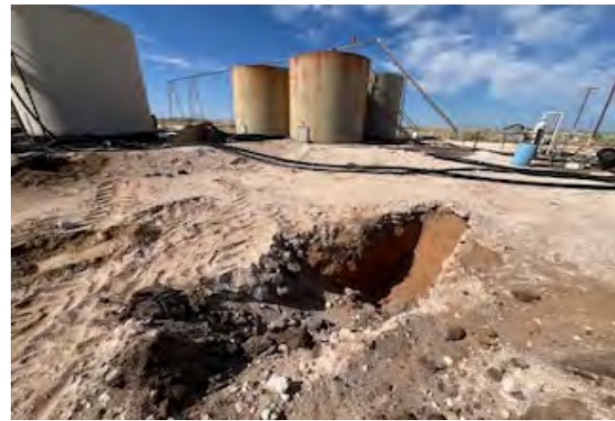
View to NW of test hole TH-26 (10/16/25).
