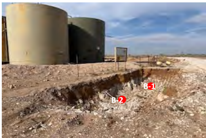
View to W of excavation N of tanks (4/22/26).
