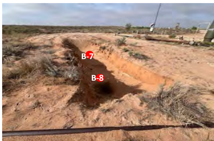
View to S of excavation at TH-15/B-7 (4/22/26).
