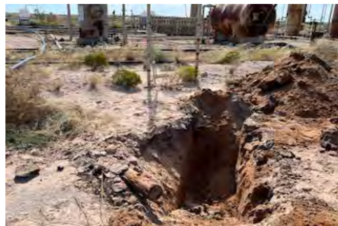
View to S of test hole TH-20 (10/16/25).
