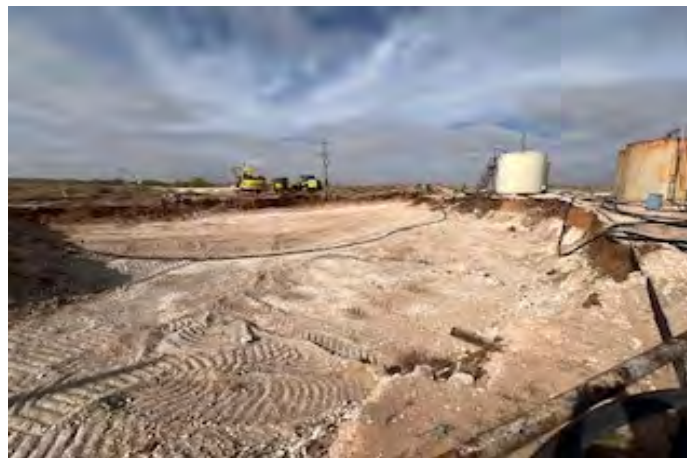
View to W of excavation (4/22/26).
