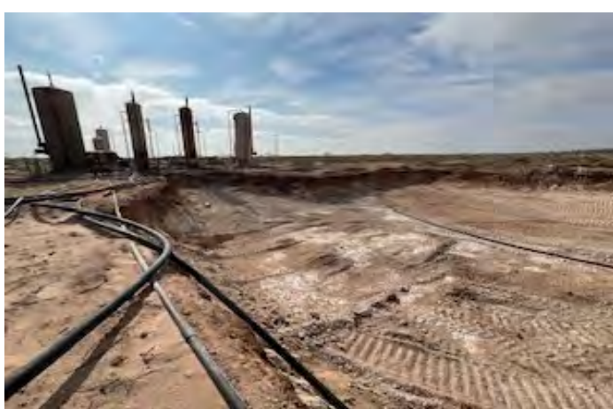
View to E of excavation (4/22/26).
