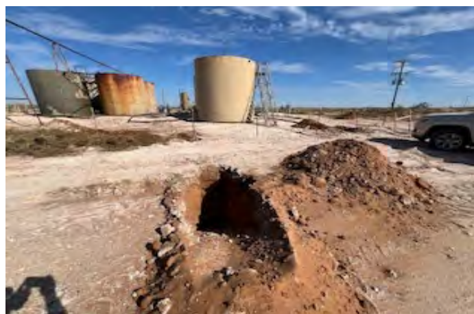
View to E of test hole TH-32 (10/16/25).
