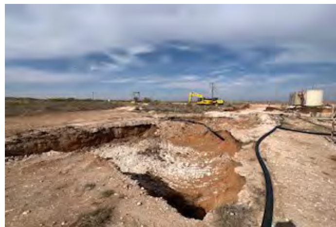
View to W of excavation S of TB (4/22/26).
