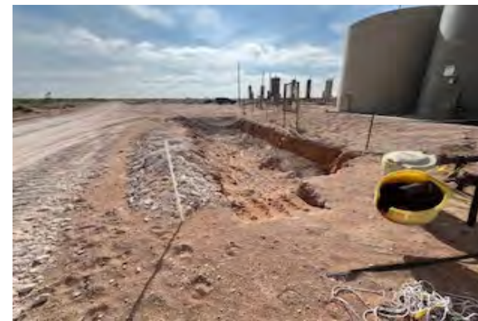
View to E of excavation N of tanks (4/22/26).
