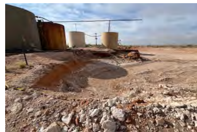
View to S of excavation W of storage tanks (4/22/26).
