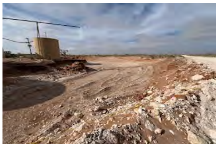
View to S of excavation W of tanks (4/22/26).
