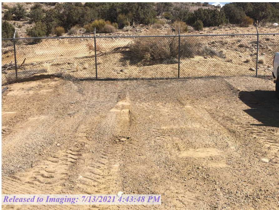
Backfilled area of former Tank A
