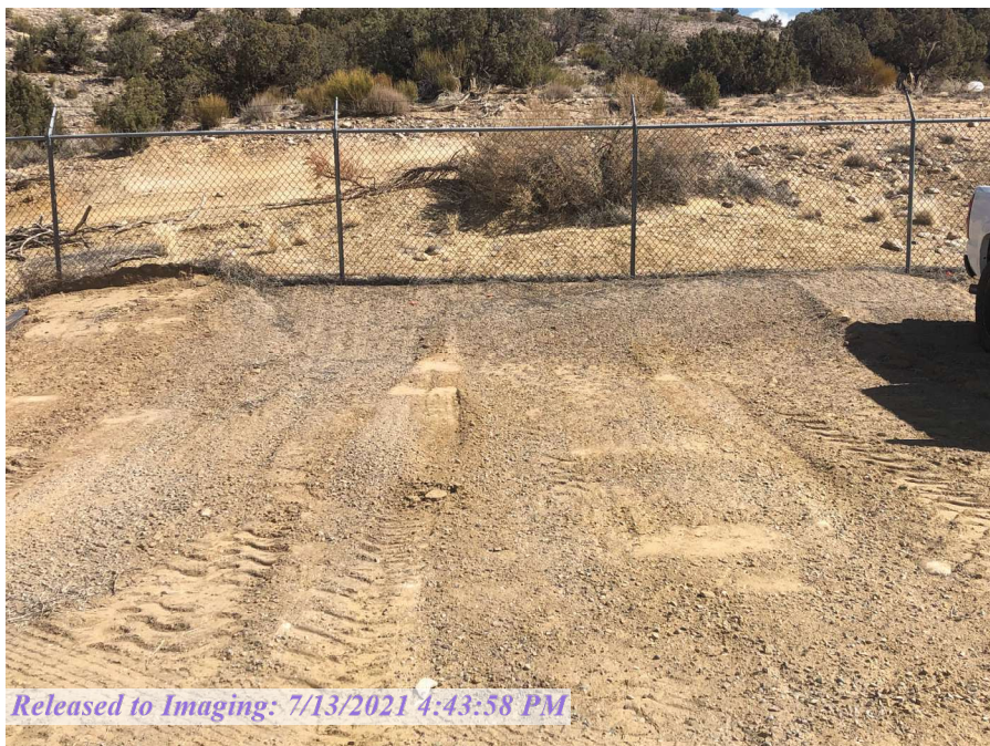
Backfilled area of former Tank A
