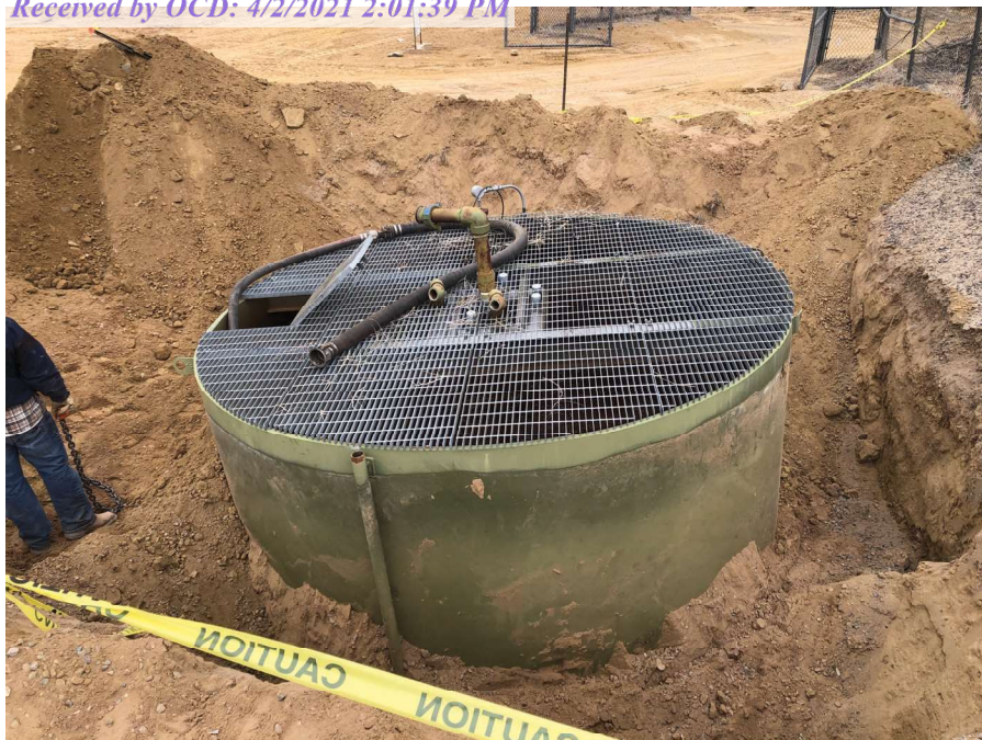
GCU 133E - BGT Tank A prior to removal
