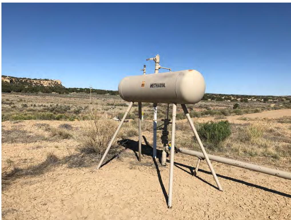
Figure 12. Methanol drip equipment to be removed.
