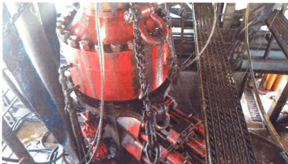
Figure 1: Winch System attached to BOP Stack
