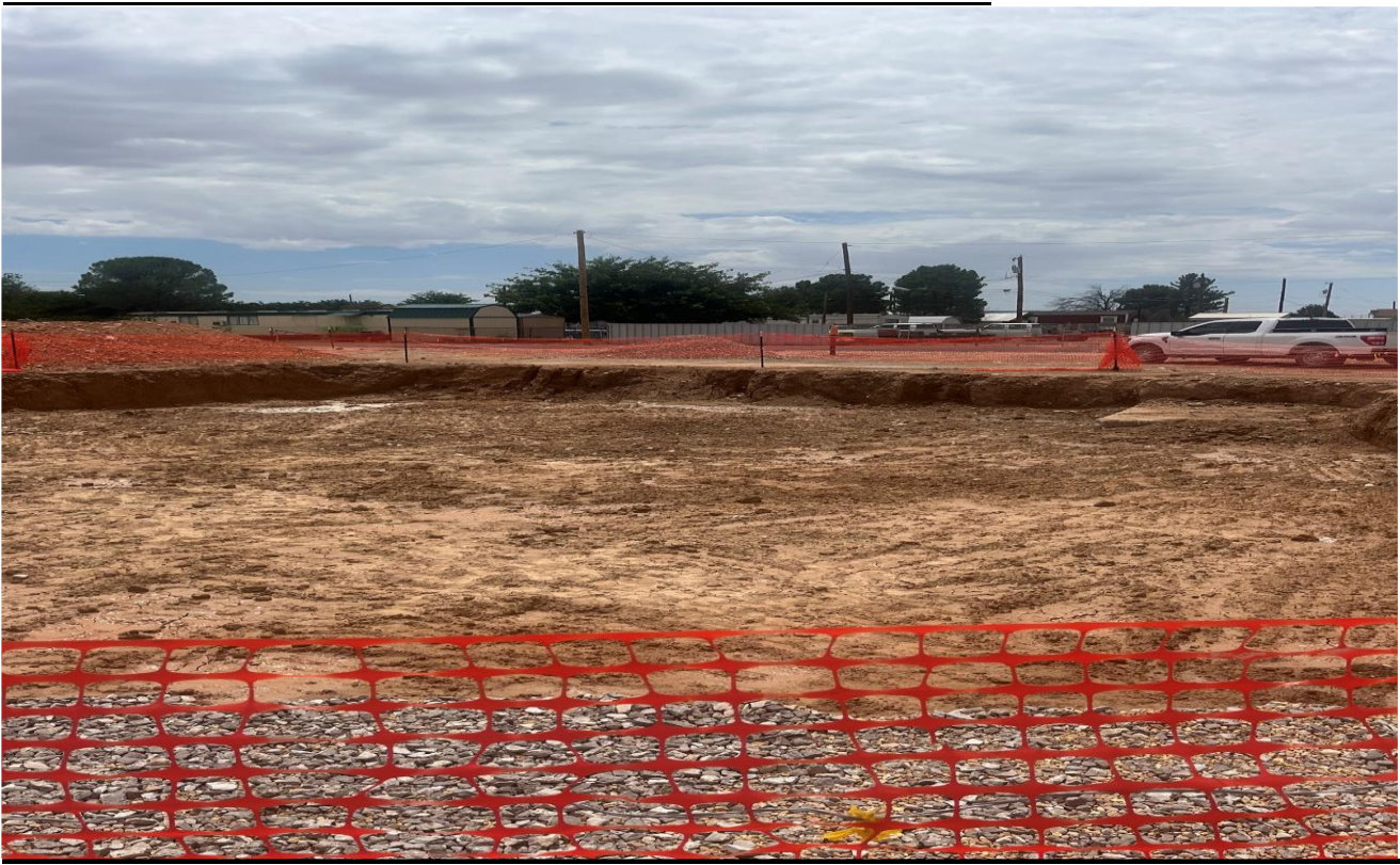
Figure 3 View of excavation looking south.
