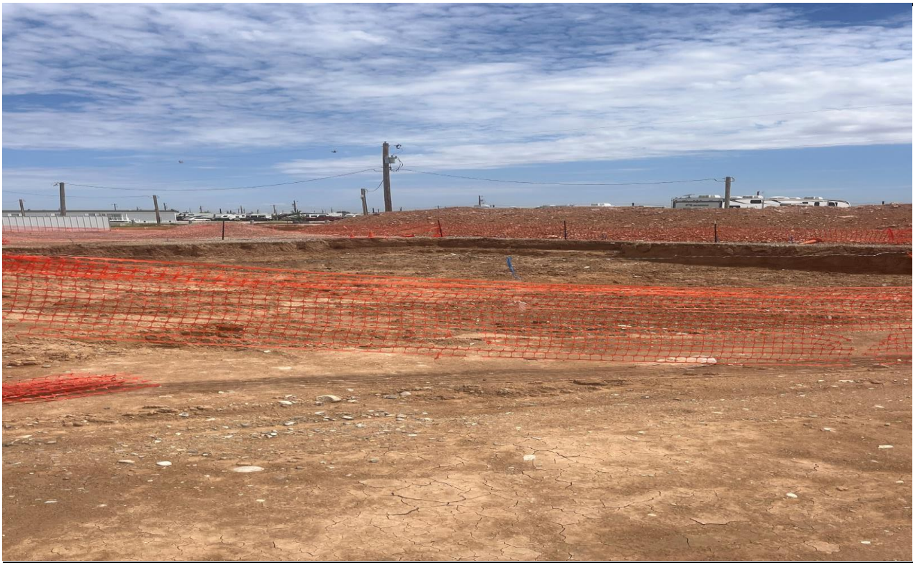
Figure 2 View of excavation looking north west.
