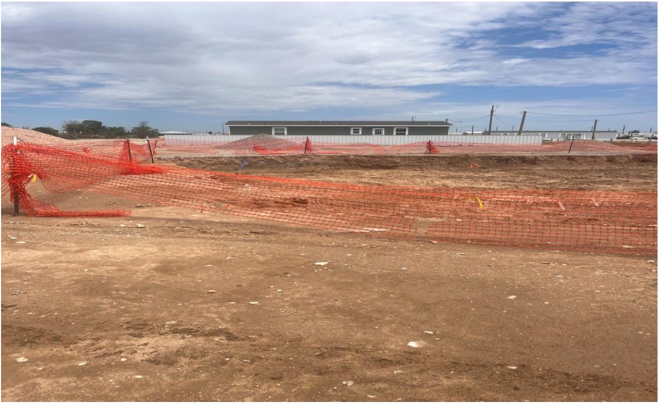
Figure 1 View of excation looking north.
