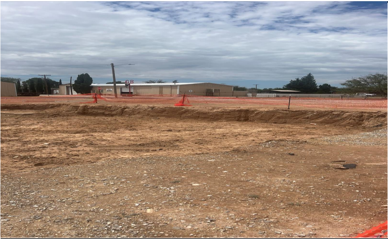
Figure 4 View of excavation looking Southwest.
