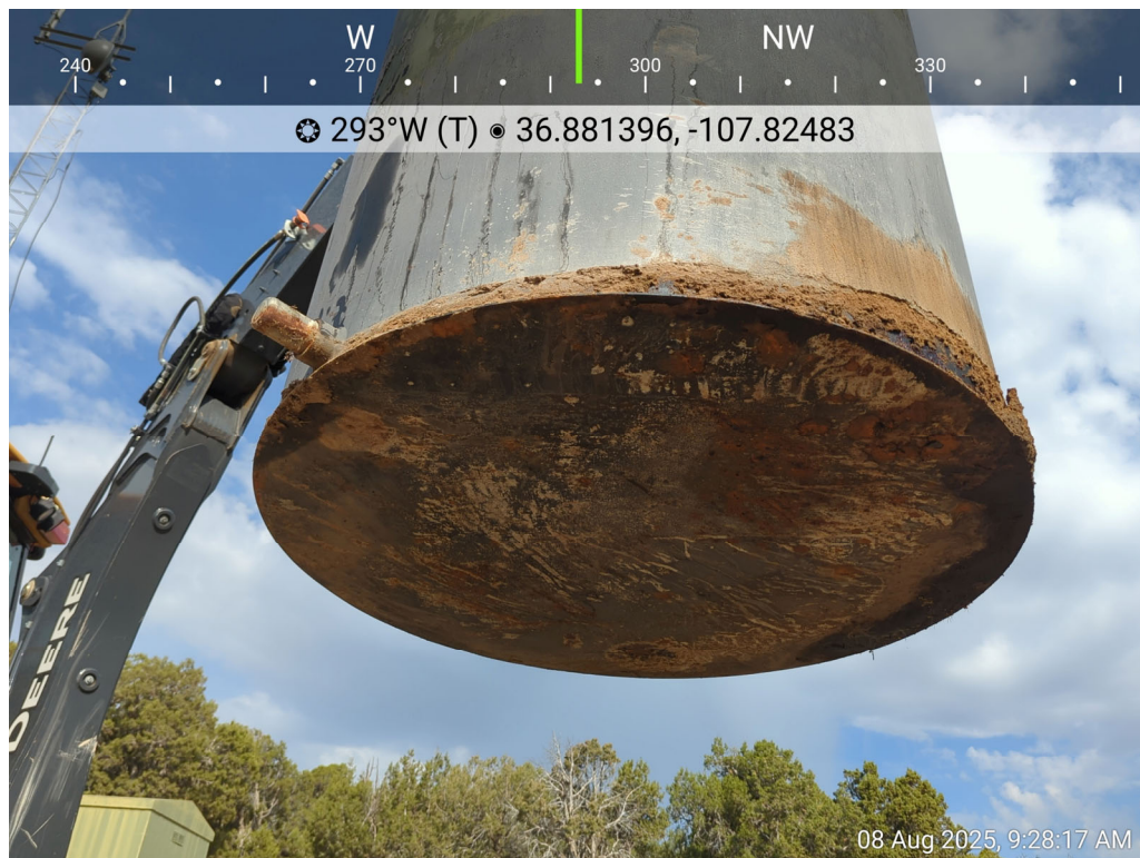
Photo 4: Bottom of BGT following removal.
