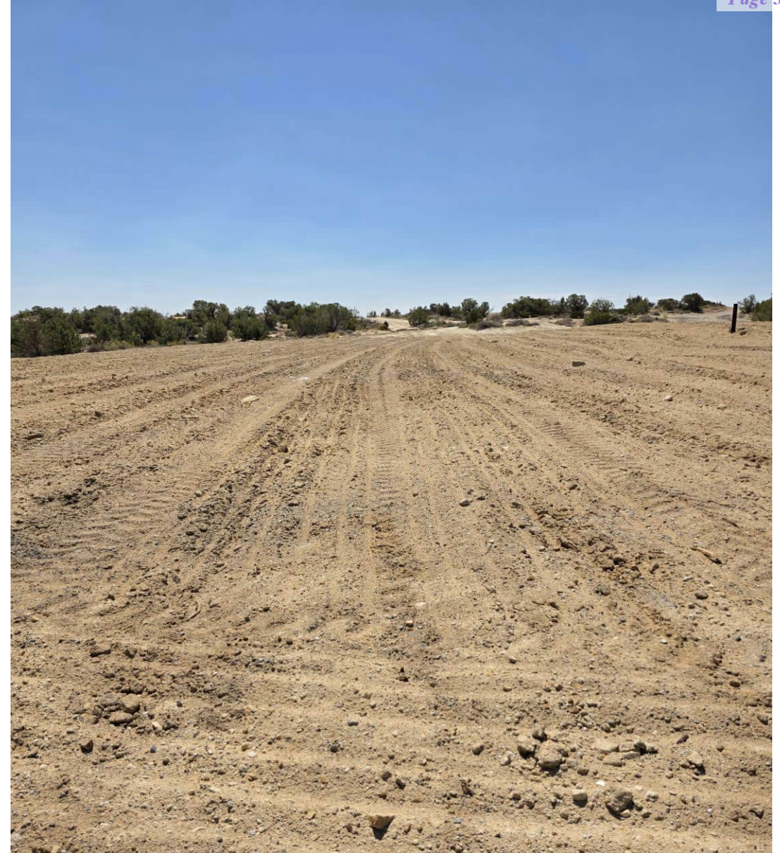
View Looking South
